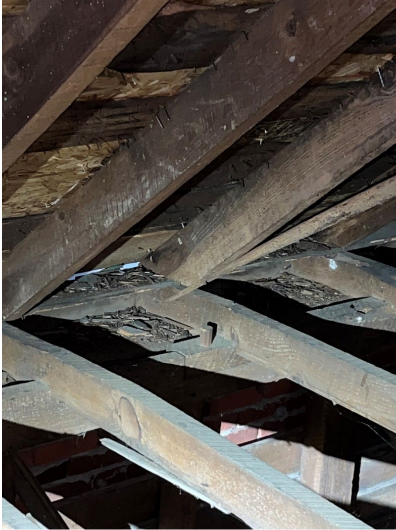
Pegged plate (above; Figure 12) and detail of peg (below; Figure 13).
