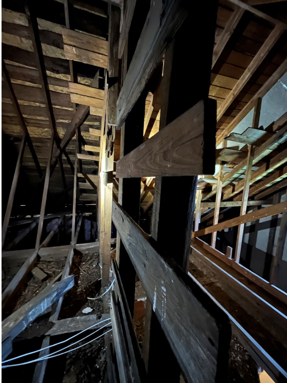
Ladder leading to bell tower (removed) (Figure 18).
