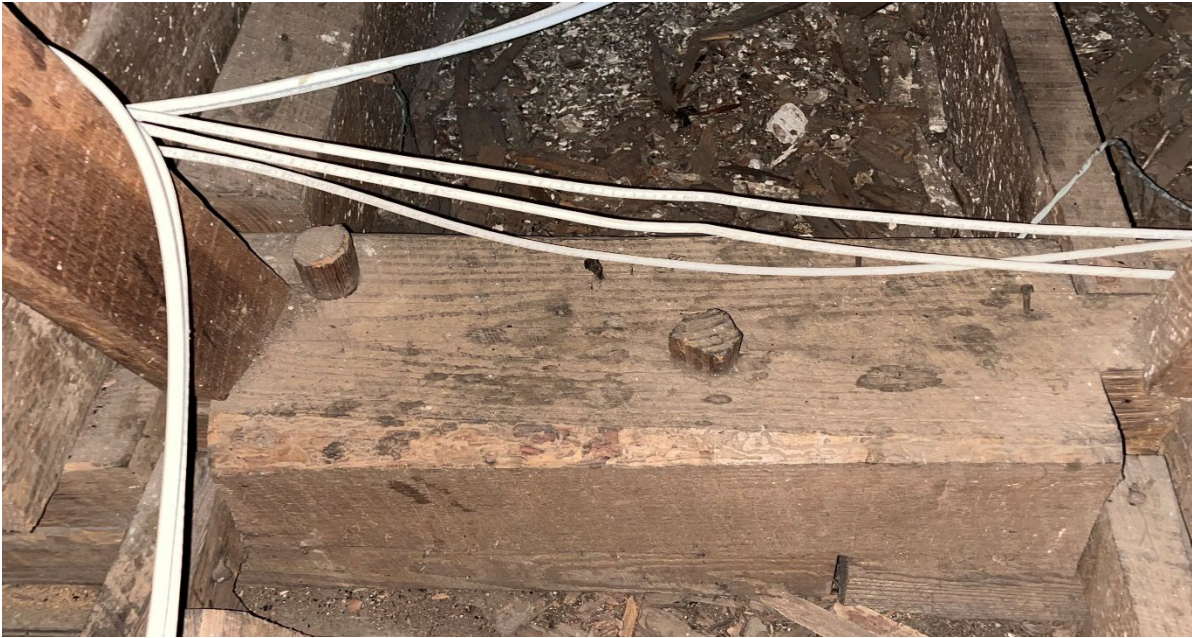
Pegged construction (above; Figure 14) and hand forged nails (below; Figure 15).
