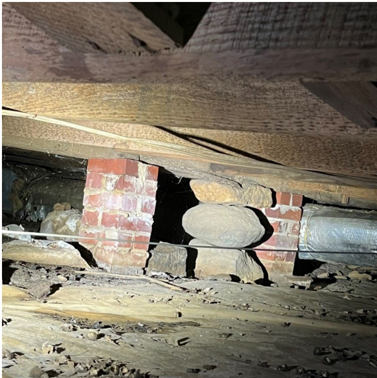
Foundation pier and subfloor (above; Figure 9); foundation stones and newer piers (below; Figure 10).
