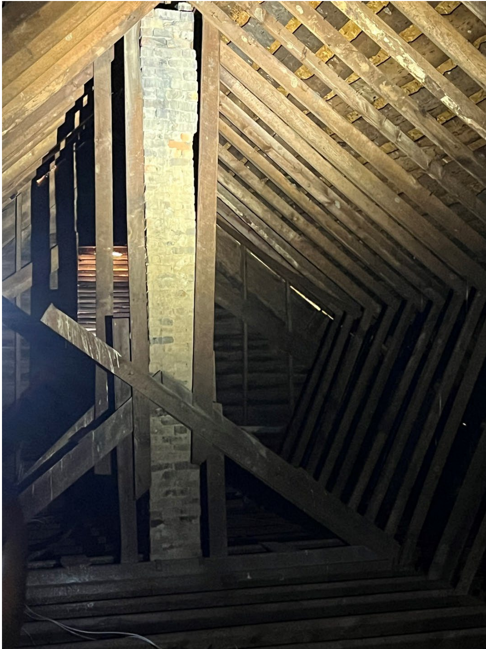
Attic chimney and framing (Figure 11).
