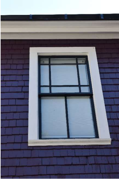
Typical upstairs window, nine-over-two configuration
