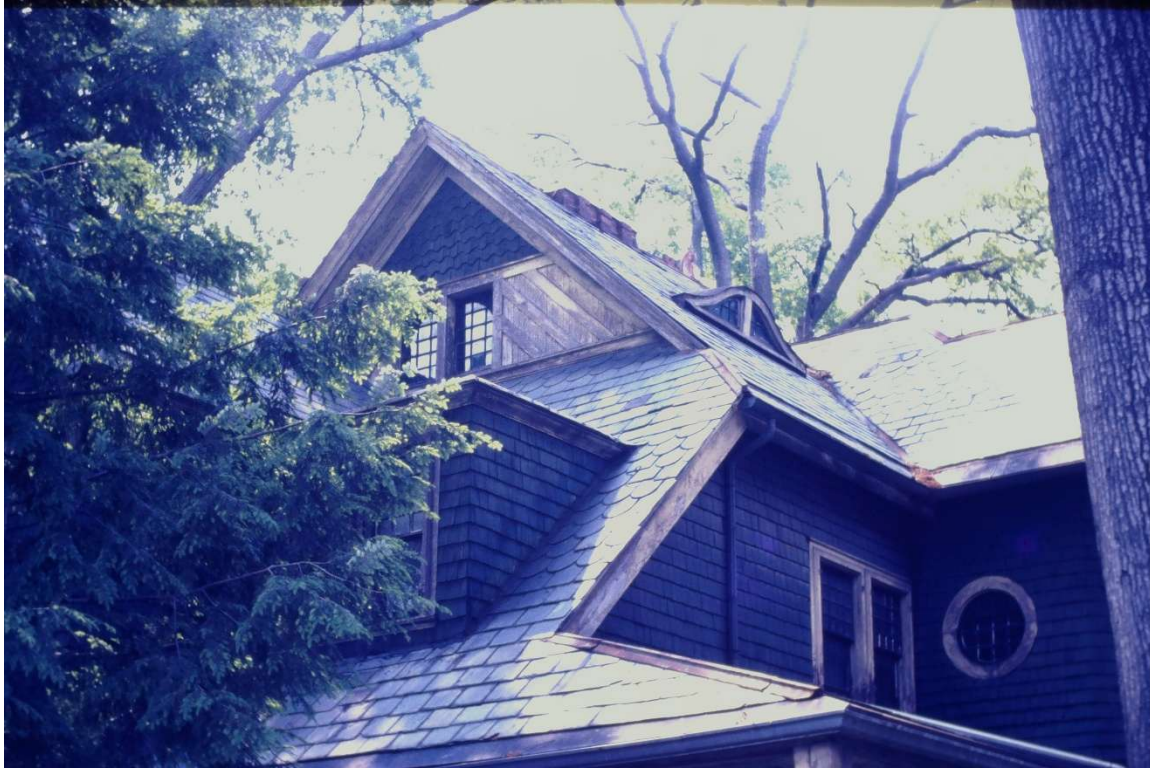
Façade/East Elevation, ca. 1975
