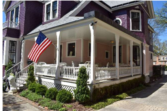
Front porch looking southwest
