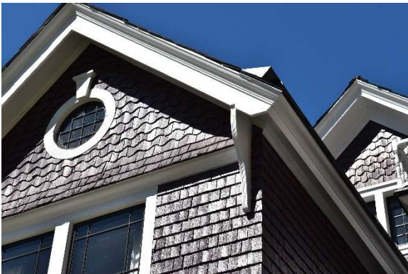
Gable and eave detail of two-story façade bay
