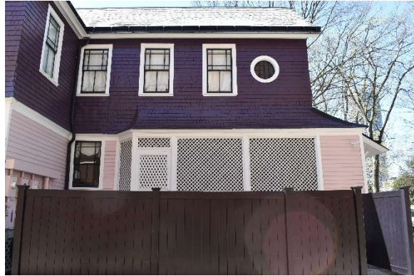
Rear section looking south
