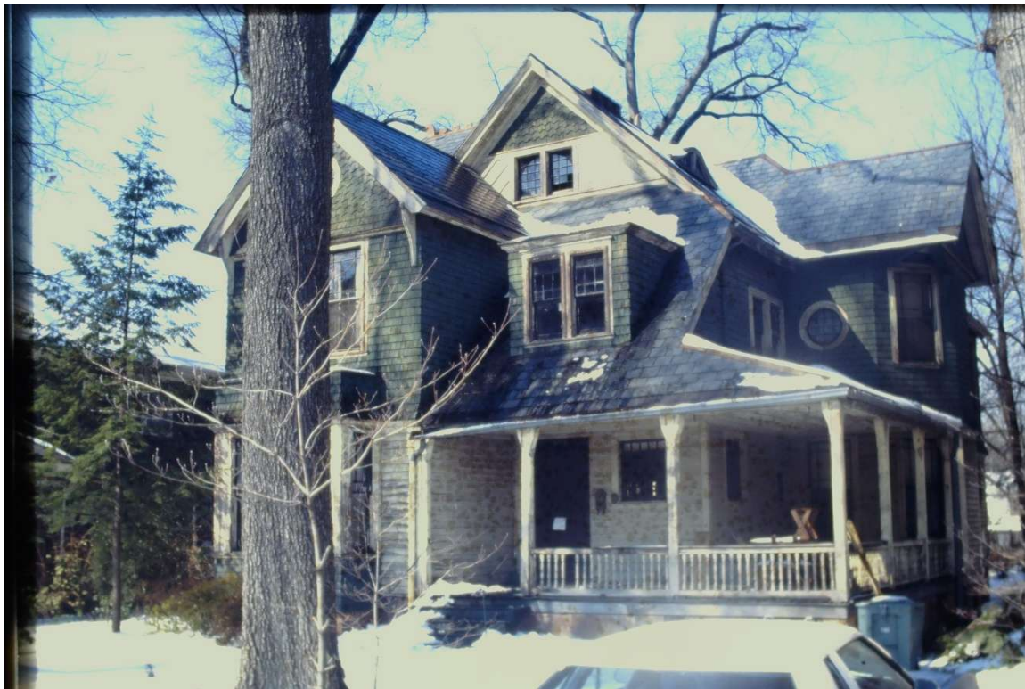
Façade/East Elevation under renovation, ca. 1980
