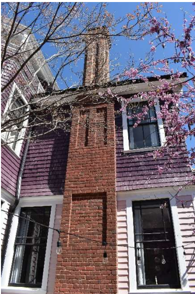
Front chimney looking north
