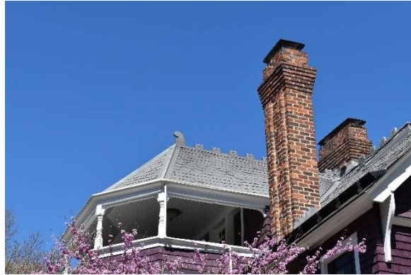
View of attic porch looking west also showing roof rake details, front chimney of south elevation, and interior chimney
