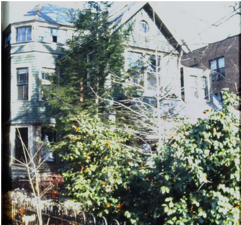
Façade/East Elevation, ca. 1975
