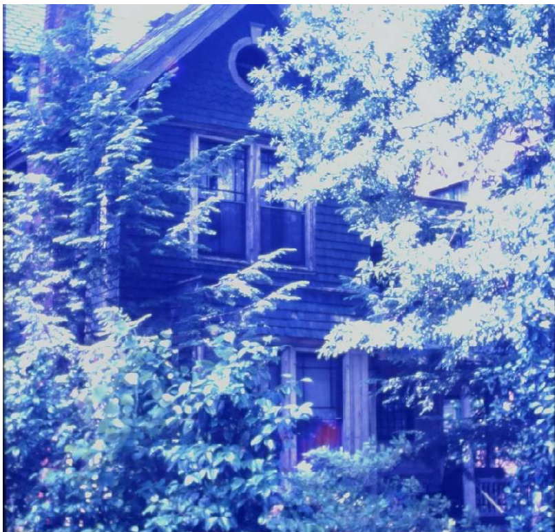
Façade/East Elevation, ca. 1975
