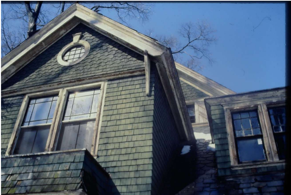
Façade/East Elevation, ca. 1980
