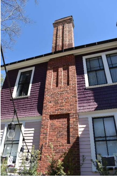
Rear chimney looking north
