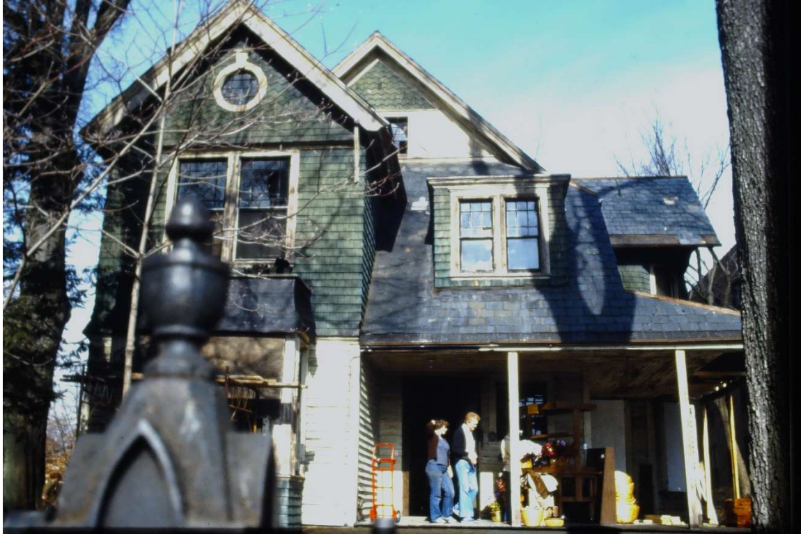
Façade/East Elevation under renovation, ca. 1980
