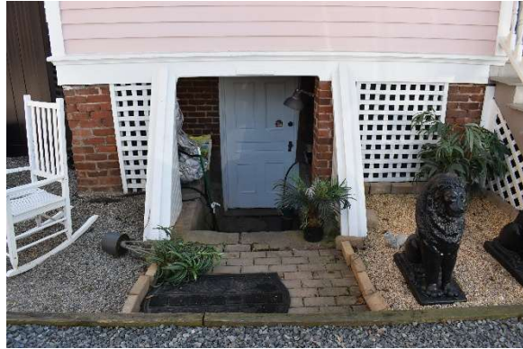
Door to cellar looking east
