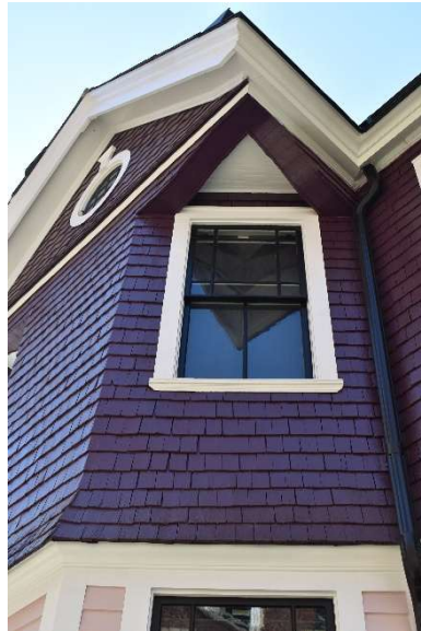
Window and gable eave detail in two-story bay section looking southeast
