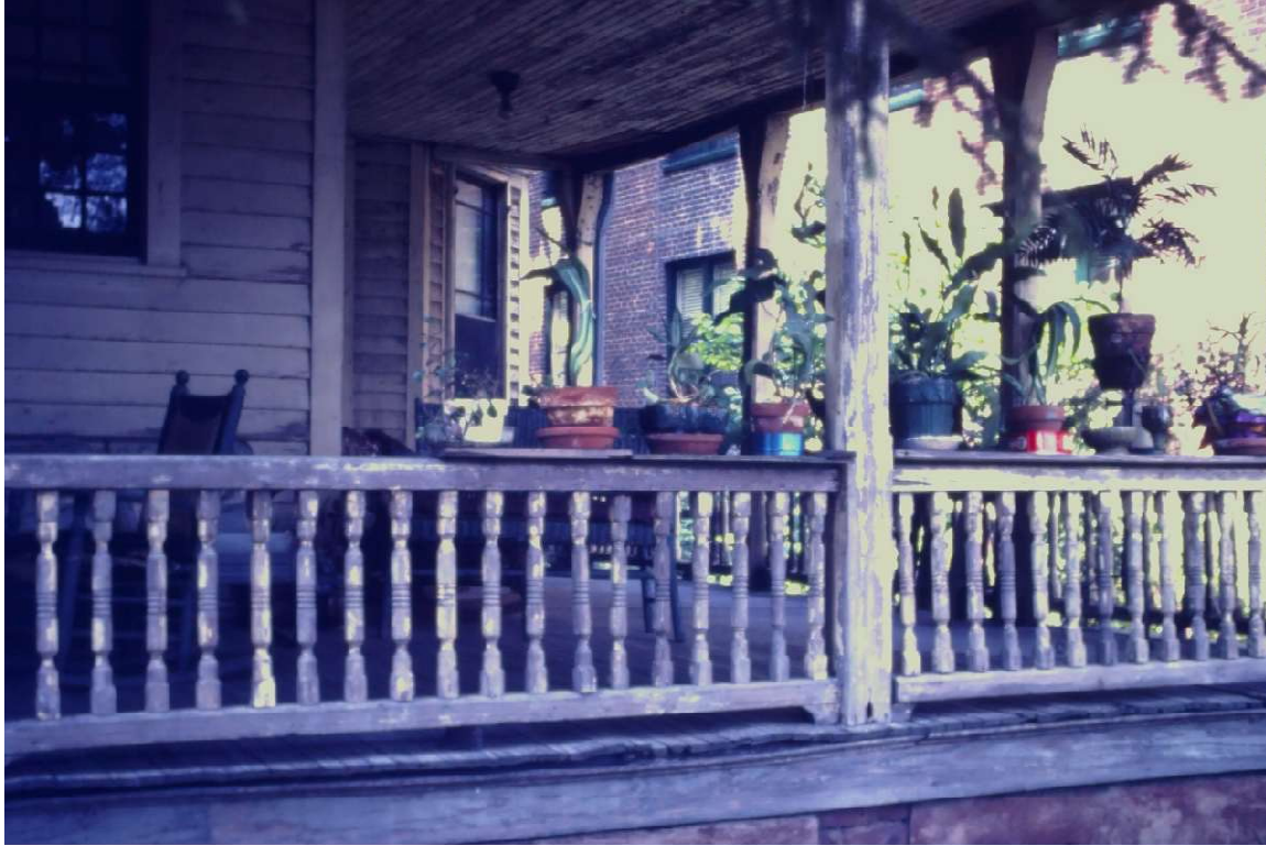
Porch at Façade/East Elevation looking North at Frederick Apartments, ca. 1975
