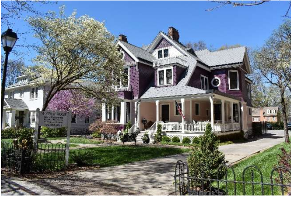
Looking southwest from northeast corner of property
