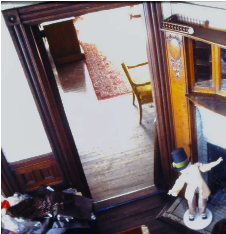
Looking from the Staircase in the Entry Hall to the West Parlor, ca. 1975
