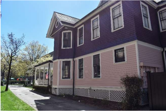
Looking southeast from north property line
