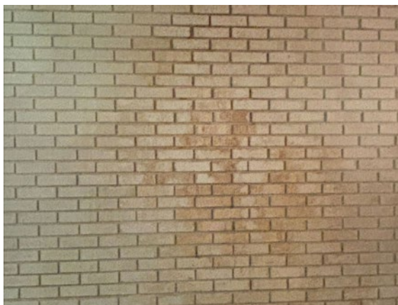
Figure 6: Cream Brick in Lower-Level Office Space
