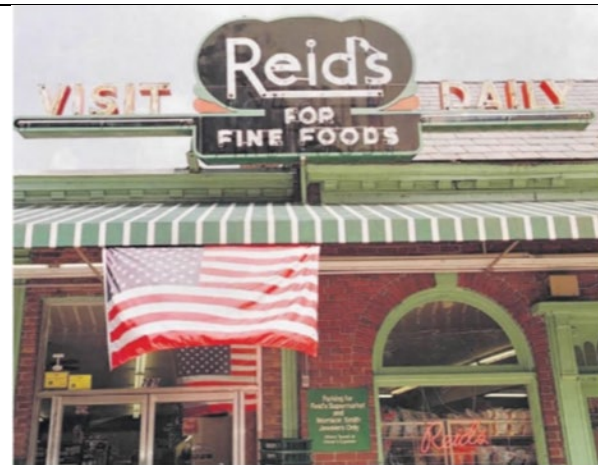
This Reid's sign is one way businesses look to preserve the city's history - by keeping and rehabilitating old signage.
