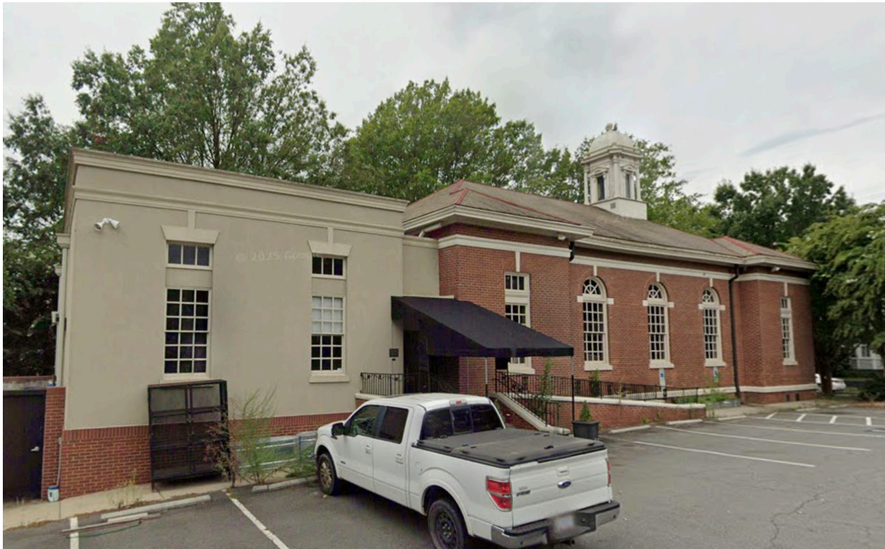
14. Additional view of northeast elevation in 2022.
