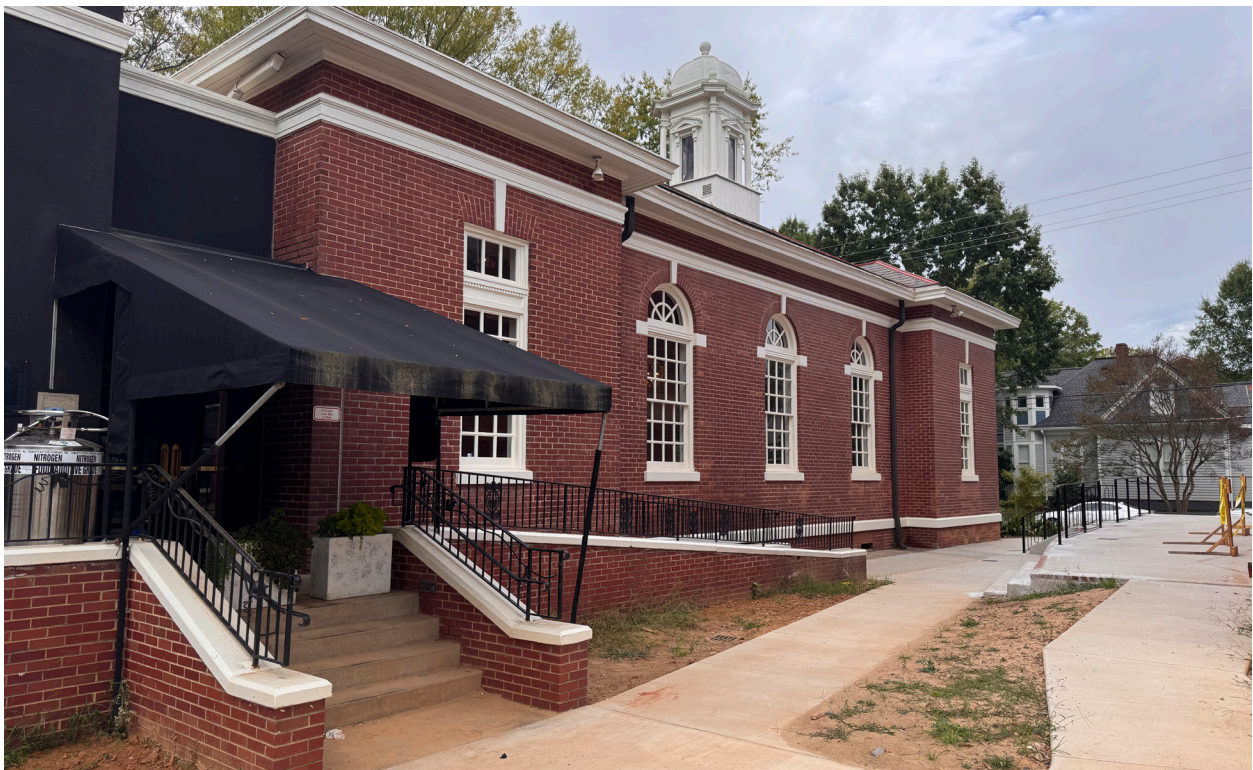
4. Looking northwest, view of the northeast elevation.
