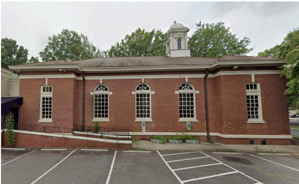
13. View of northeast elevation in 2022.
