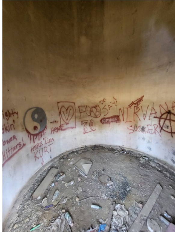
Above: Interior walls of north silo.
