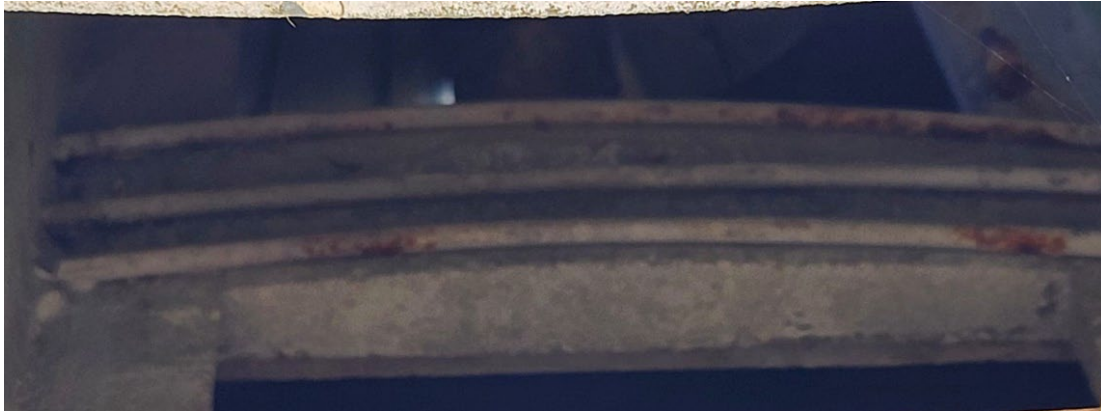
Above: One of the concrete lintels within the north silo's front elevation poured concrete frame that spans the silo's continuous door. Note the reinforcement hoops.
