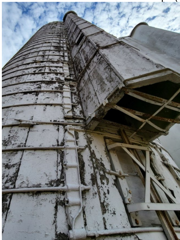
Above : Detail of poured concrete frame on north silo's front/west elevation. The top opening features the only remaining unloading door in the silo's continuous door. Below : Views of north silo's poured concrete frame showing placement of the chute and anchor fixtures for reinforcement hoops (left) and detail of an anchor fixture (right).
