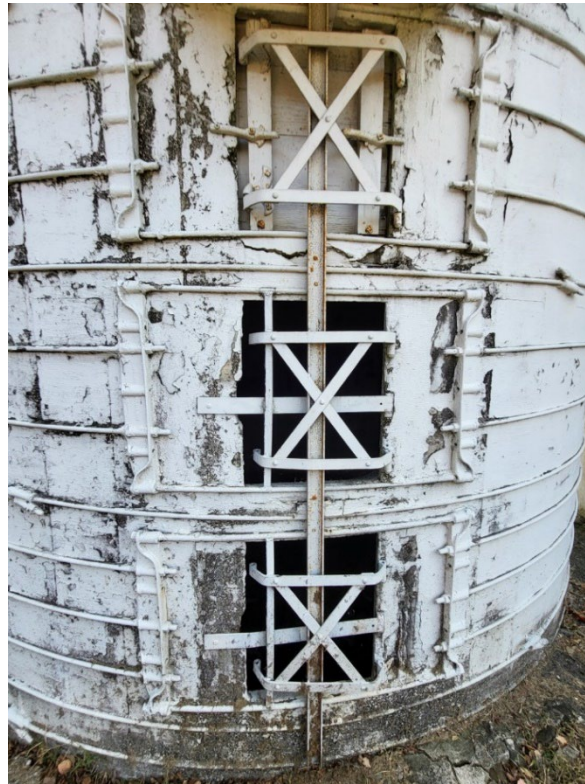
Above : Detail of poured concrete frame on north silo's front/west elevation. The top opening features the only remaining unloading door in the silo's continuous door. Below : Views of north silo's poured concrete frame showing placement of the chute and anchor fixtures for reinforcement hoops (left) and detail of an anchor fixture (right).
