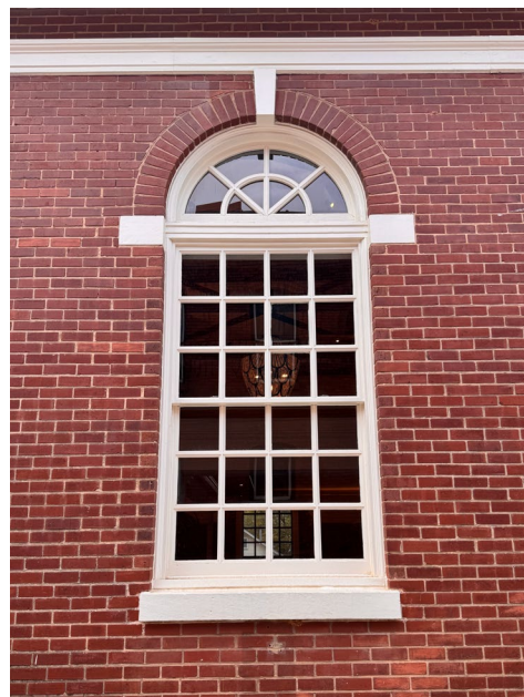
Figure 9. Current photograph of building window and belt coursing.
