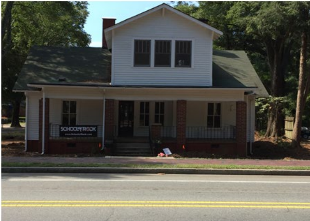
EXISTING FRONT - DOMINANT FEATURE OF OVERSIZED DORMER
