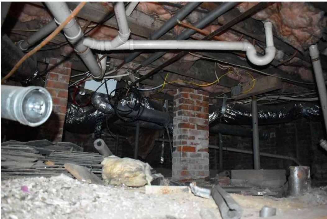
The brick foundation was insufficient to support the house, and metal posts were installed ca. 2003 as reinforcement.
