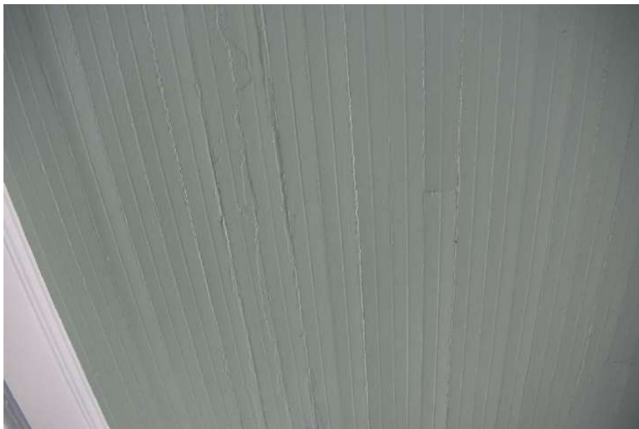
Beadboard wood ceiling at the front porch.
