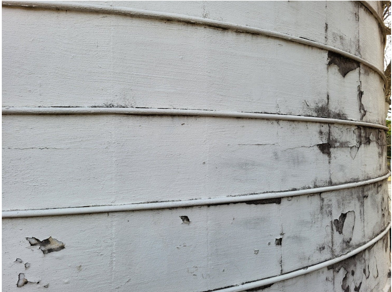
Below: Detail of south elevation of north silo showing its concrete stave and steel reinforcement hoop construction.
