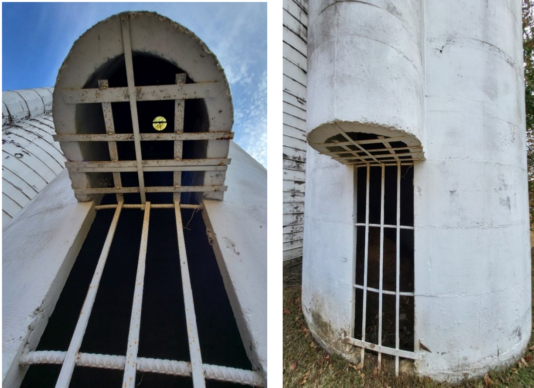
Chute opening (left) and bottom portion of continuous door (right), both on the south silo's front/west elevation.
