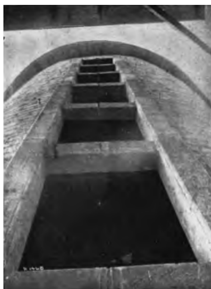
Above and below: Illustrative images of a poured concrete frame for a concrete stave silo. 59
