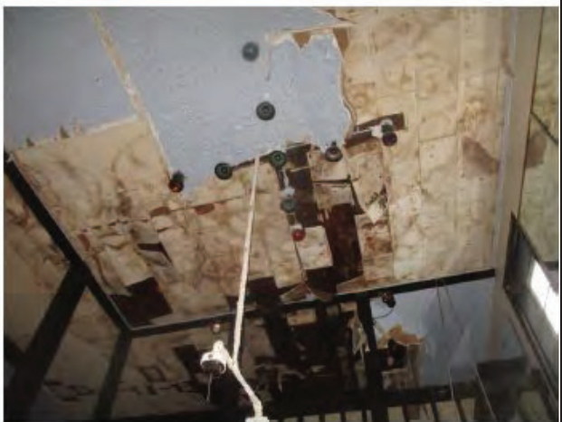
Damage to second floor ceiling finishes
