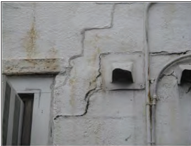
Typical exterior cracking
