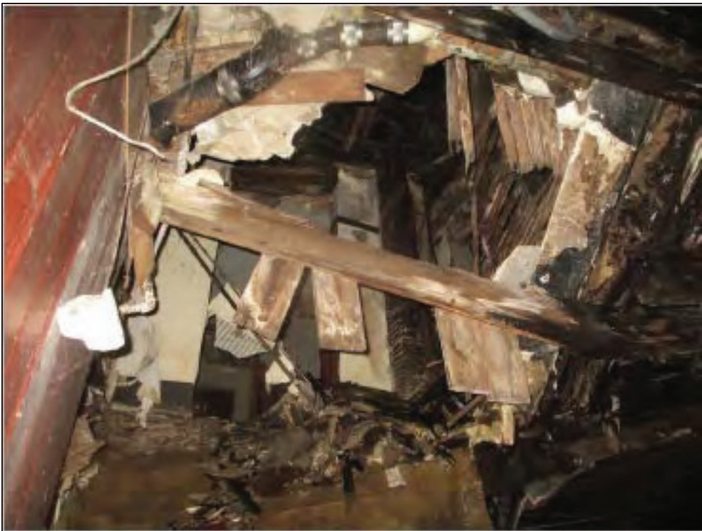
45 - Collapsed framing
