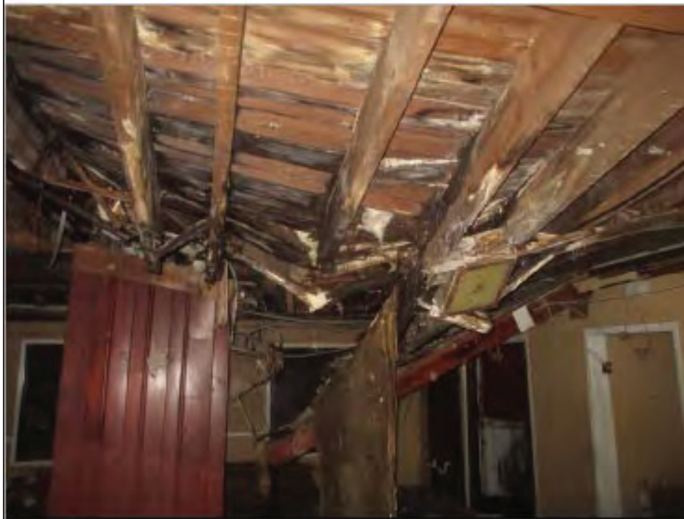
40 - Partially collapsed second floor, heavy damage
