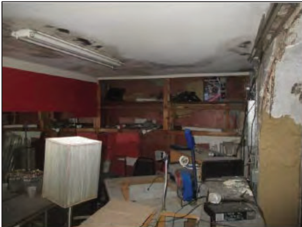
Typical damage to interior finishes
