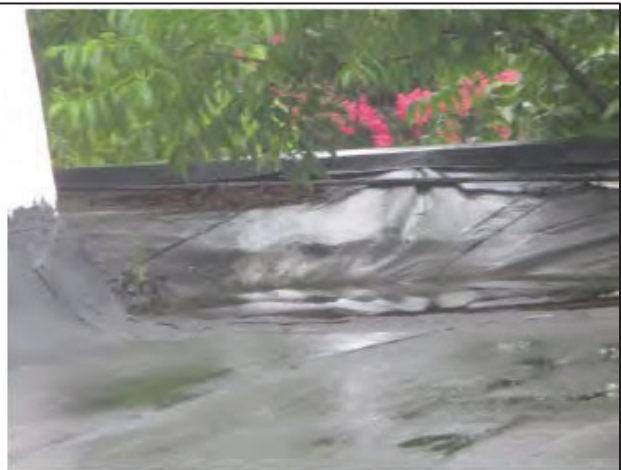
Low roof apparent collapse area
