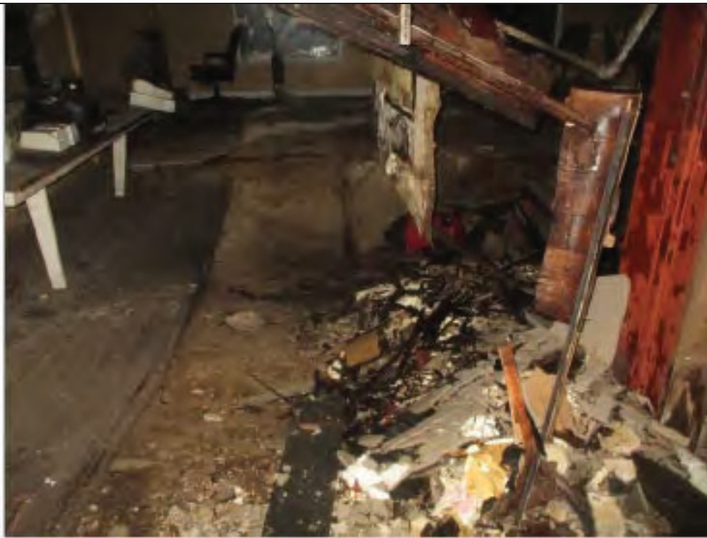
43 - Collapsed area of first floor
