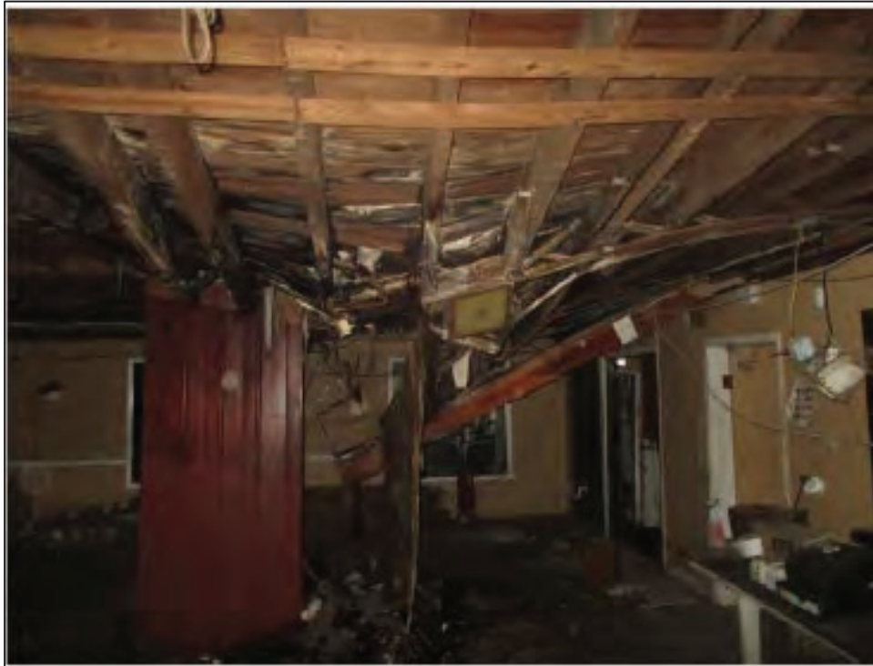
39 - Interior showing partially collapsed second floor
