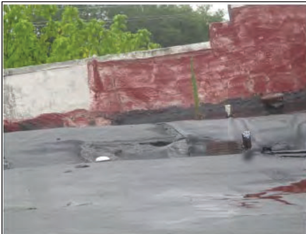
High roof apparent partial collapse, note the sloped front parapet
