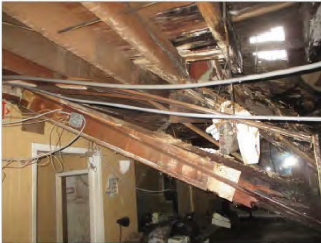
44 - Collapsed framing
