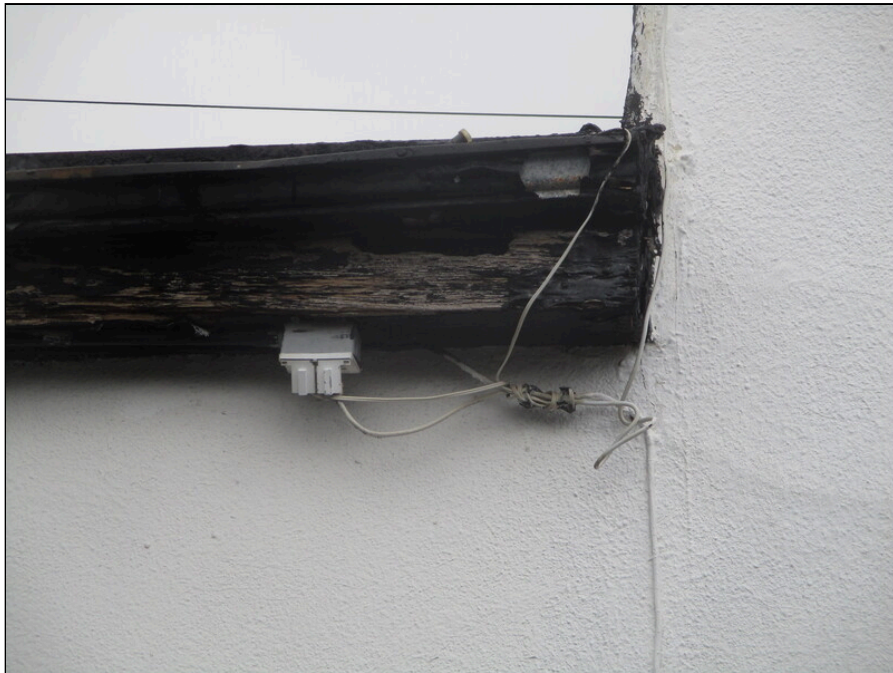
26 - Typical deteriorated wood rake edge
