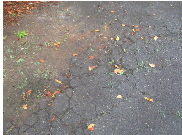
Typical pavement distress, failed overlay
