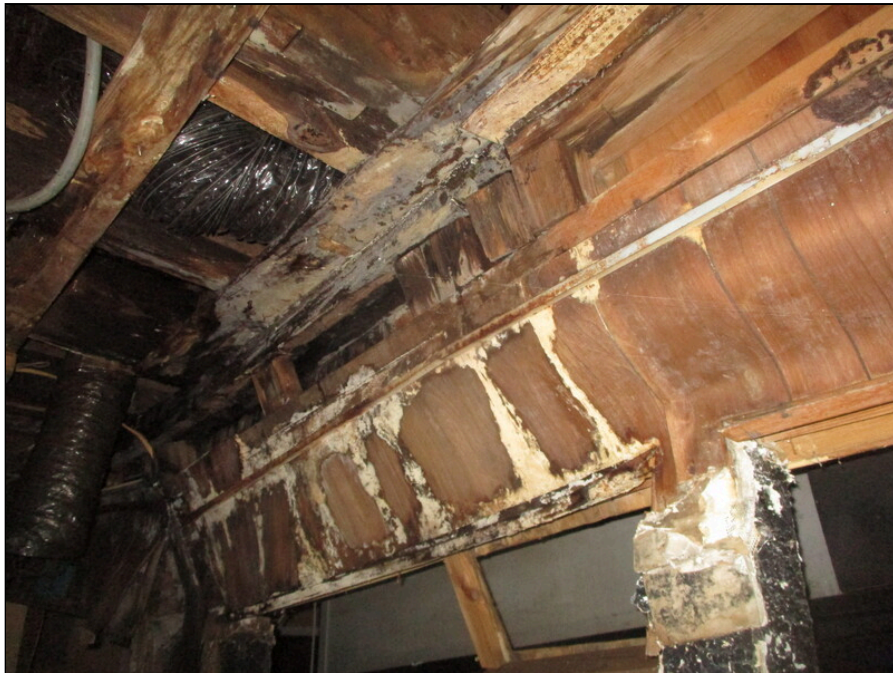
52 - Typical damaged framing and finishes, partial ductwork
