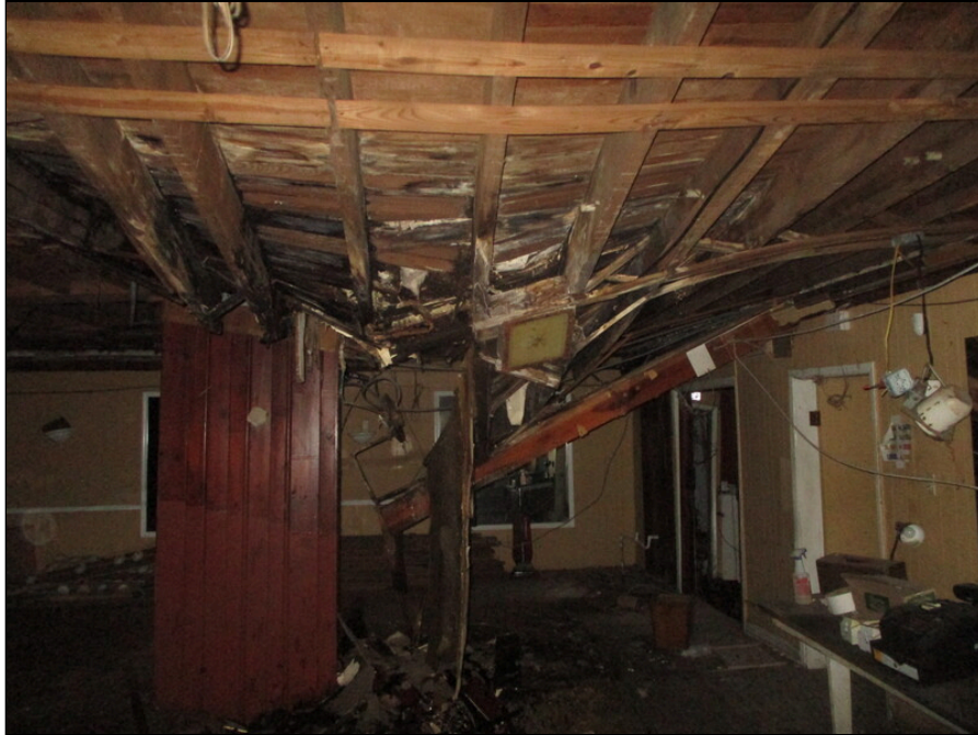
39 - Interior showing partially collapsed second floor
