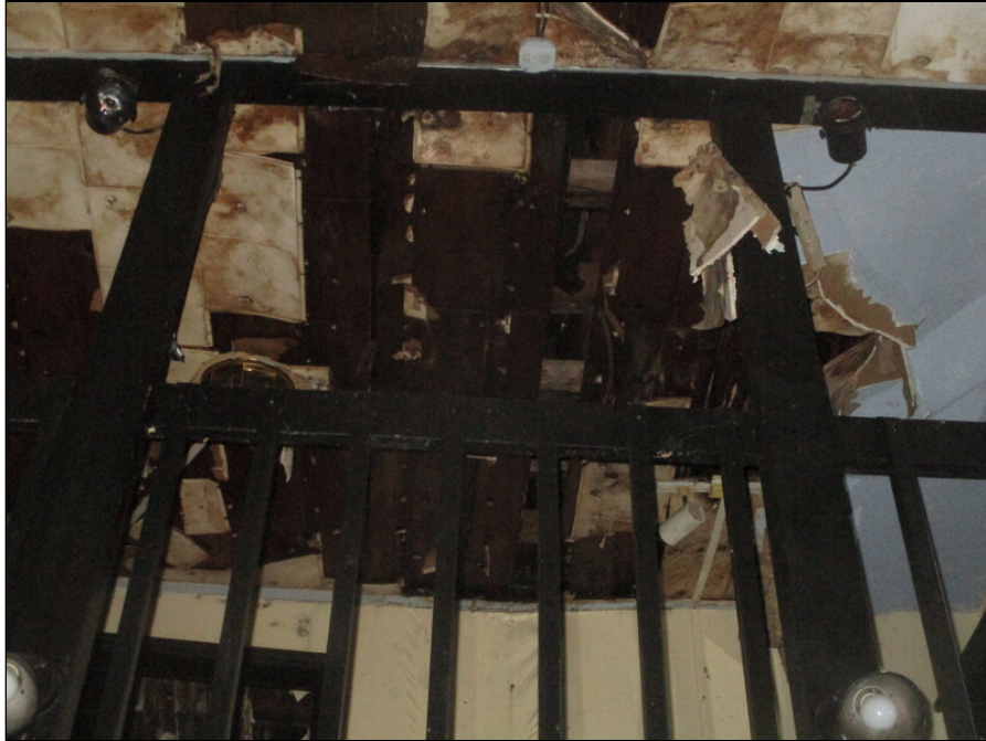
61 - Damage to second floor ceiling finishes
