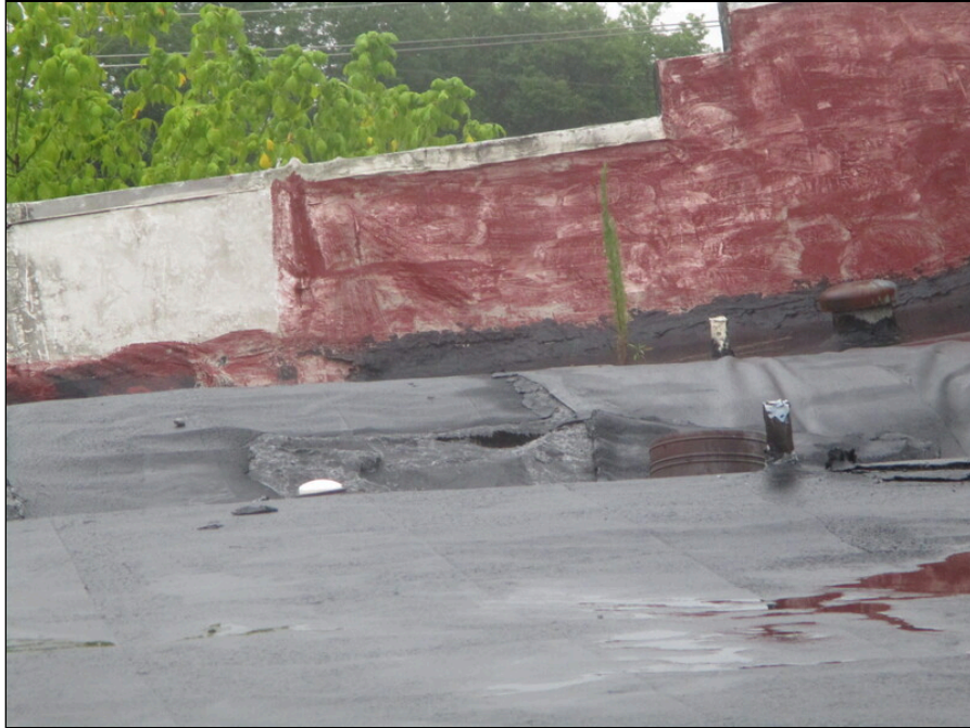
23 - High roof apparent partial collapse, note the sloped front parapet
