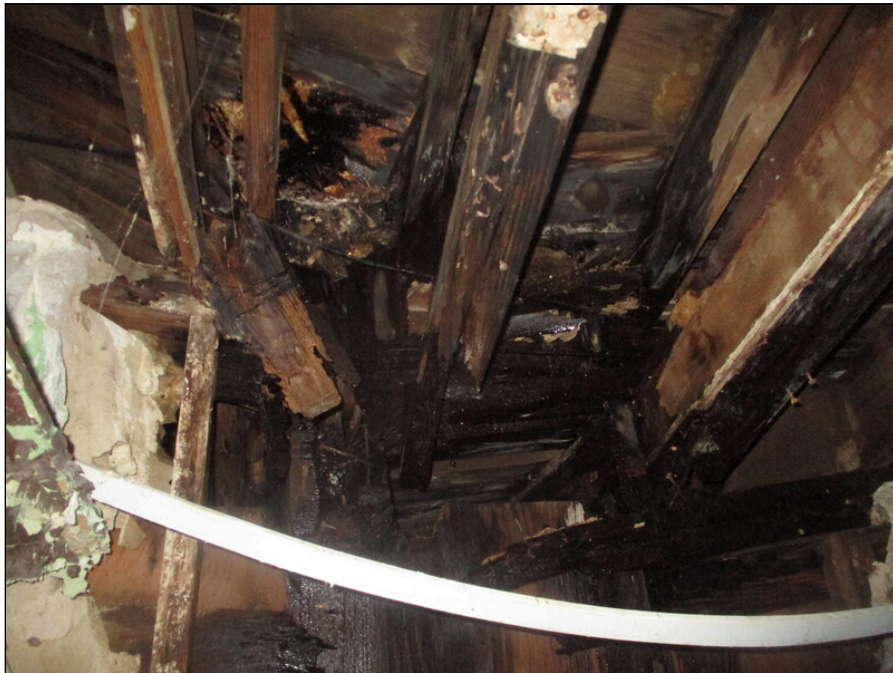
56 - Extensive wood rot due to long-term water infiltration
