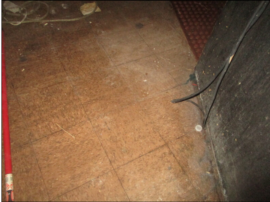
59 - Apparent 9x9 floor tile
