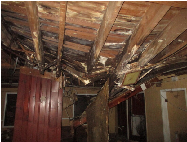
Partially collapsed second floor, heavy damage
