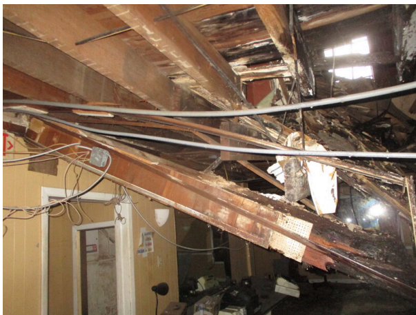
Collapsed framing
