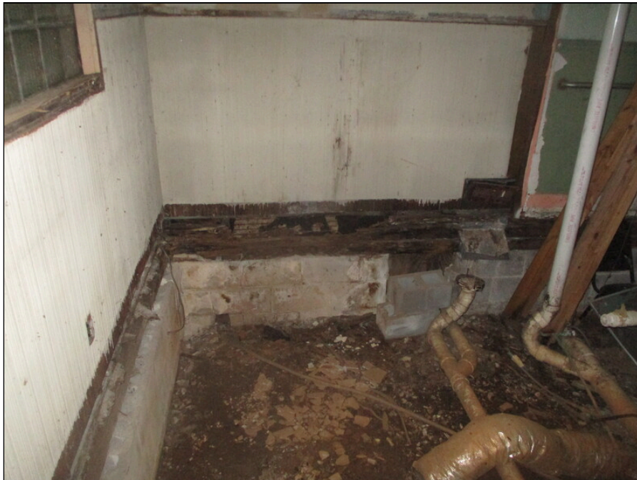
48 - Area at east elevation previously demolished, PVC piping remnants, damage at foundation wall
