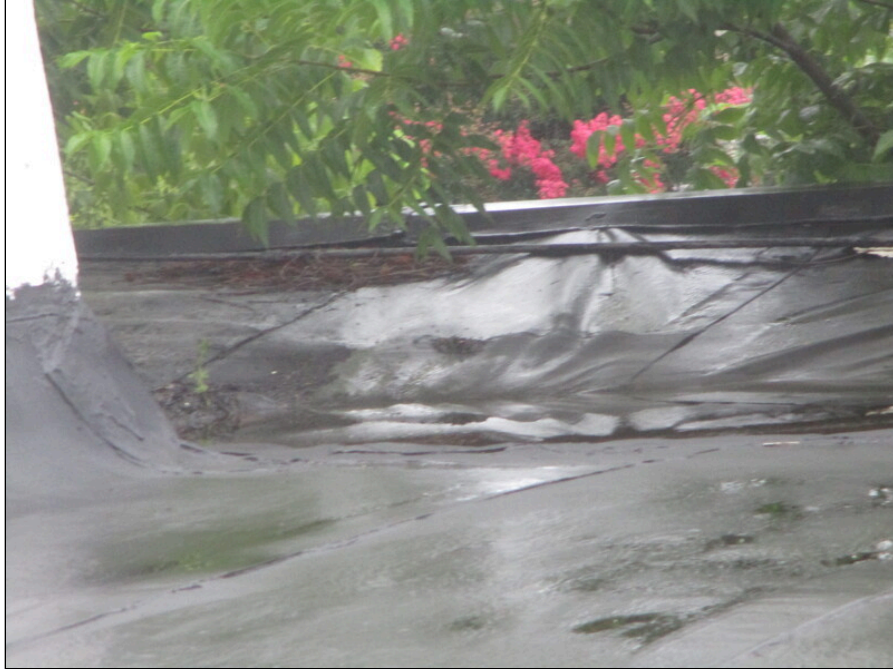
25 - Low roof apparent collapse area
