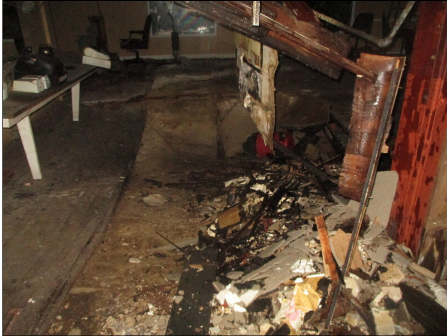
43 - Collapsed area of first floor
