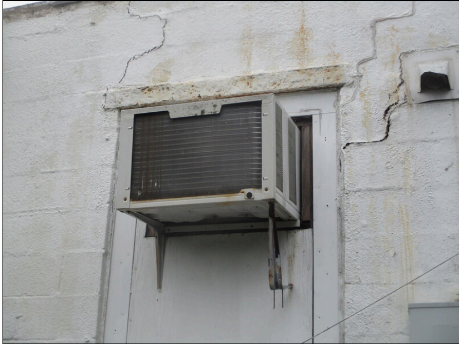
29 - Typical second floor air conditioner, wall cracking
