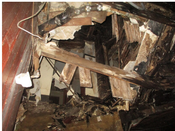
Collapsed framing
