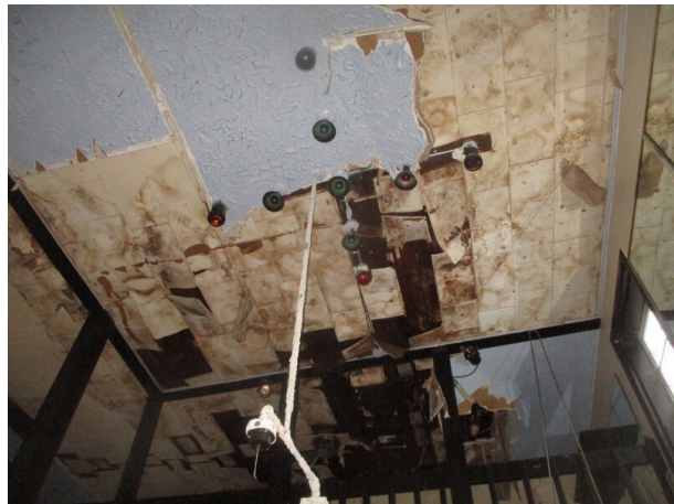
Damage to second floor ceiling finishes
