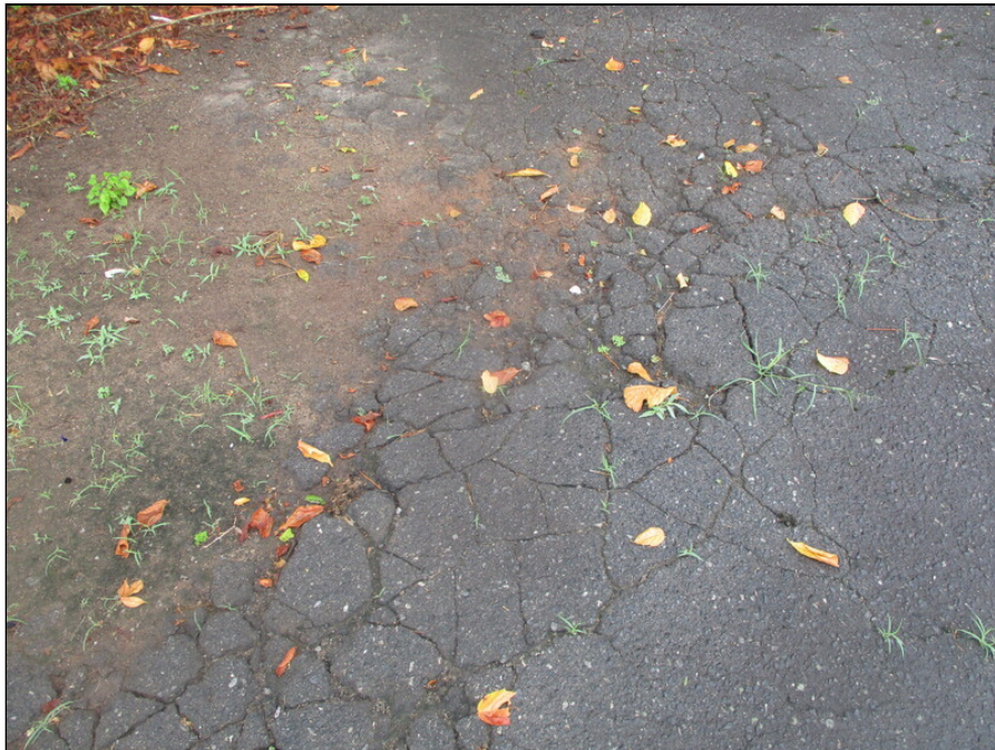
12 - Typical pavement distress, failed overlay
