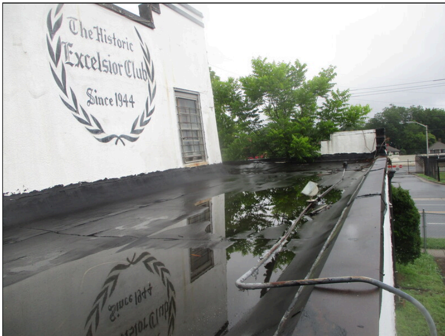
24 - Low roof overview, ponding
