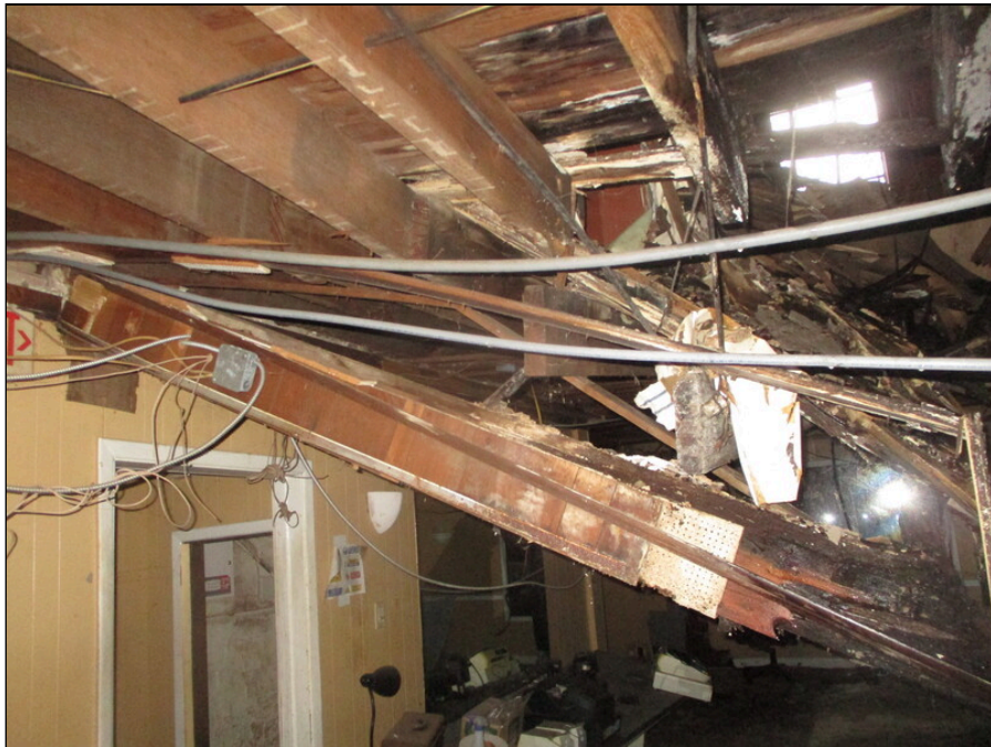
44 - Collapsed framing
