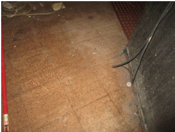
Apparent 9x9 floor tile
