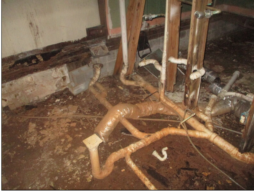
47 - Area at east end previously demolished, PVC piping remnants, damage at foundation wall
