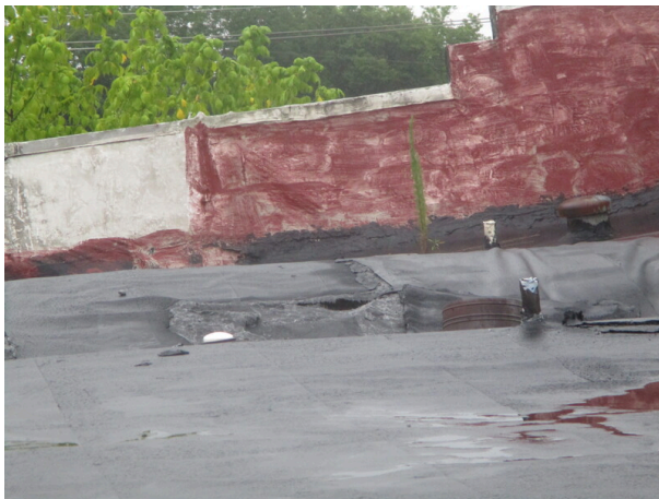
High roof apparent partial collapse, note the sloped front parapet
