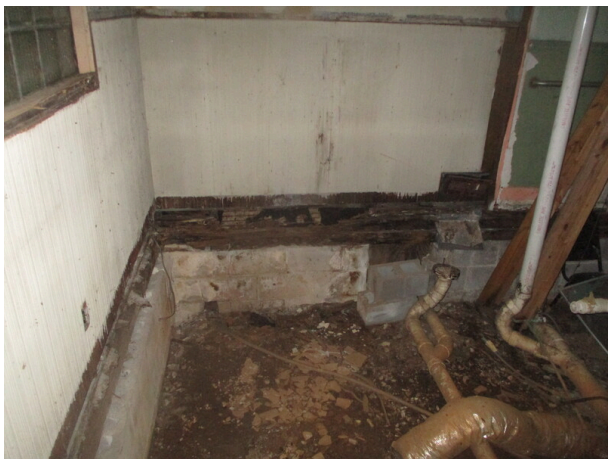
Area at east elevation previously demolished, PVC piping remnants, damage at foundation wall
