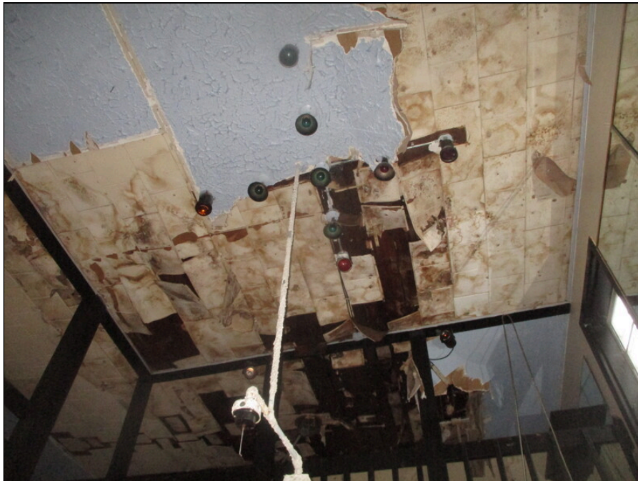
60 - Damage to second floor ceiling finishes
