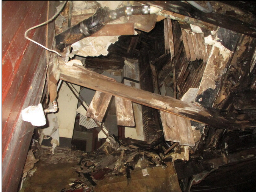
45 - Collapsed framing
