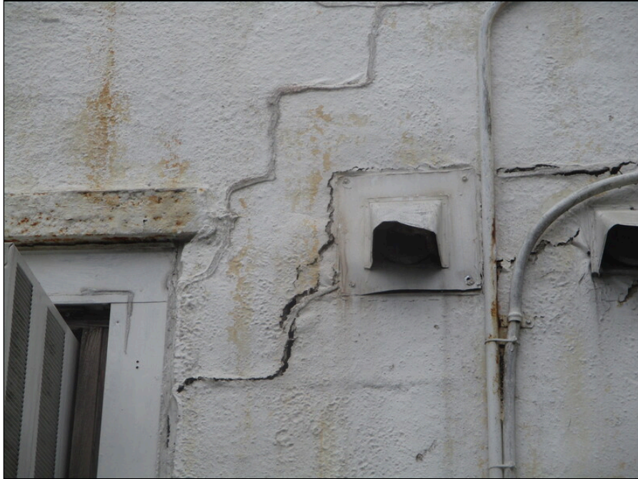
19 - Typical exterior cracking
