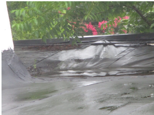
Low roof apparent collapse area
