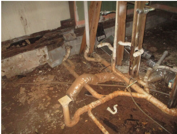
Area at east end previously demolished, PVC piping remnants, damage at foundation wall
