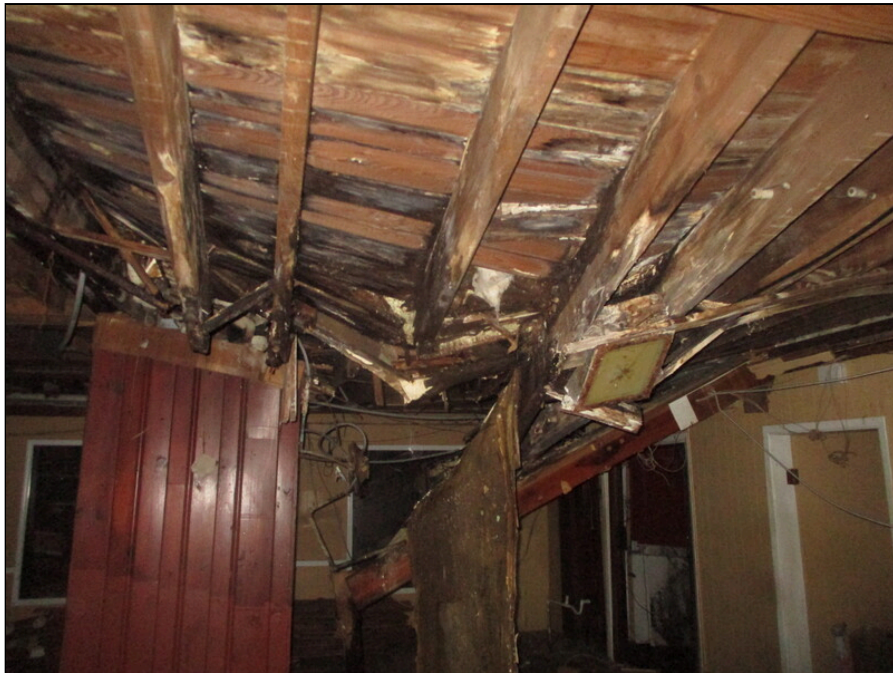
40 - Partially collapsed second floor, heavy damage
