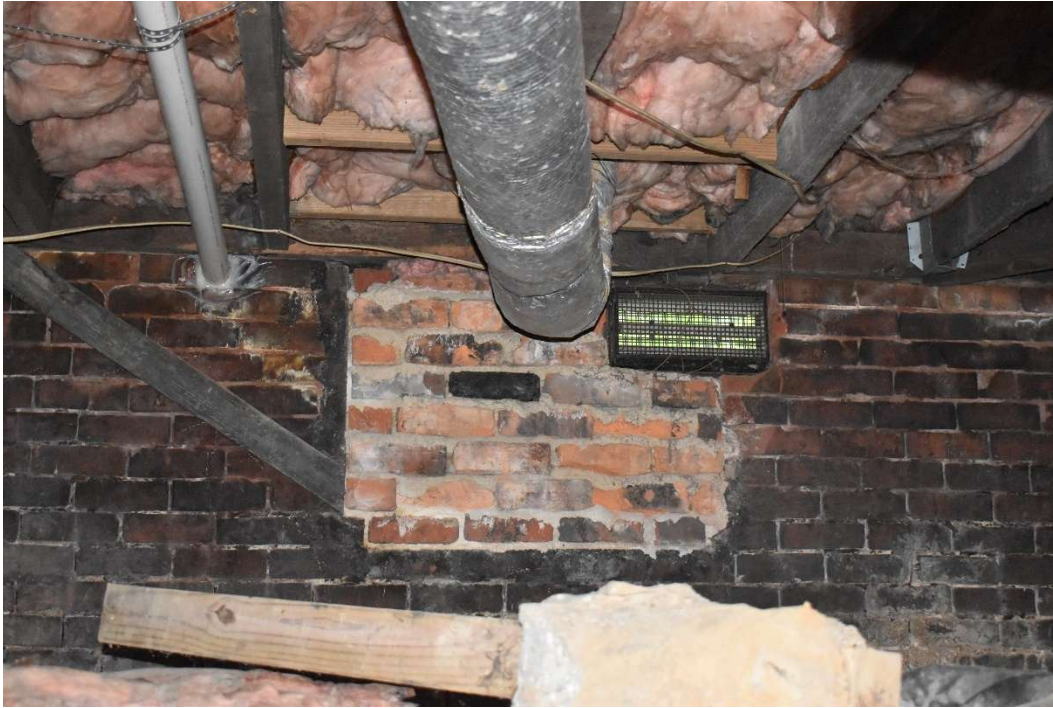
The coal chute was located on the north elevation along W. Ninth Street. It has been removed and infilled with brick.
