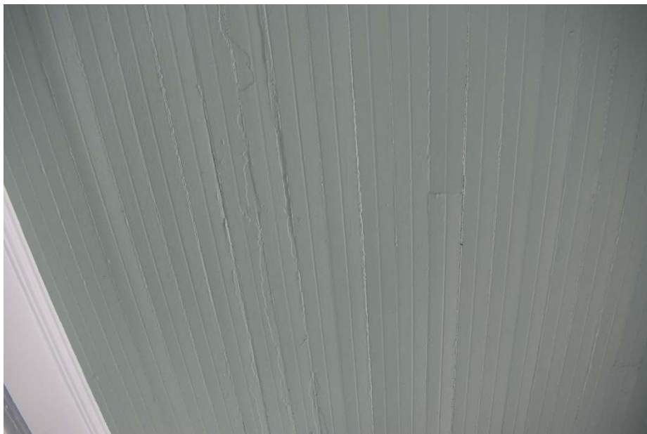
Beadboard wood ceiling at the front porch.
