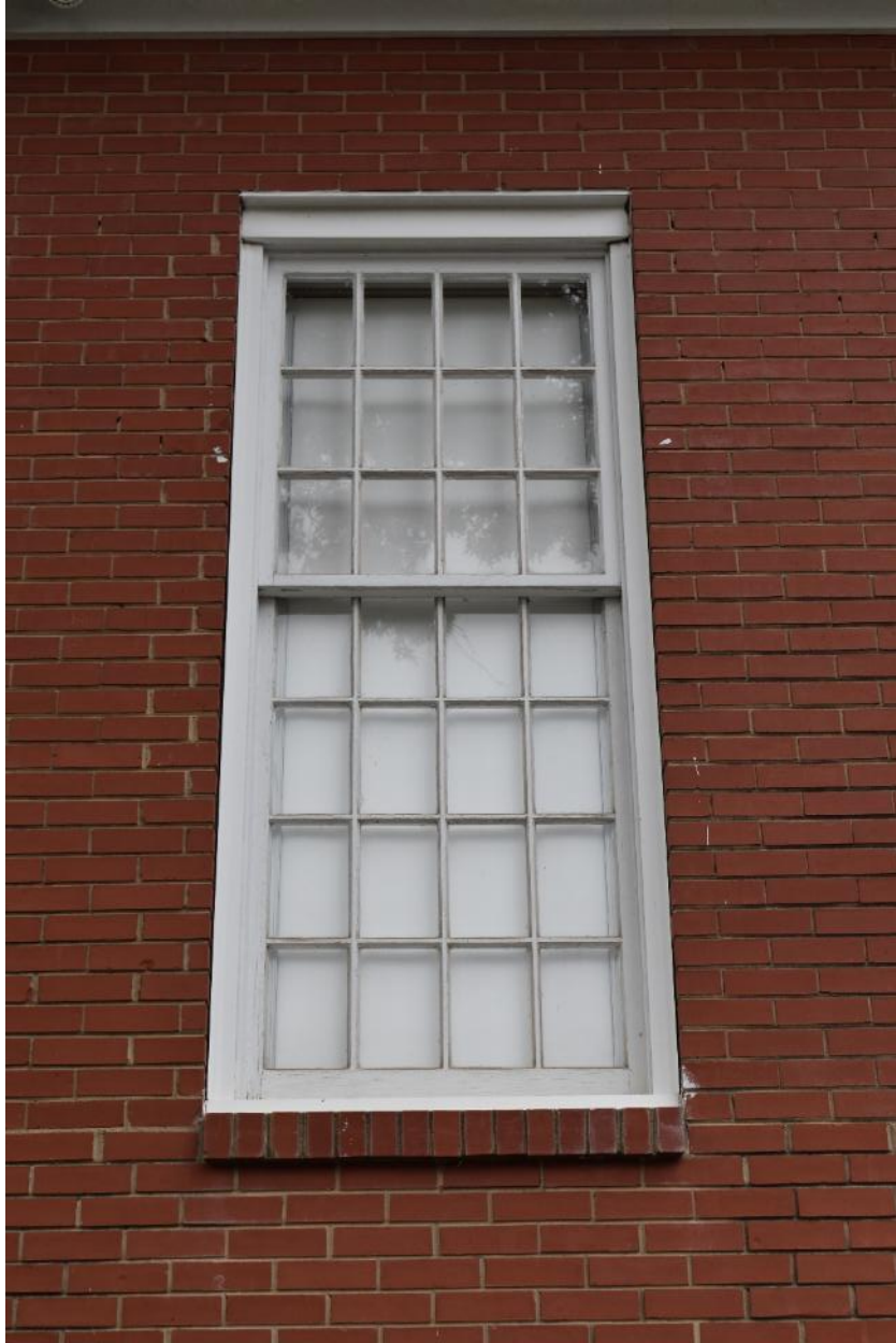
Typical twelve-over-sixteen wood sash window
