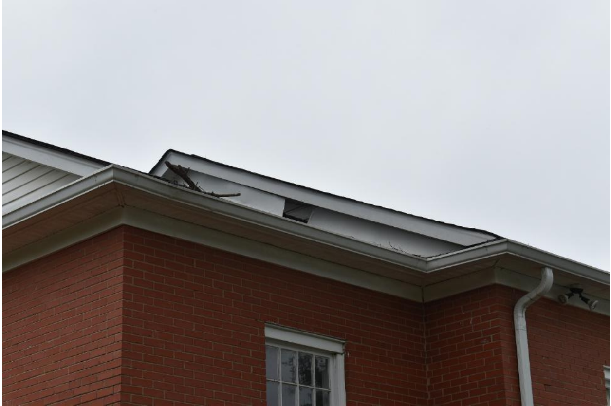
The original wood German siding of the gable is visible through missing trim.
