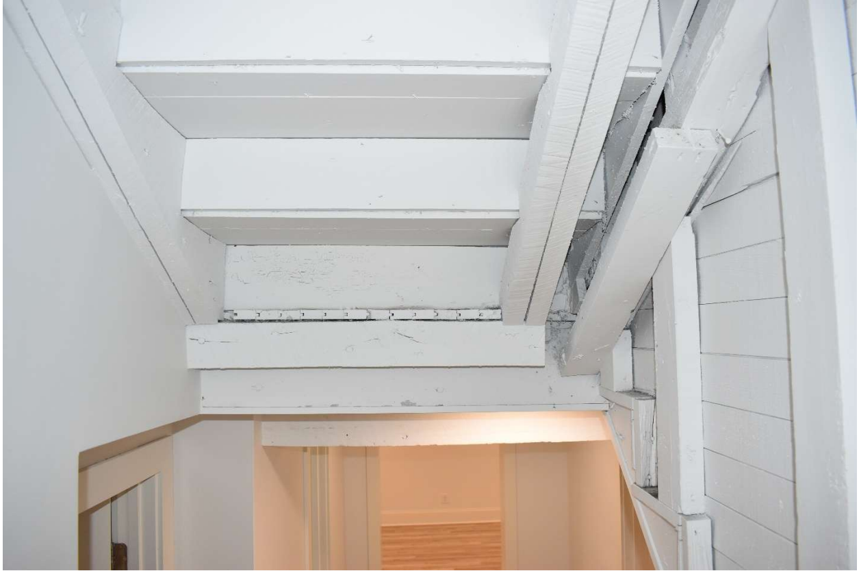
Structure of stairwell at basement landing.
