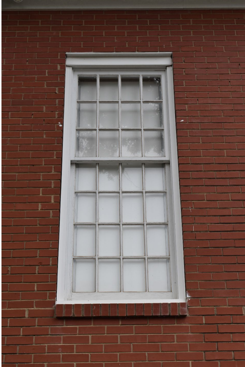
Typical twelve-over-sixteen wood sash window
