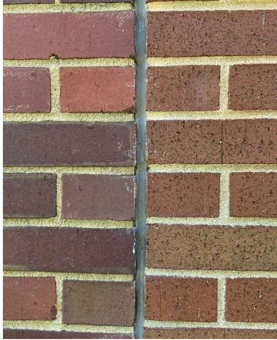
Close-up of the seam between the original building and the addition.
