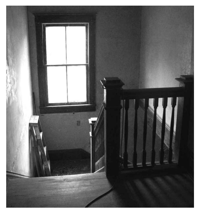
The remodeled rear wing is connected by a new door opening on the second story. The remodeled wing feature new woodwork that replicates the woodwork found in the original sections of the house.
