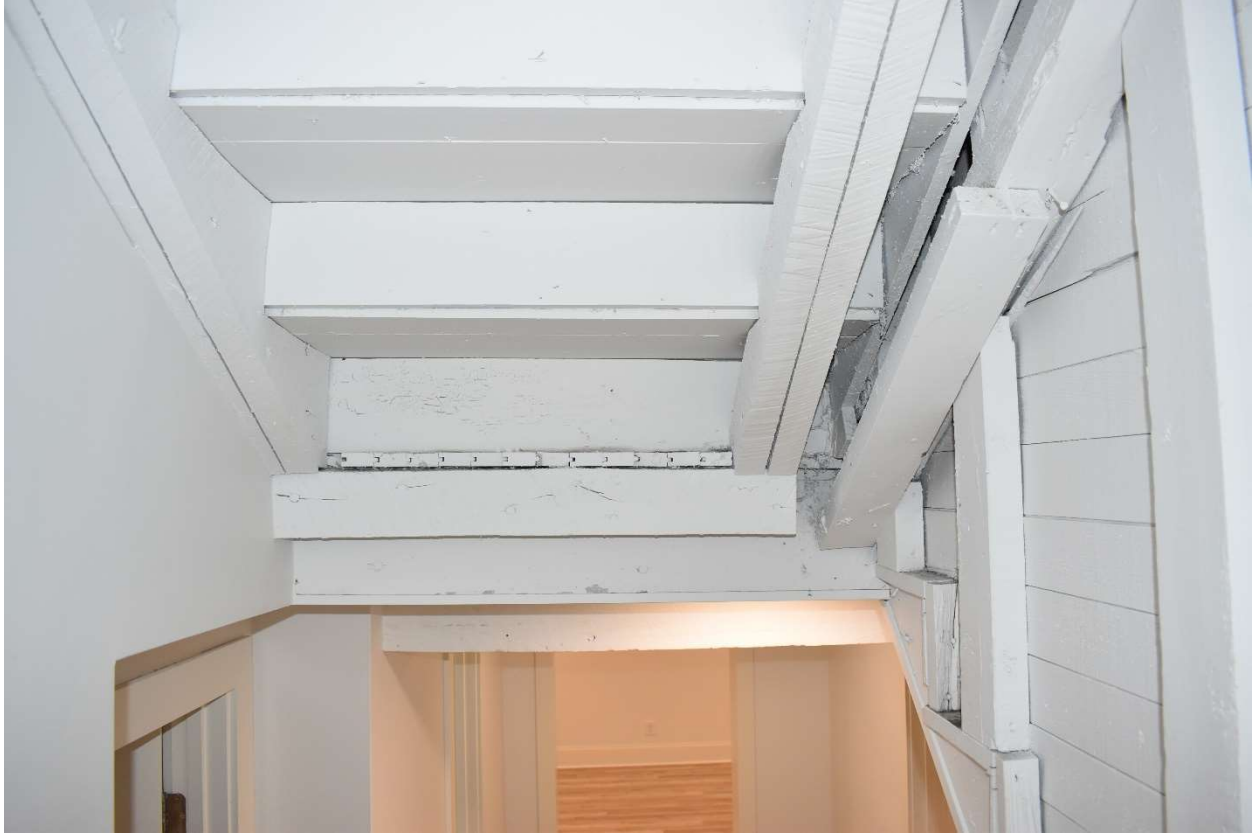
Structure of stairwell at basement landing.
