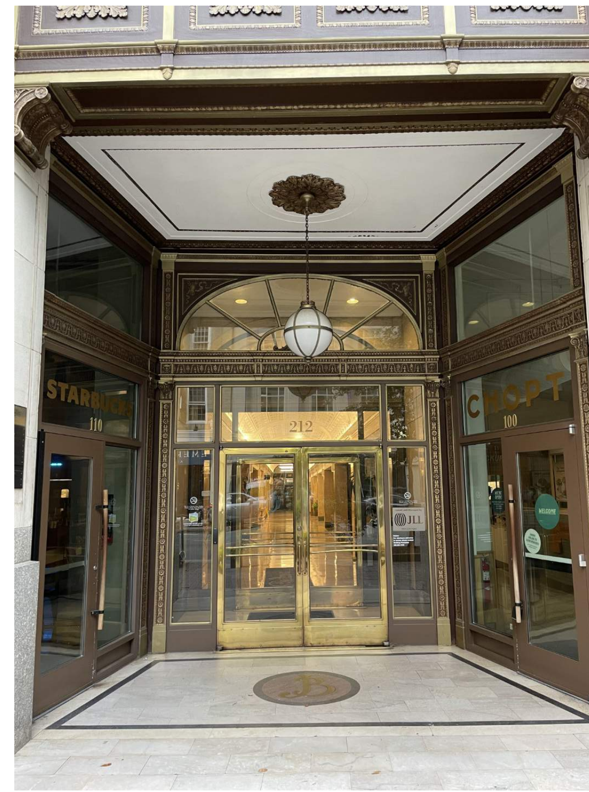
BUILDING EXTERIOR - MAIN ENTRY VESTIBULE
