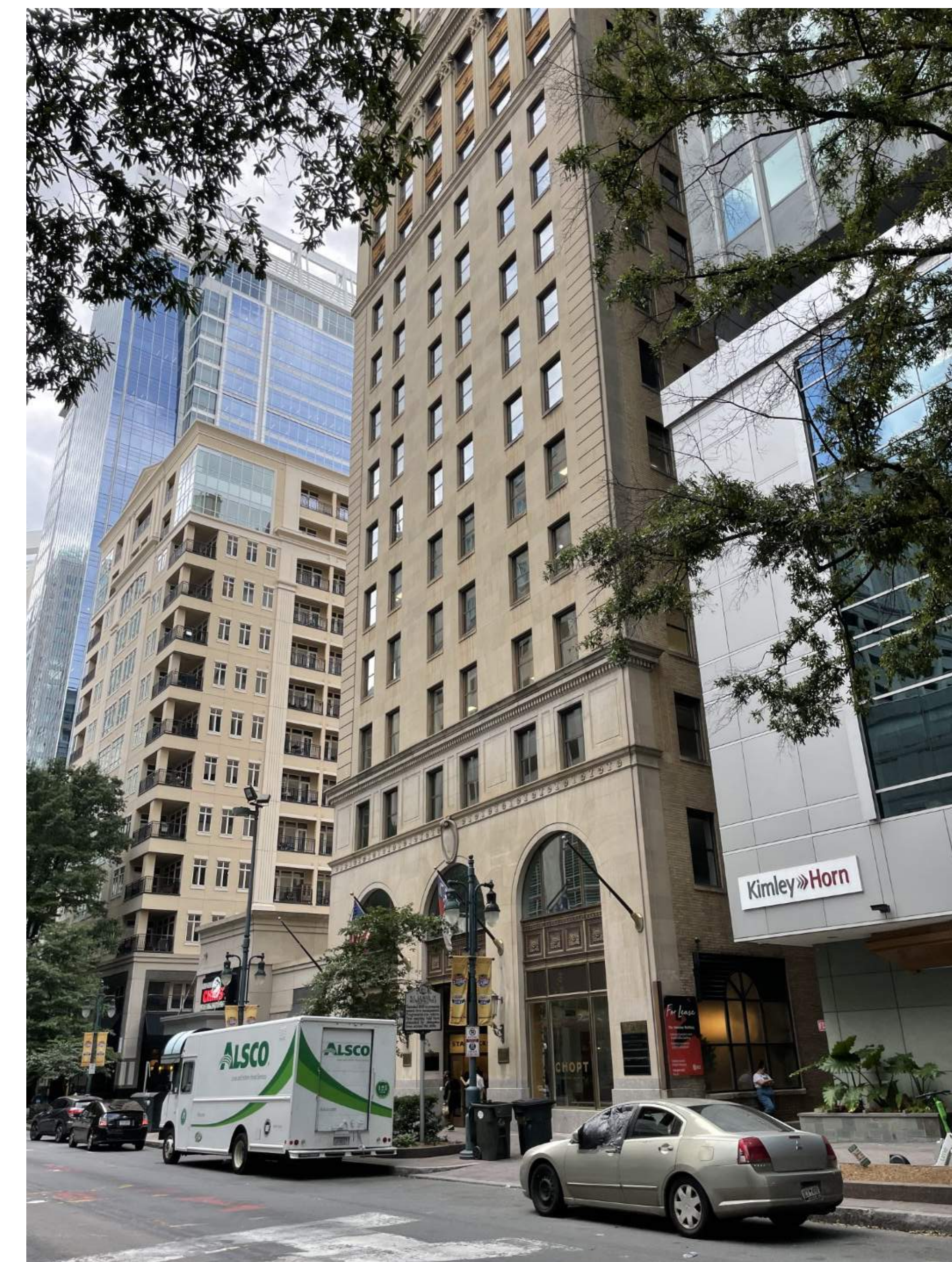
BUILDING EXTERIOR - SOUTH TRYON STREET, LOOKING WEST
