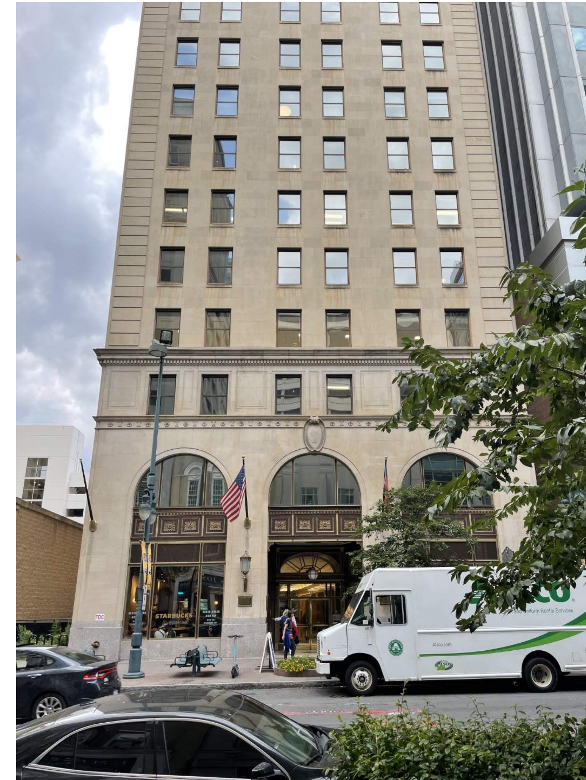
BUILDING EXTERIOR - SOUTH TRYON STREET, LOOKING NORTHWEST
