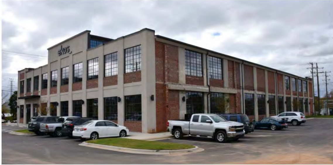
Rear/North Elevation and East/Left Elevation
