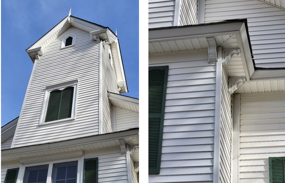
Details of design features of Coddle Creek Presbyterian Church, Mooresville
