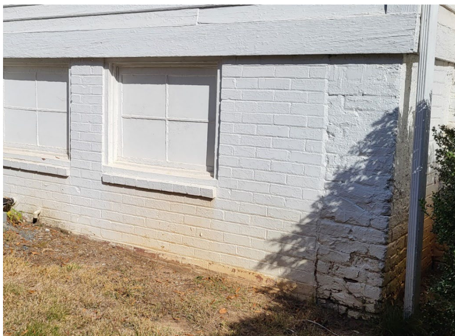
South elevation foundation.
