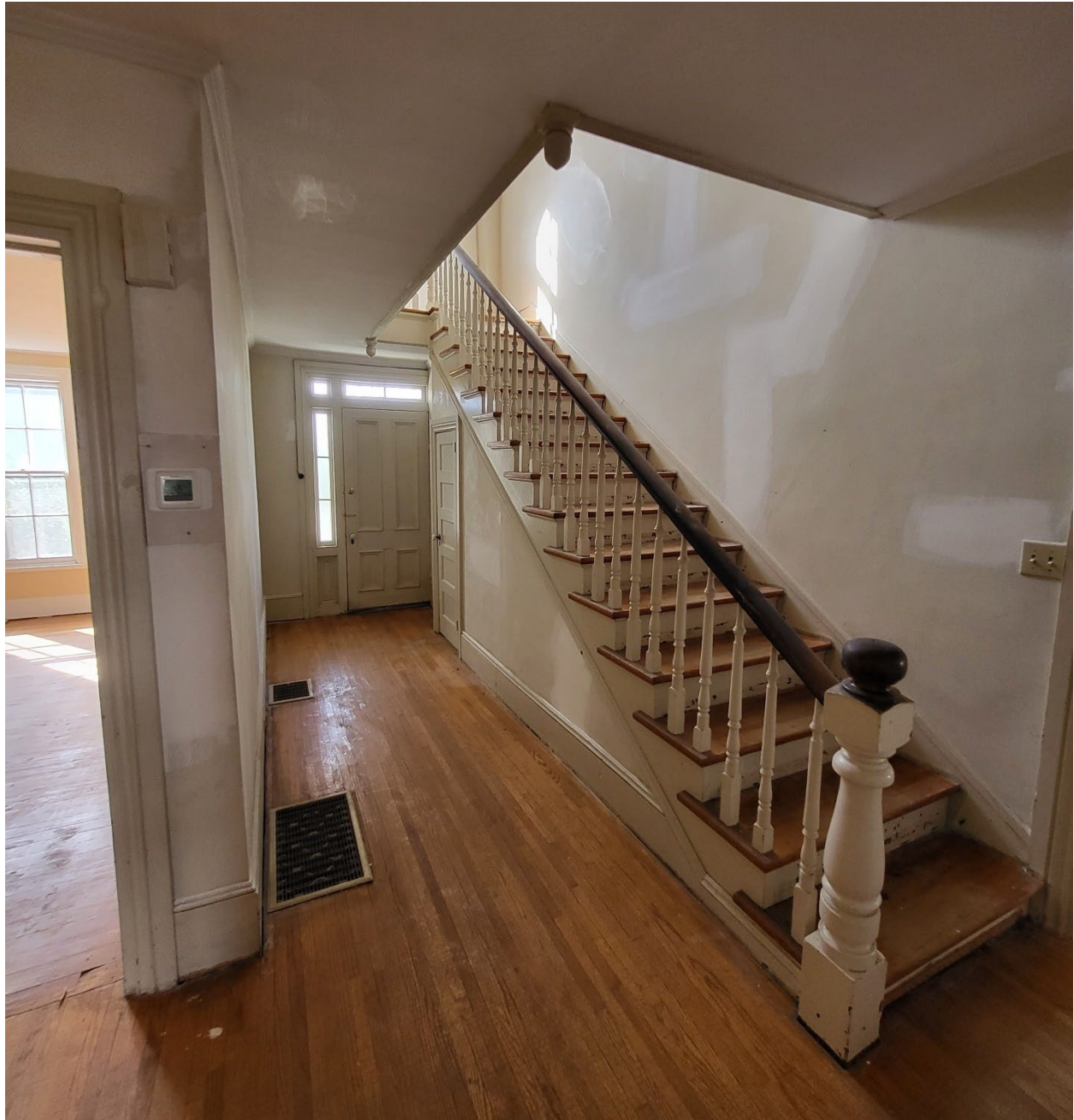
First floor stair hall and stairway. The doorway in the left foreground leads to the den. The door in the rear center is the south elevation entrance; to its right is the powder room door. Picture also shows illustrative original wood floors and crown and baseboard moldings typical throughout the house, as well as the acorn-shaped pendills.
