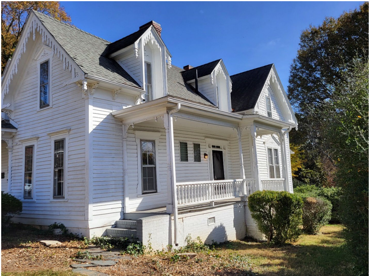
Front and south elevations.
