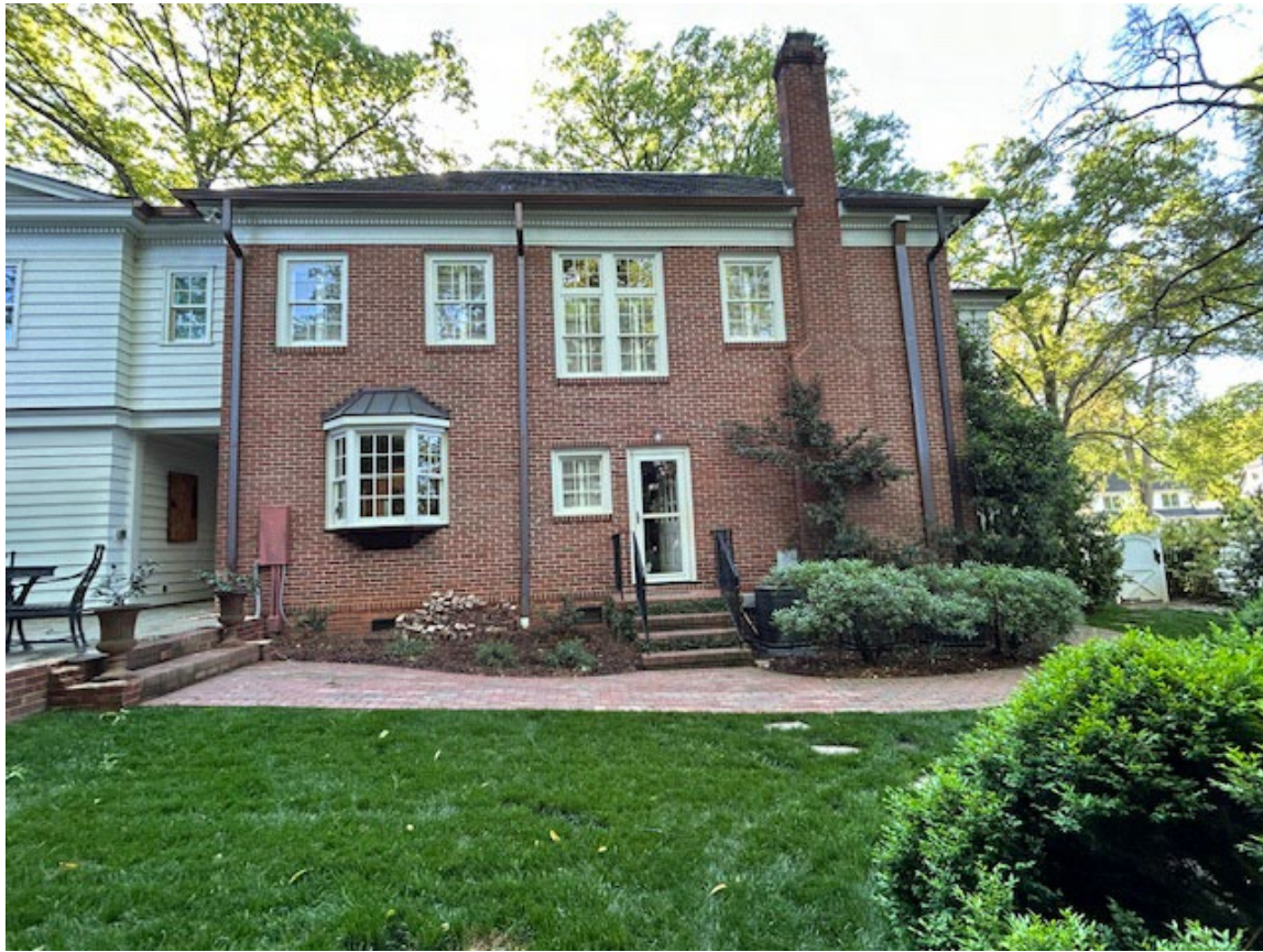
Photo 4: Rear (West) Elevation
