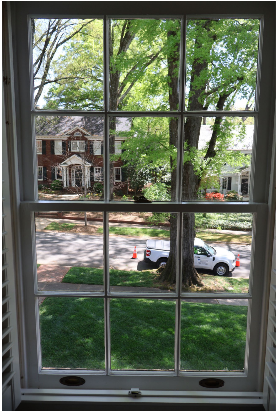
Photo 25: Window in Original House
