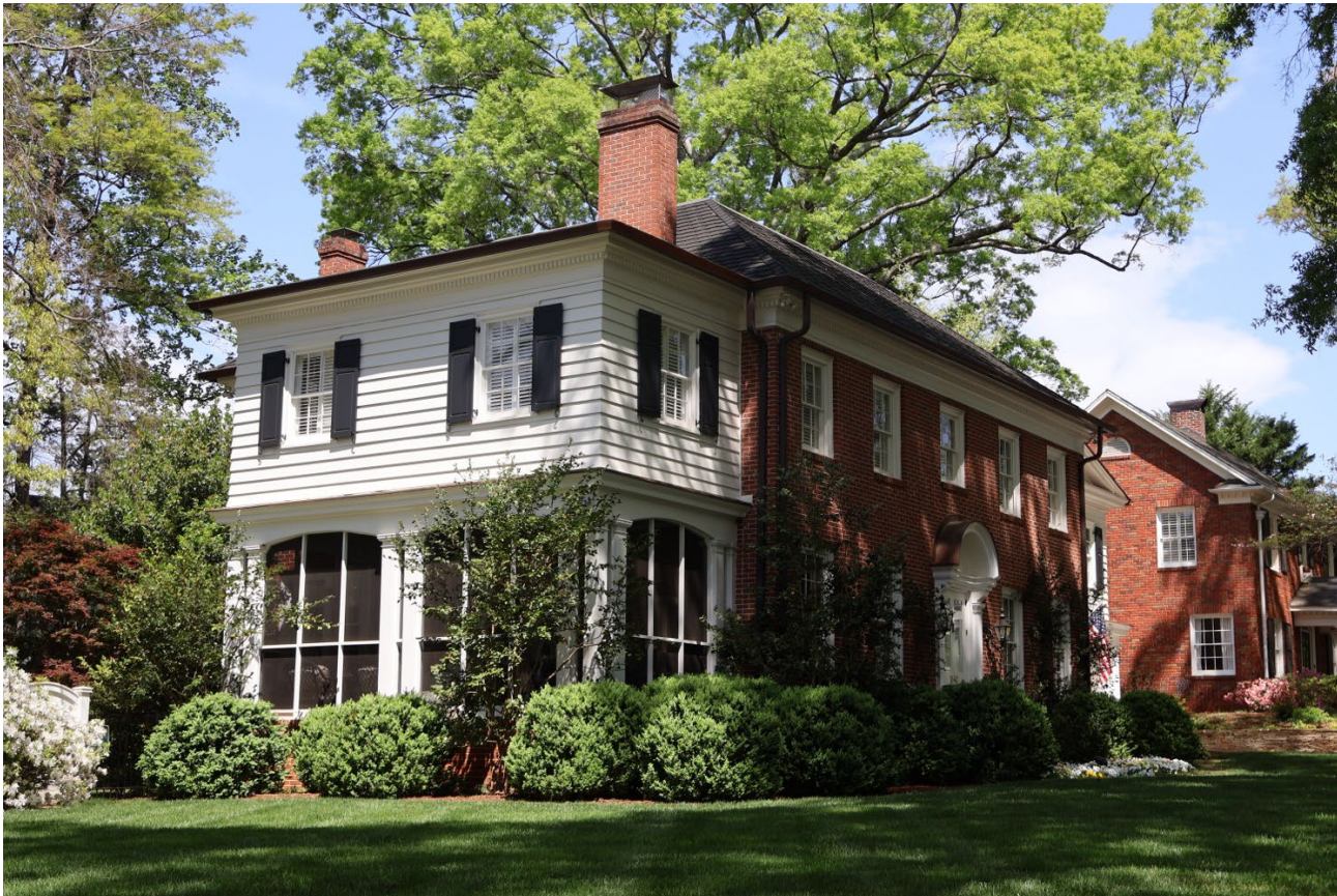
Photo 3: Side (South) Elevation
