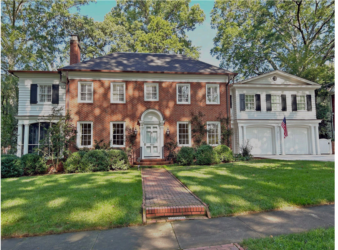
Photo 2: Front (East) Elevation
