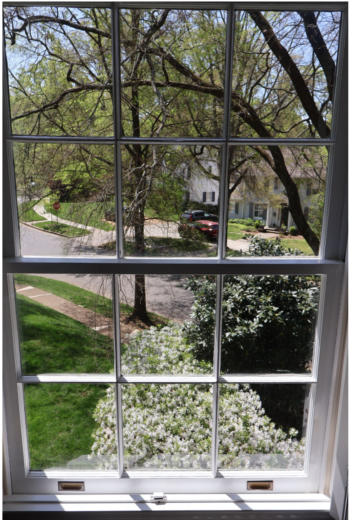
Photo 24: Window in 1947 Addition
