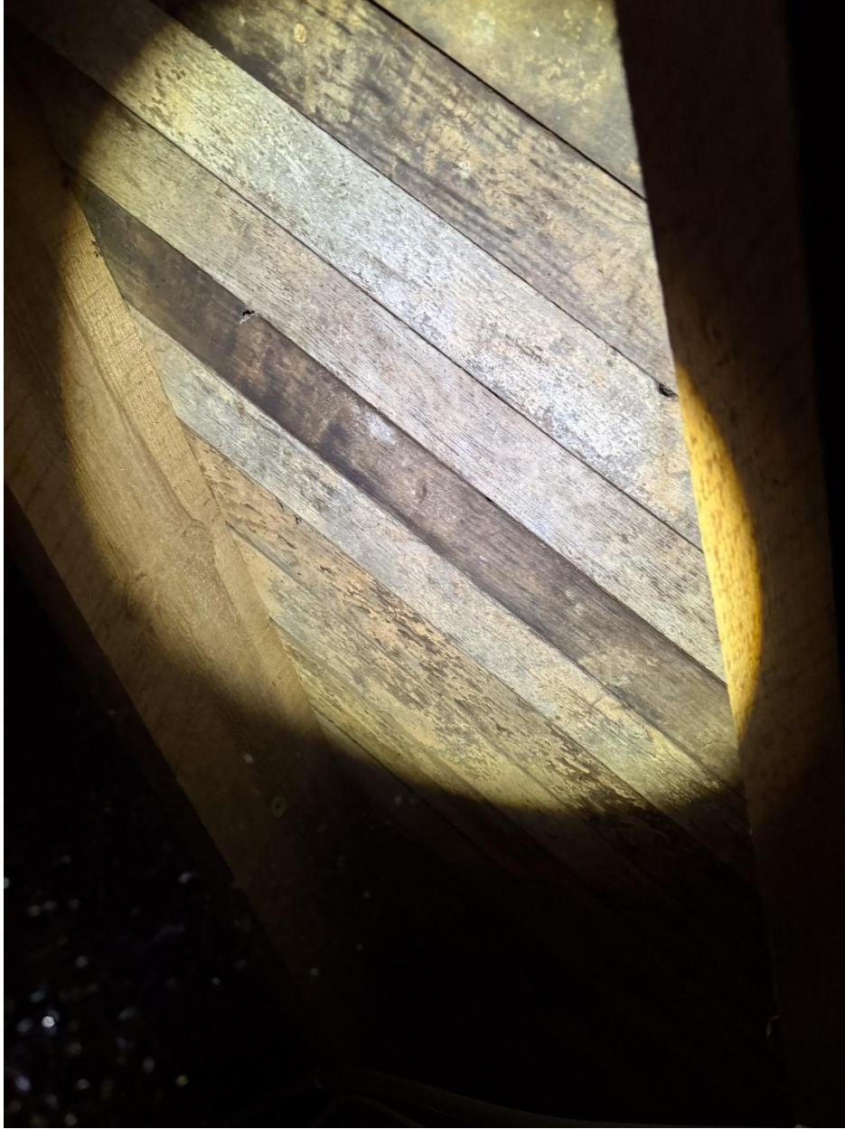
Figure 15 Looking up at the wood plank subfloor and wood joists at the west portion of the Caldwell-Bradford School in the crawlspace. This section was likely added later when the former school was converted into a residence.
