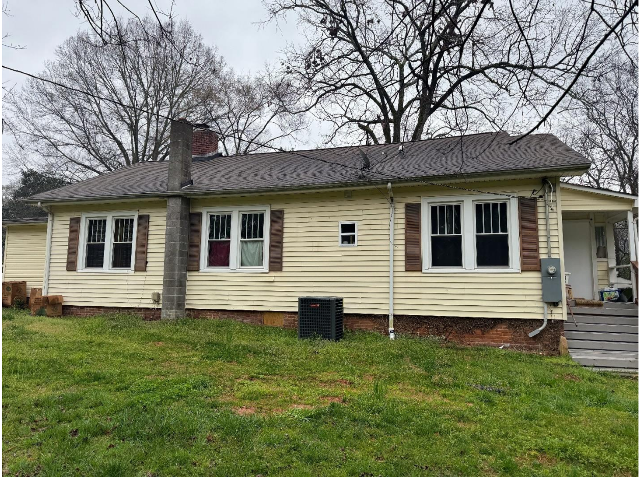
The west elevation of the Caldwell-Bradford School is three bays wide, each bay with a pair of replacement windows. The north and middle bays are divided by a replacement chimney.
