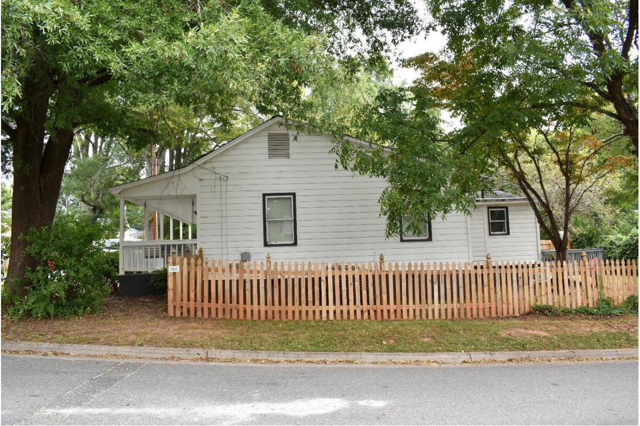
The west elevation of the Armour Street Mill House faces Watson Street. It is three bays wide, with the shed porch comprising the first bay. The middle bay is centered in the gable with large louvered vent above a typical window, and the third bay has a typical window.
