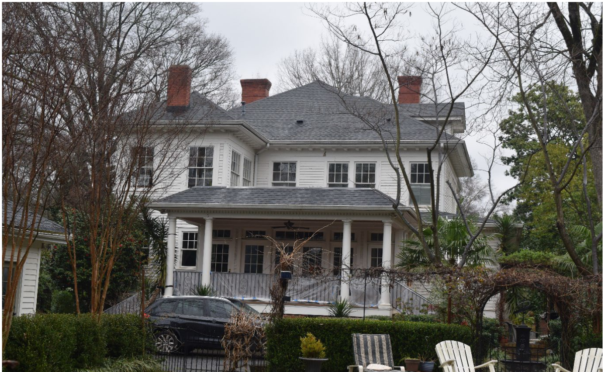
Rear of house (west elevation) after ca. 2015 renovation
