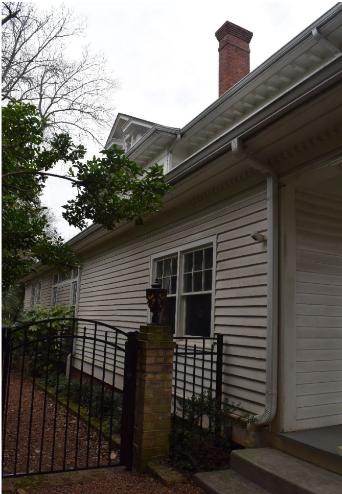
Southeast corner of house, view northwest.
