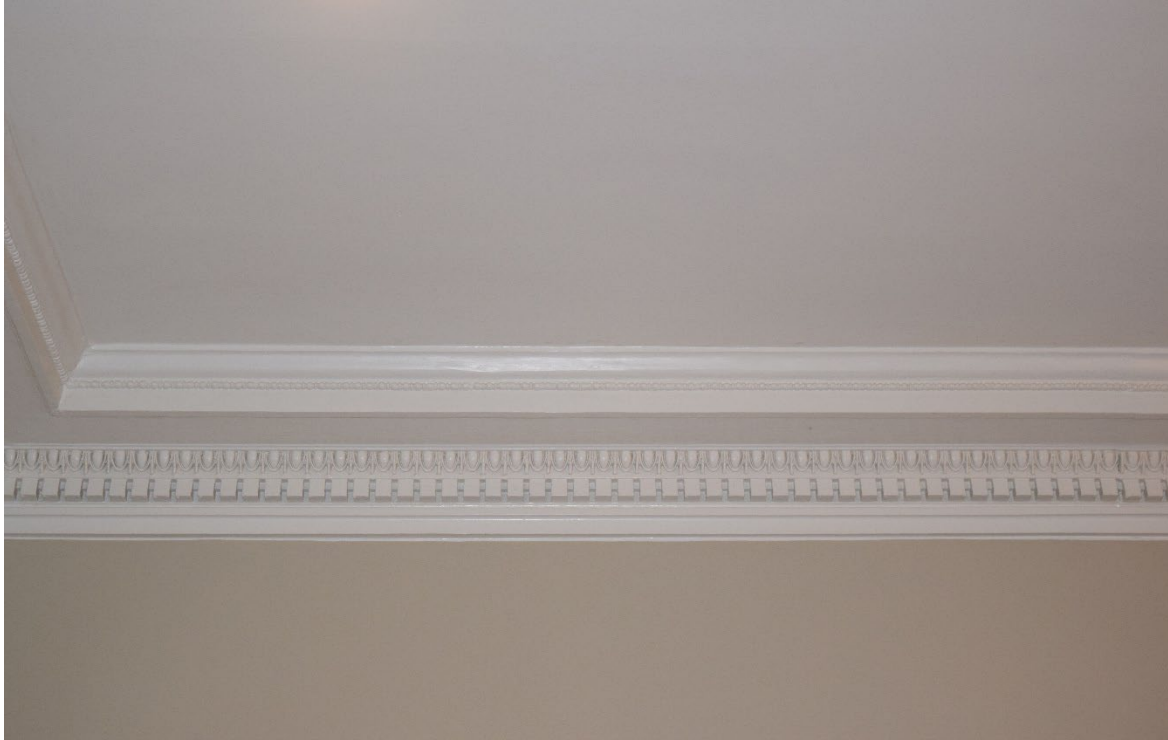
Crown molding throughout first floor
