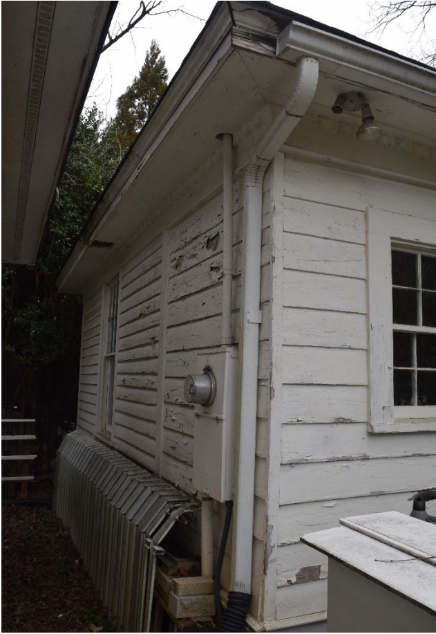
West elevation, servant's quarters/guest house, view northeast
