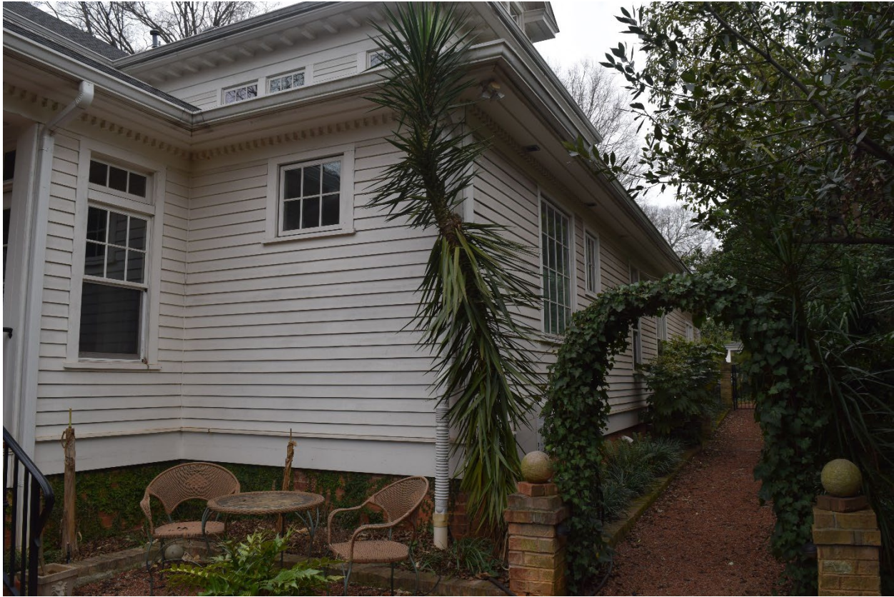
Southwest corner of house, view northeast.
