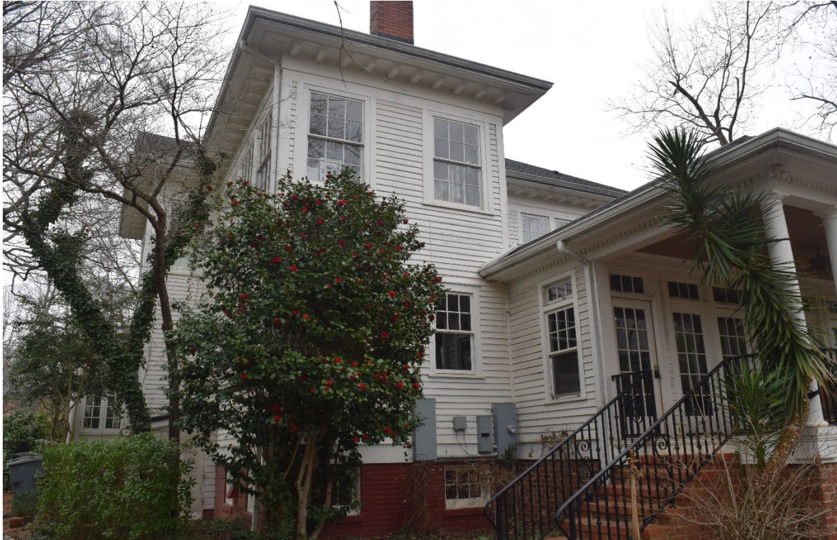
Northwest corner of house, view southeast.
