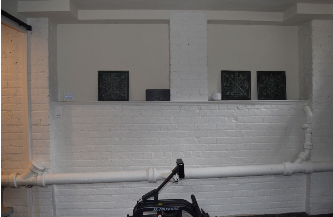
Painted brick, basement walls.
