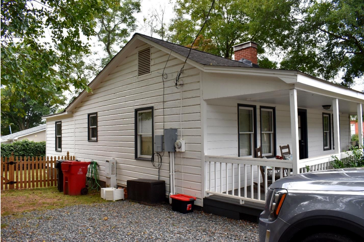
The east elevation of the Armour Street Mill House is similar to the west elevation at the first and second bays. However, the third bay has a shorter 1/1 vinyl window. The gabled addition at the rear is flush with this elevation and has a typical window centered in its face. Alongside this elevation is a narrow gravel parking area and wood picket fence.
