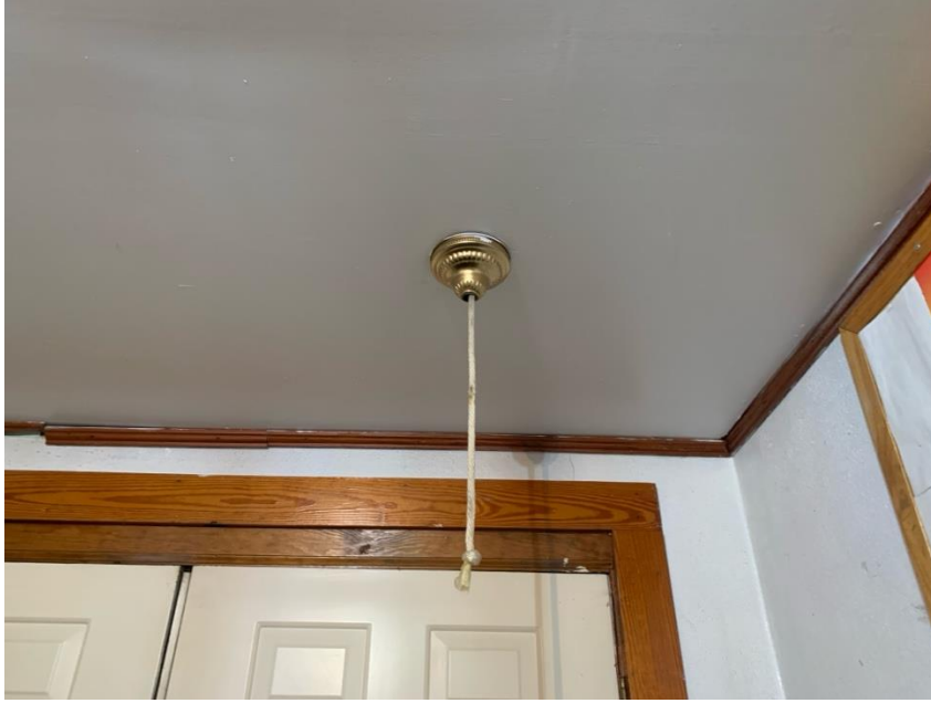
Rope pull for the original church bell housed in the 1909 steeple.
