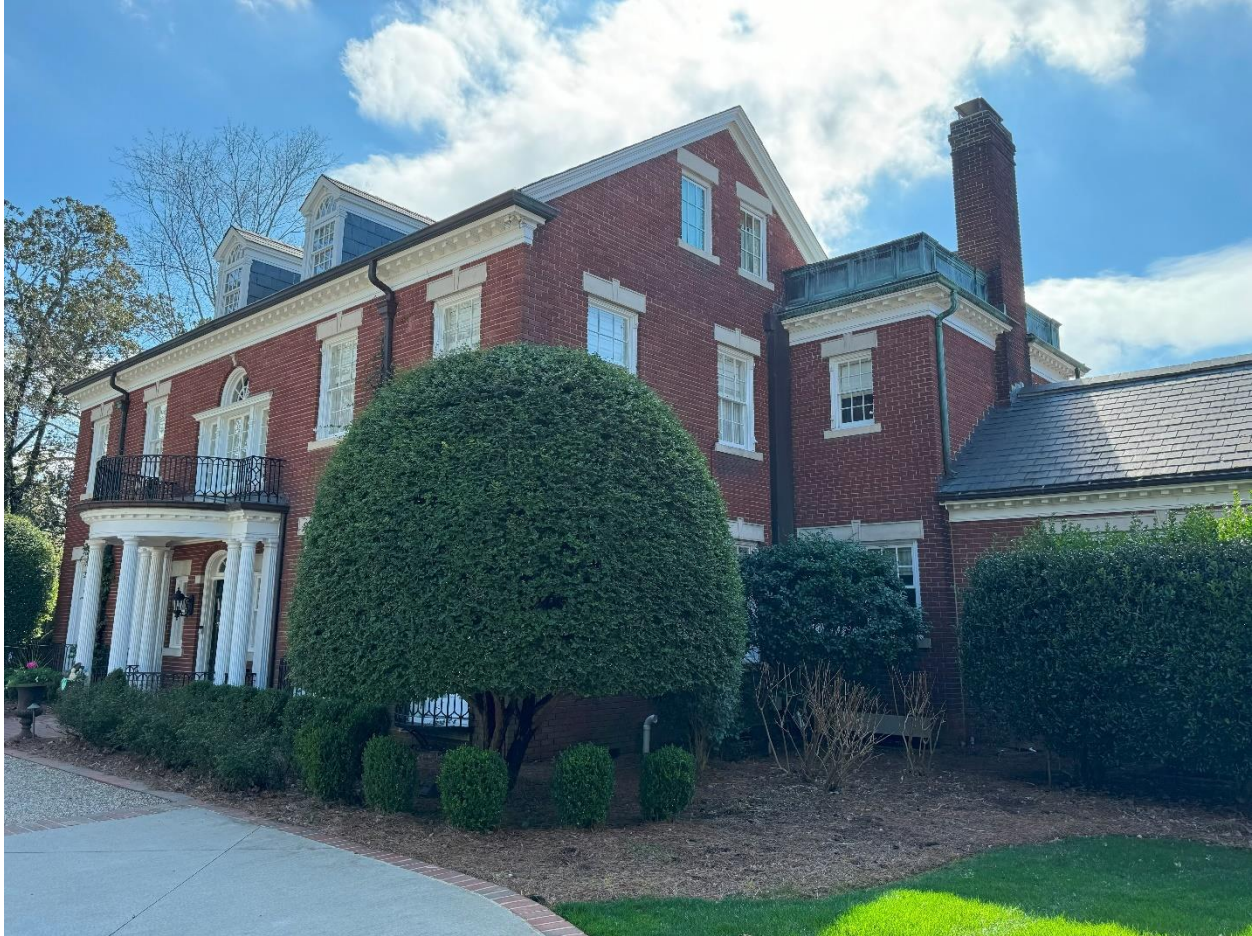
Figure 17 North Elevation looking southwest
