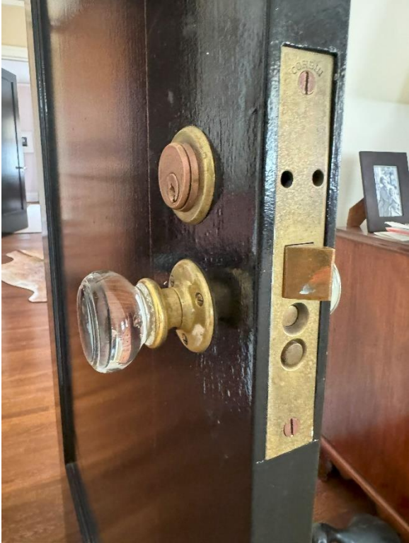
Typical original glass knob and door hardware
