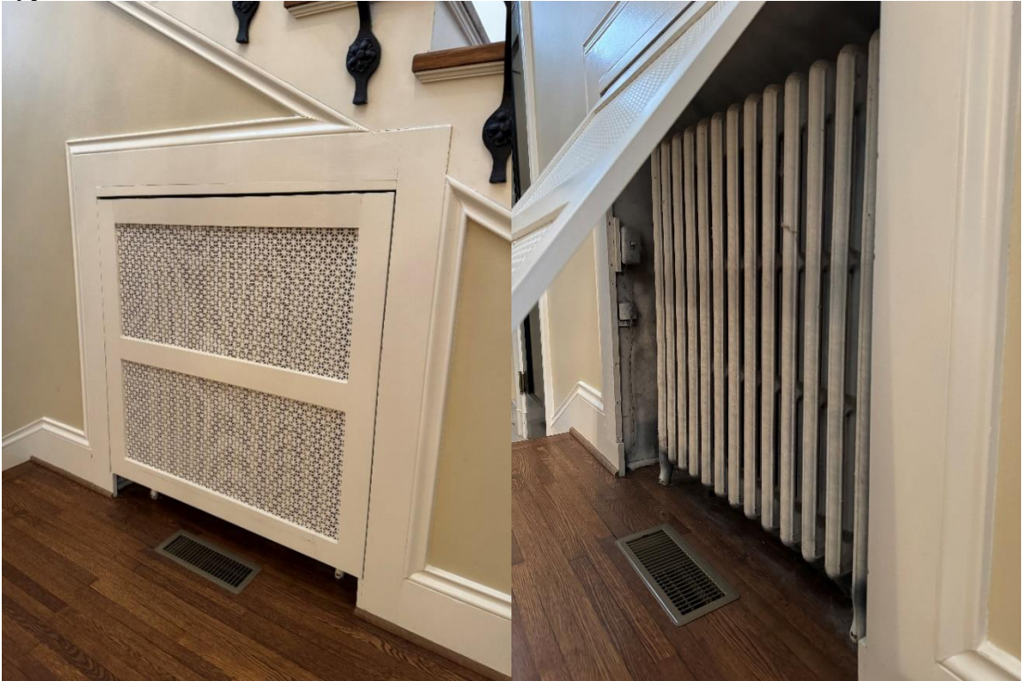
Typical radiator and cabinet
