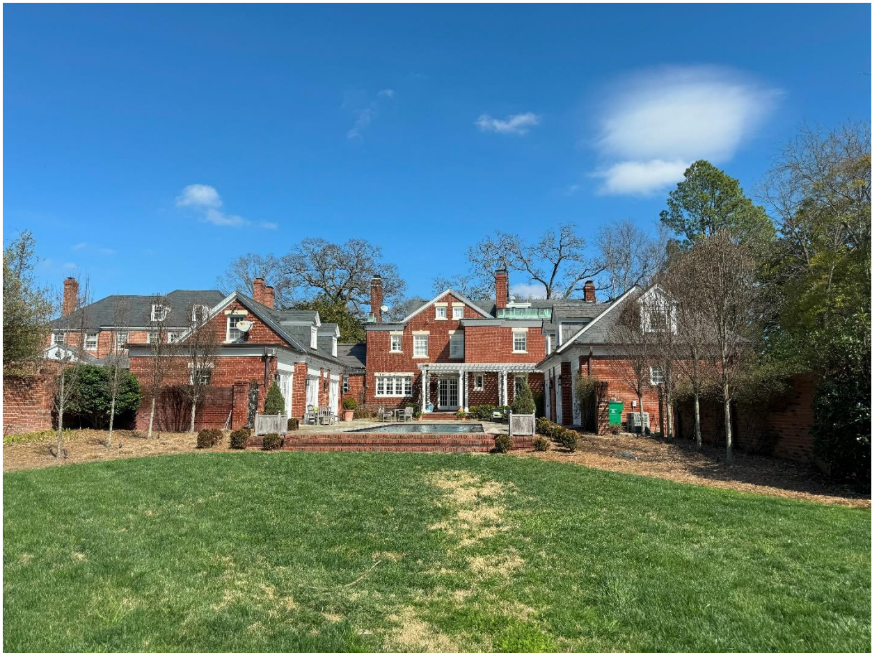
Figure 18 West Elevation looking east from rear of property
