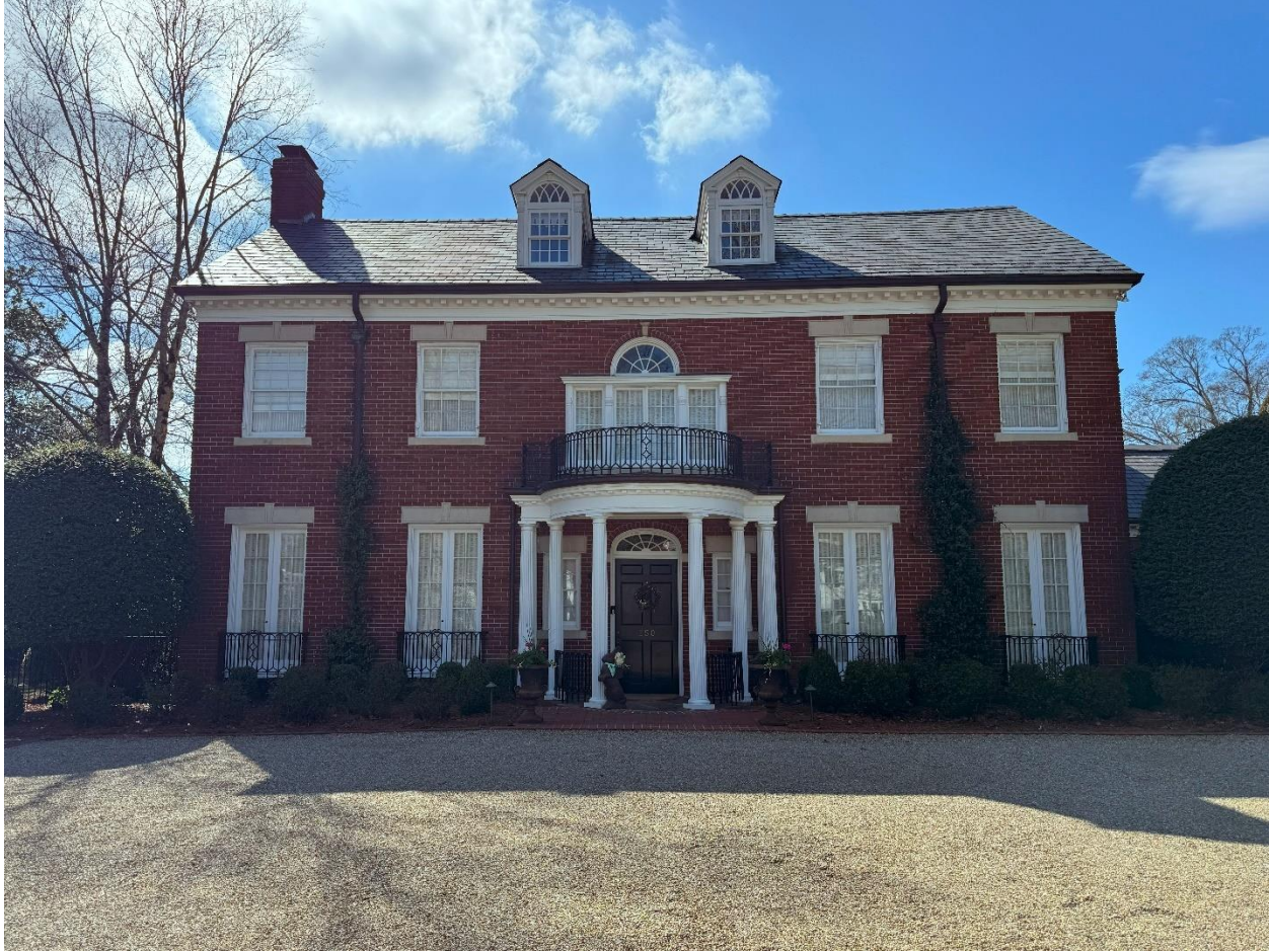
Figure 15 Façade/East Elevation looking west
