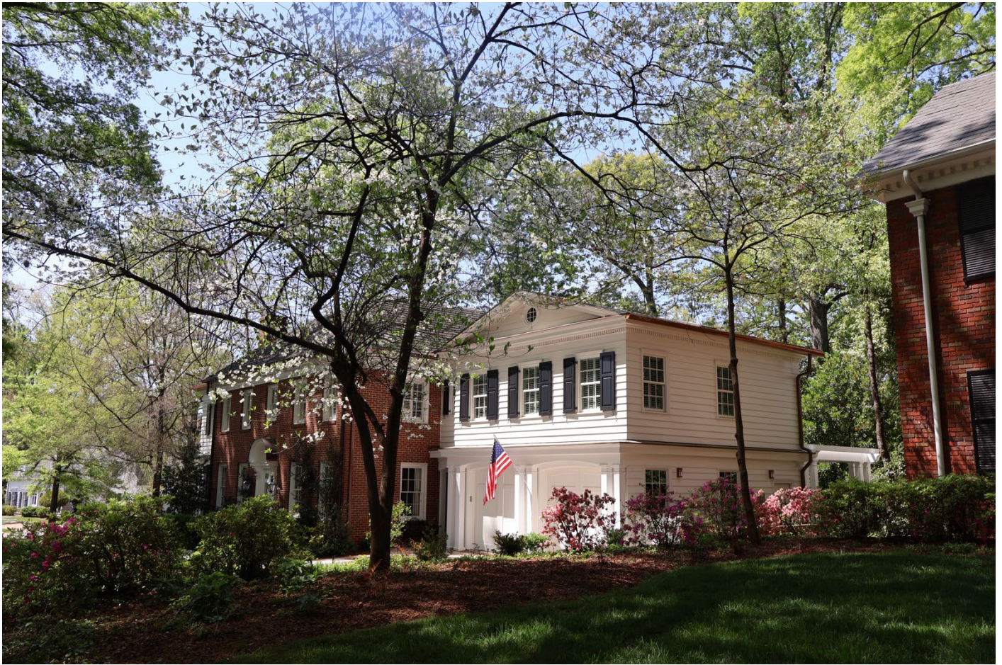
Photo 5: Side (North) Elevation
