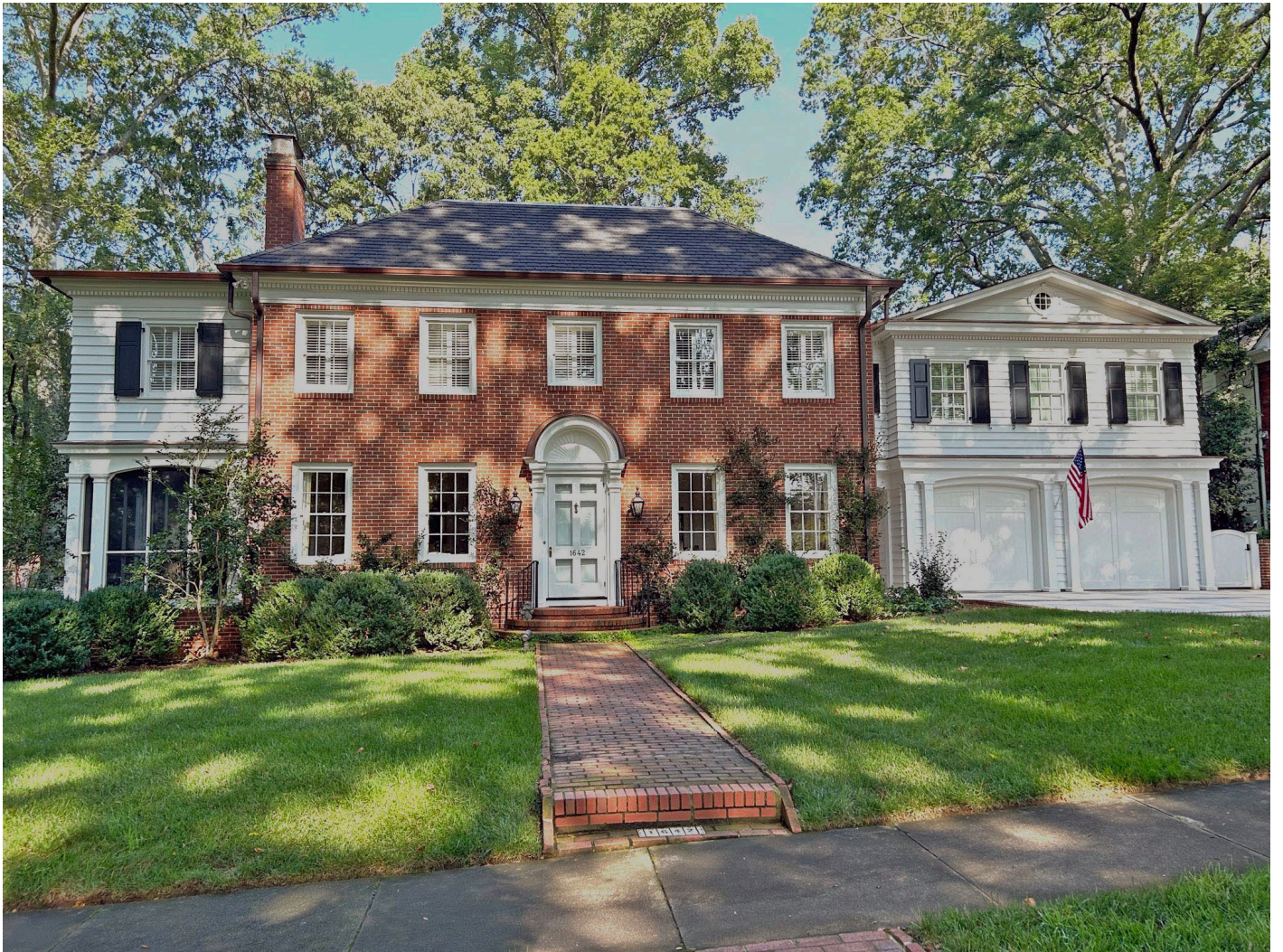
Photo 2: Front (East) Elevation
