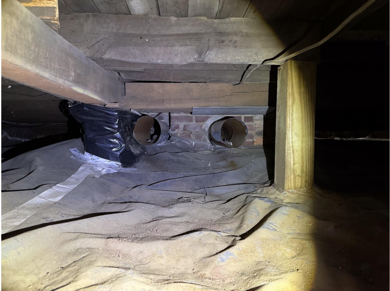
Figure 12 View at the crawlspace looking north toward the brick chimney. The wood plank subfloor at the top of the photo runs perpendicular to the floor beams, identifying this portion of the Caldwell-Bradford School as the original portion.
