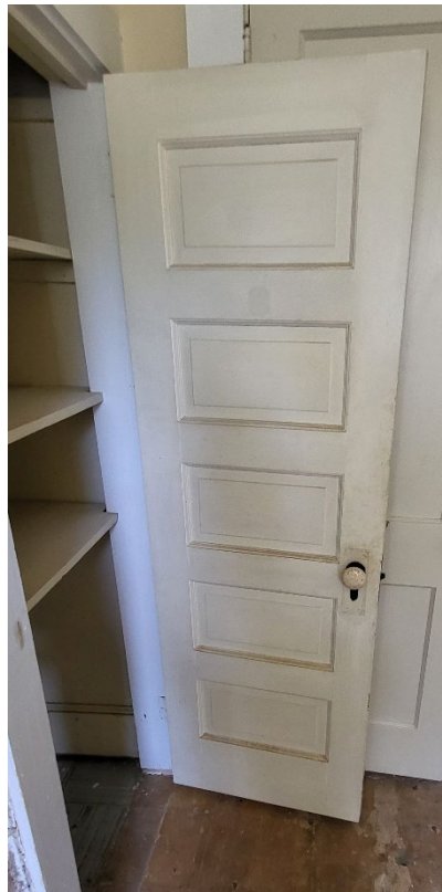
Primary Suite, right closet on north wall (above). Note original five-panel door with original hardware. Second floor bathroom, entrance (below, left) and closet (below, right) doors.
