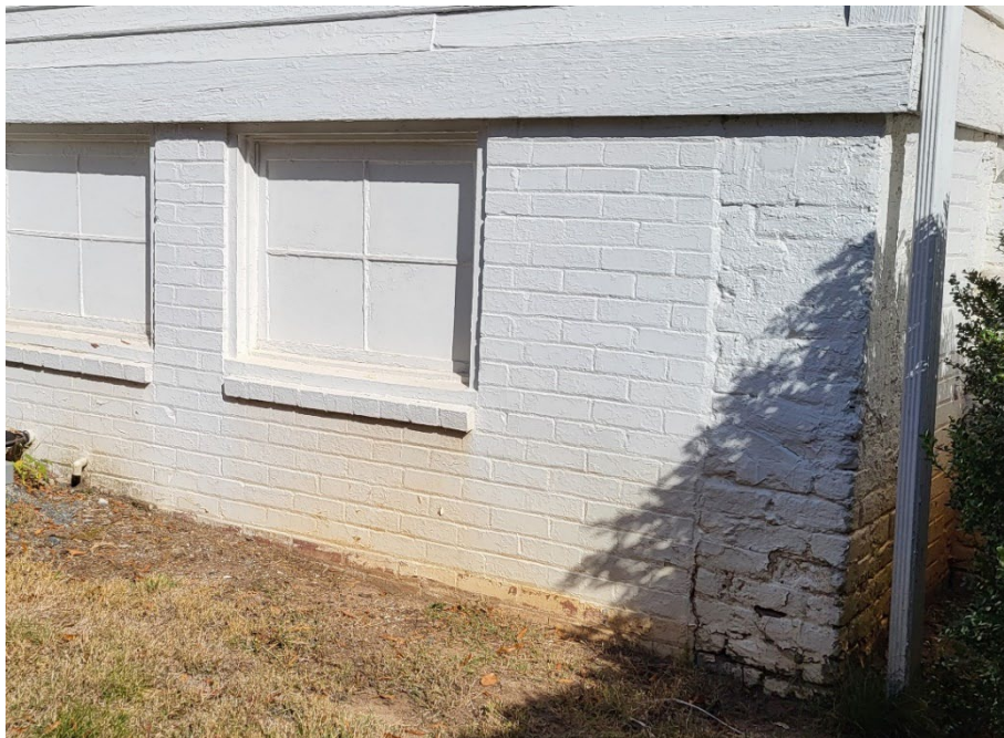
South elevation foundation.
