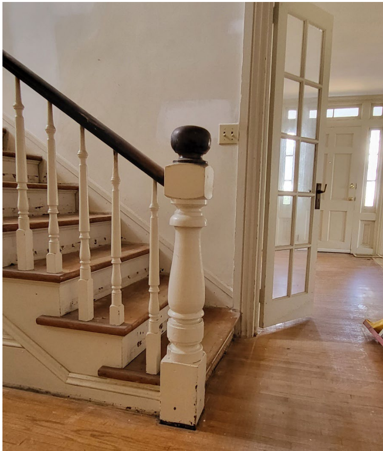
Detail of acorn-shaped pendell and molding in first floor stair hall (above) and detail of balustrade and newel (below). The glass paned door in the image below leads to the living room. The six panel wooden door in the background is the main entrance.
