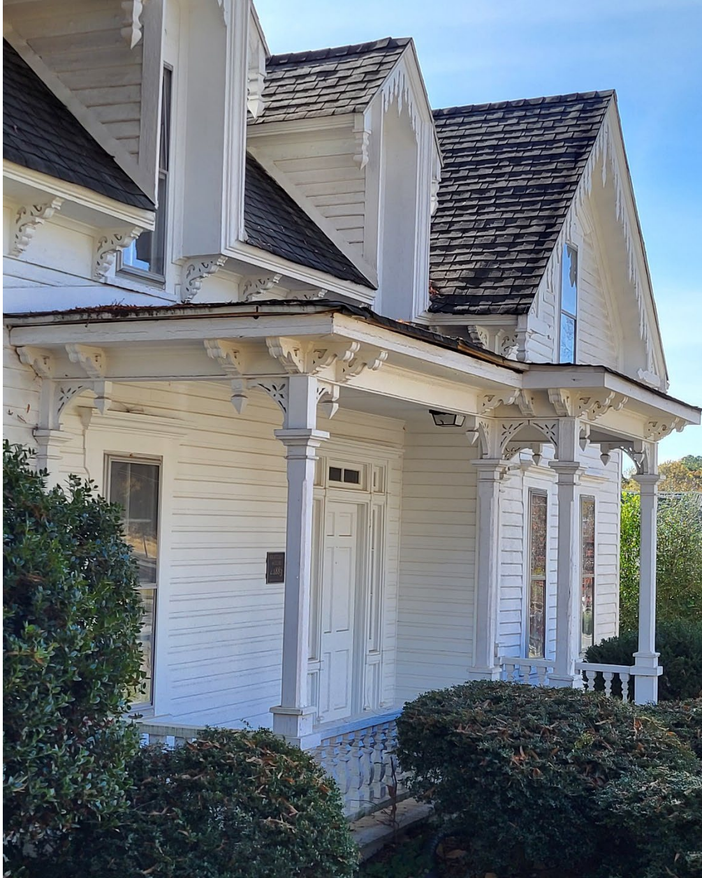
Front porch and main entrance.
