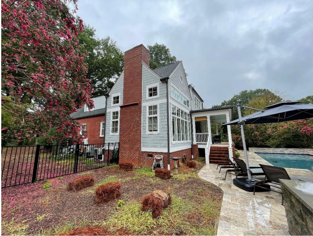
Figure 7 West and South Elevations looking Northeast
