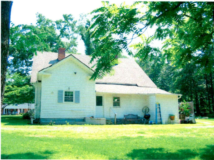
Plate 4. Rogers House, Rear (North) Elevation, Looking South.
