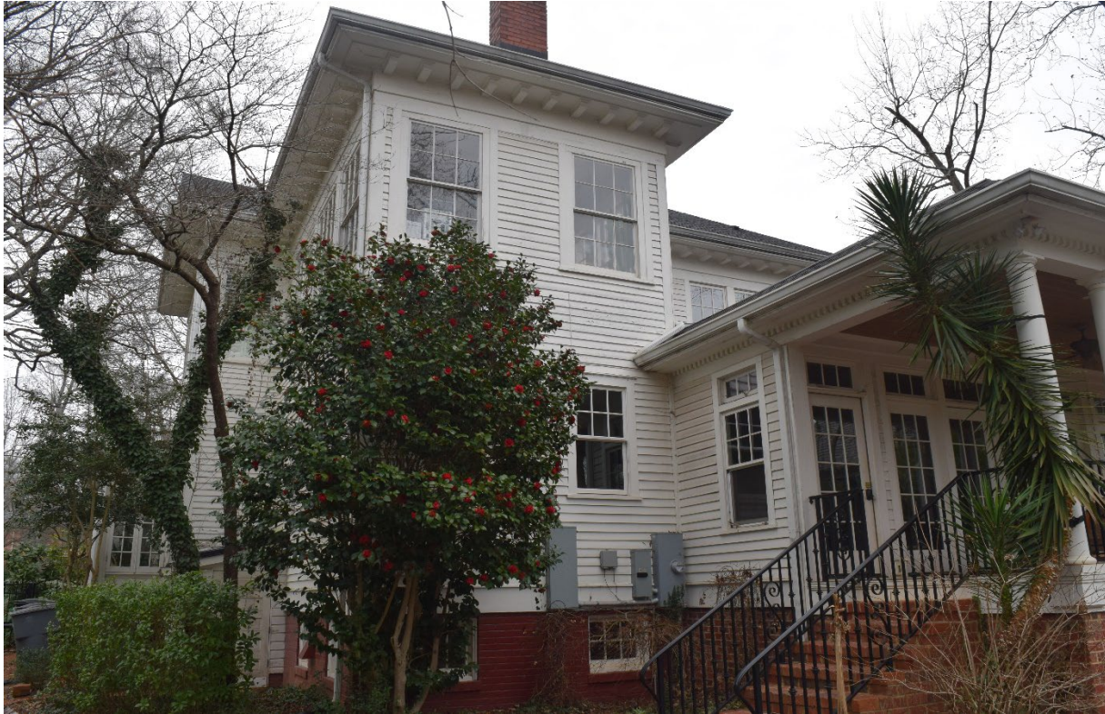
Northwest corner of house, view southeast.
