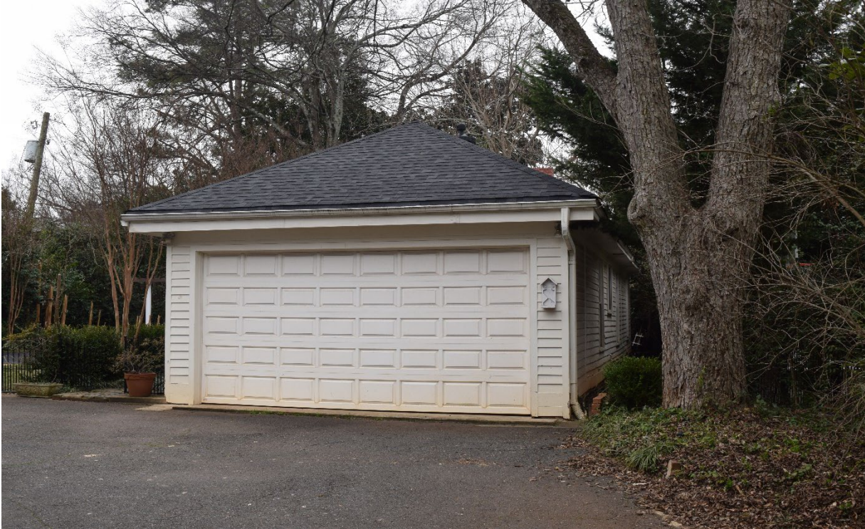
East elevation, servant's quarters/guest house, view west.
