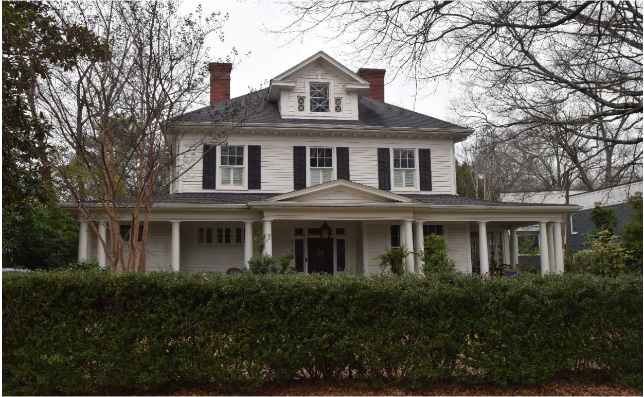
Front of house (east elevation), view west
