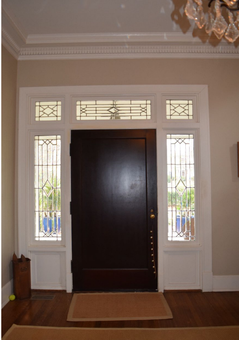
Front door detail, view east
