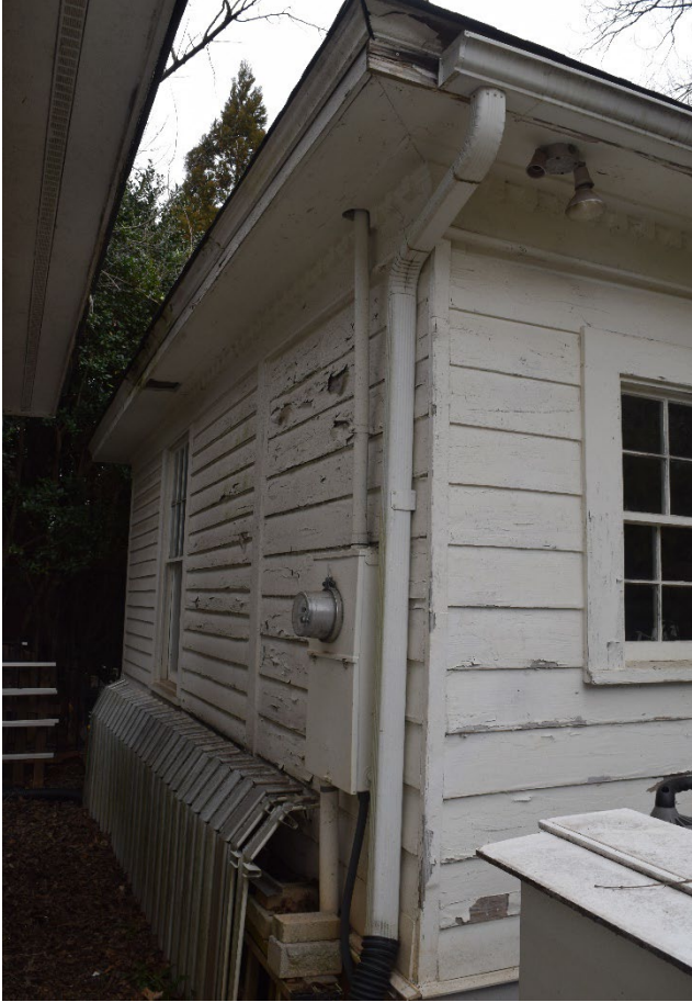
West elevation, servant's quarters/guest house, view northeast
