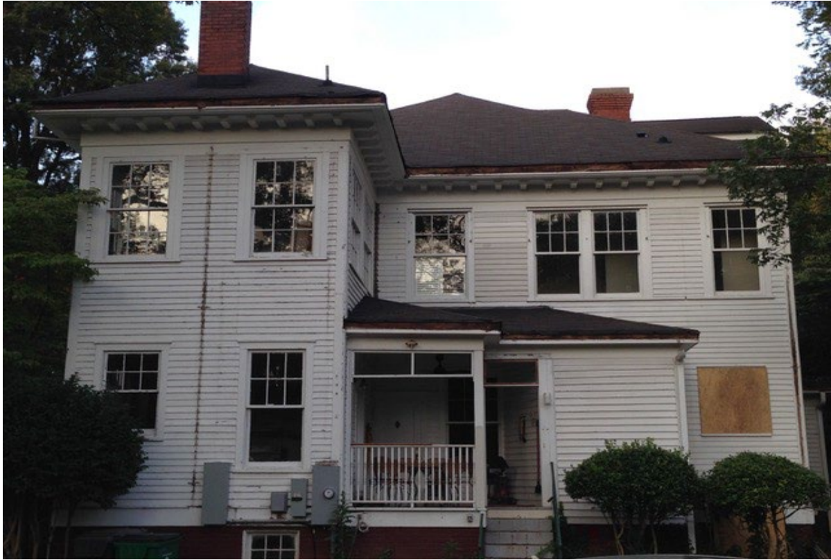
Rear of house (west elevation) before ca. 2015 renovation
