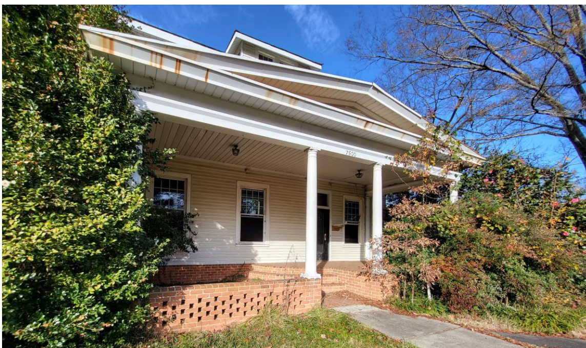
Front elevation detail showing split-level brick porch and semicircular stair.
