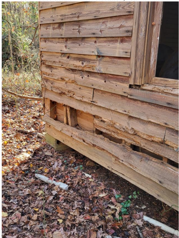
Back House detail – west elevation
