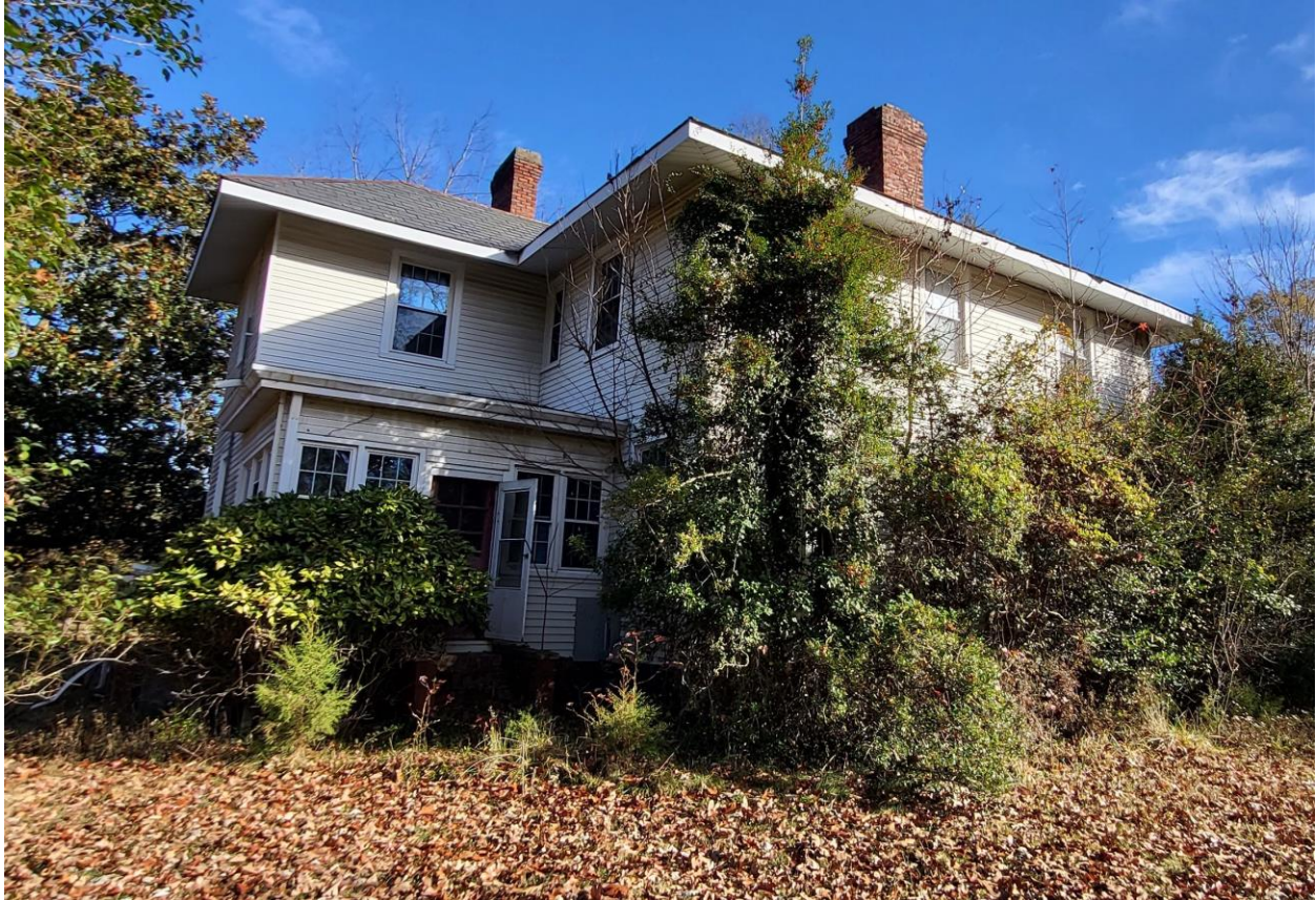
South and rear elevations.
