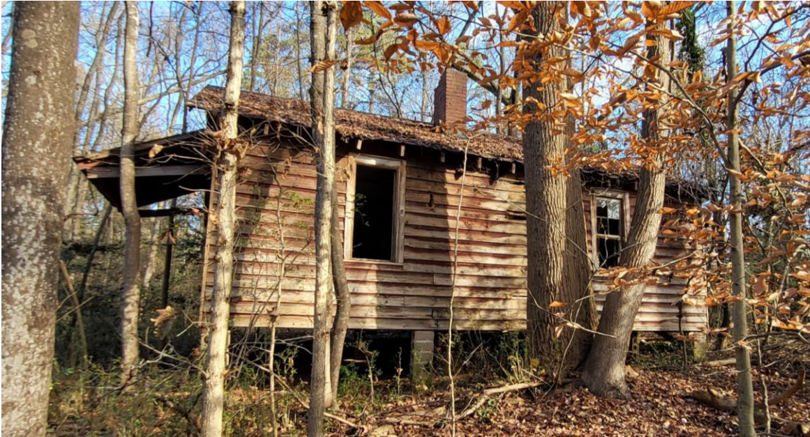
Back House east elevation.
