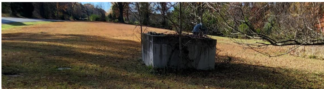
CMU block water feature located at front property line.
