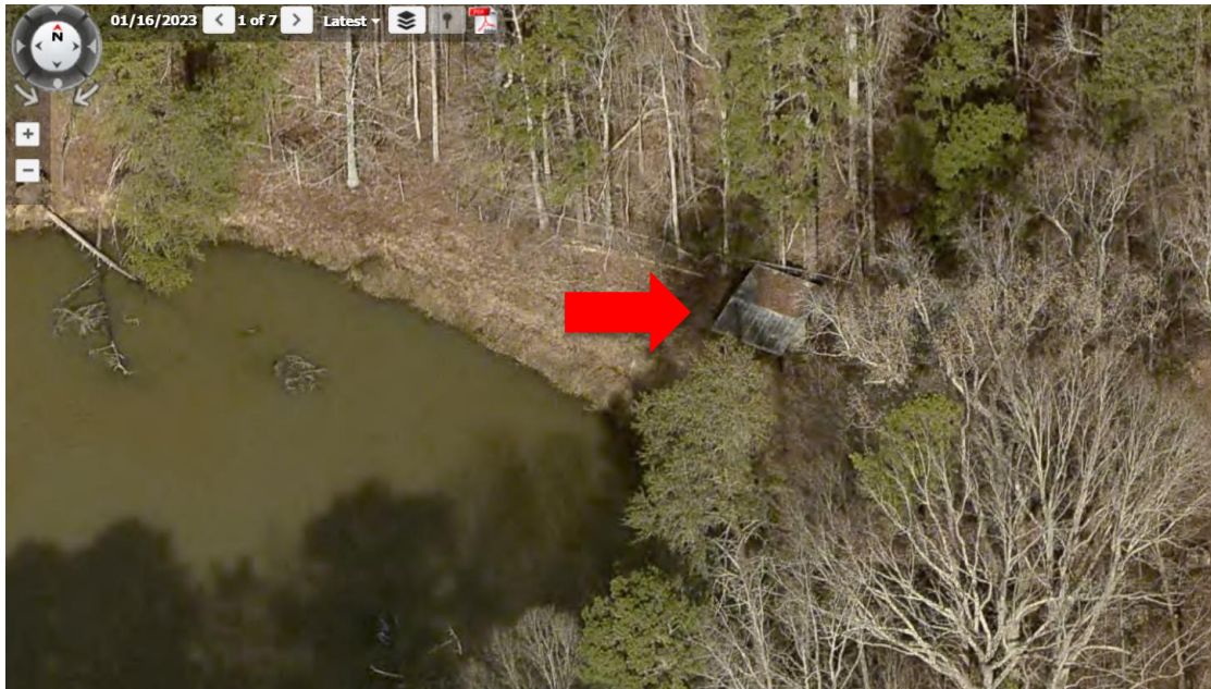
Shoaf Lake Structure
