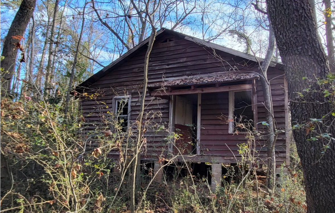
Back House rear elevation.
