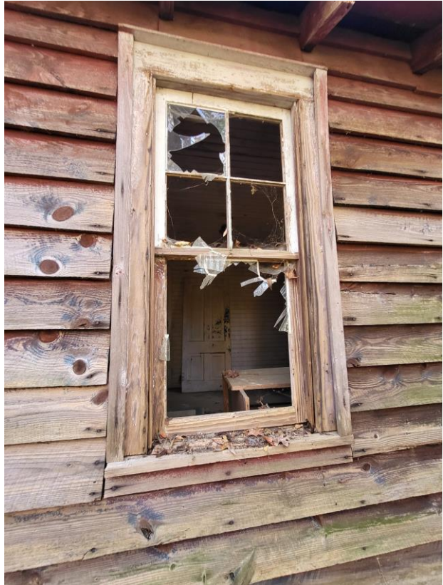
Back House detail – west elevation, rear window.
