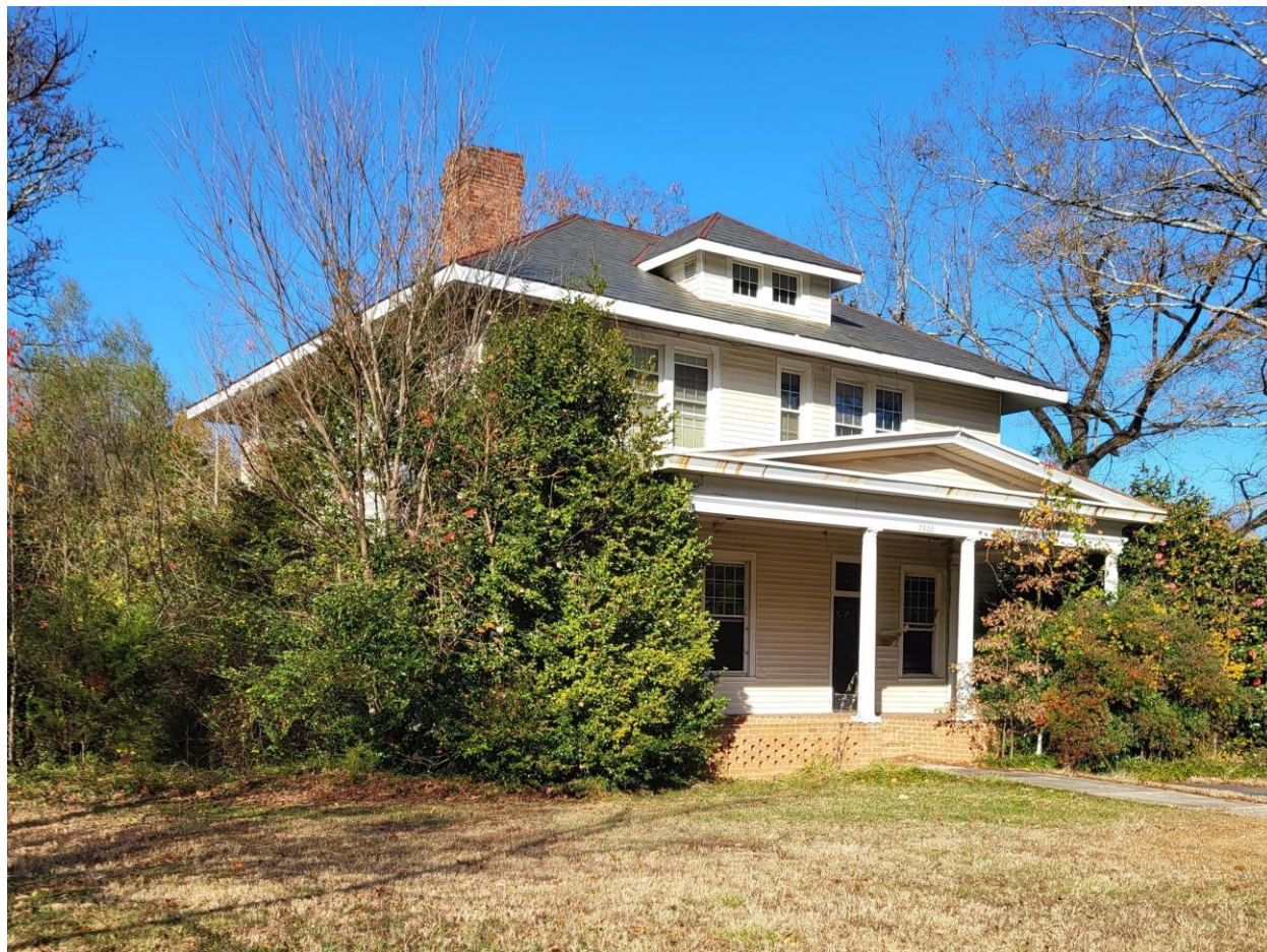
Front elevation, looking northwest.
