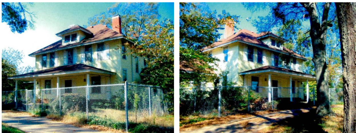
The now-demolished Dr. Richard Z. Query House (1919). Note the hipped dormer and second story window grouping on the front elevation and the contrasting symmetrical and irregular fenestration on the side elevations, reminiscent of the Steele Creek manse constructed earlier by the same builder. Source: Mattson, Alexander and Associates, Inc., "Architectural Resources Survey Report, Wallace Neel Road Relocation, Charlotte, Mecklenburg County," July 7, 2004, 15, accessed December 5, 2023, https://files.nc.gov/ncdcr/historic-preservation-office/PDFs/CH_04-0636.pdf .
