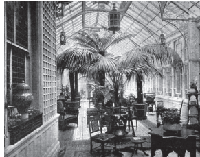
SANDRINGHAM HOUSE BUILT : 1884
