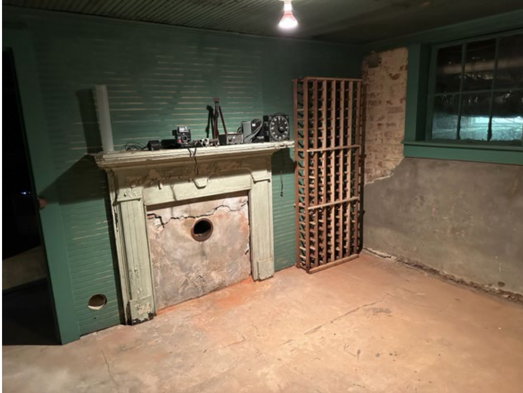
Above: Northwest basement room with original brick wall, fireplace, and mantel.
