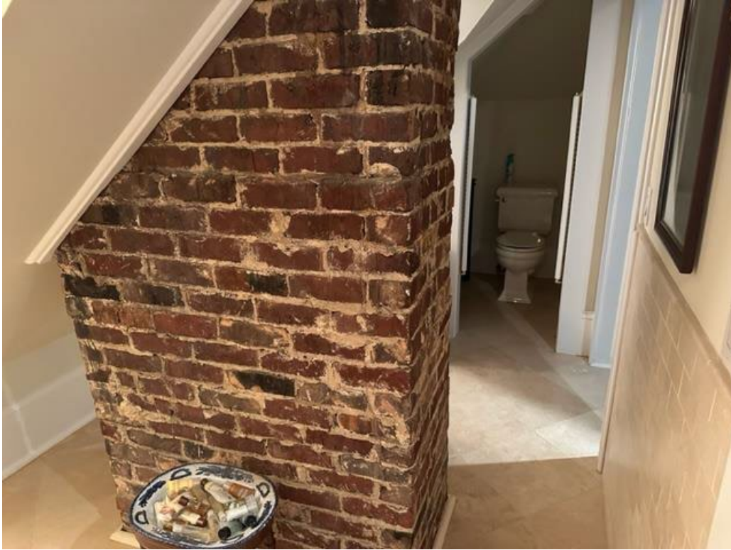
Above: Third Floor bathroom under eaves facing South.
