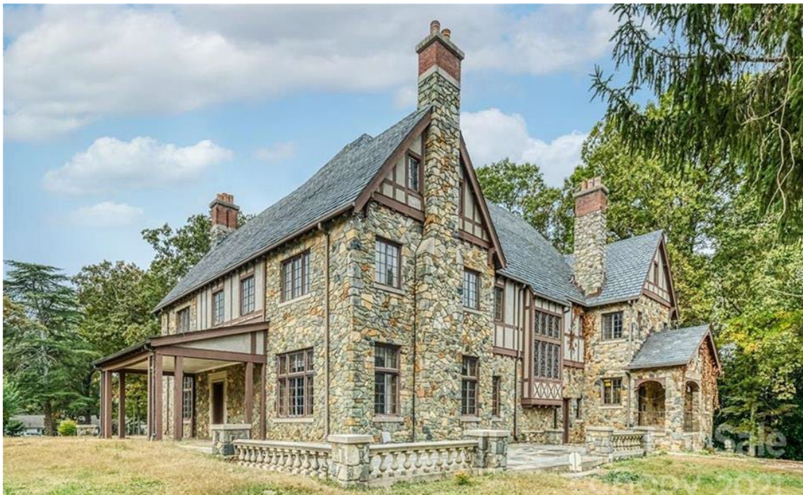
Akers House, right and rear elevations.
