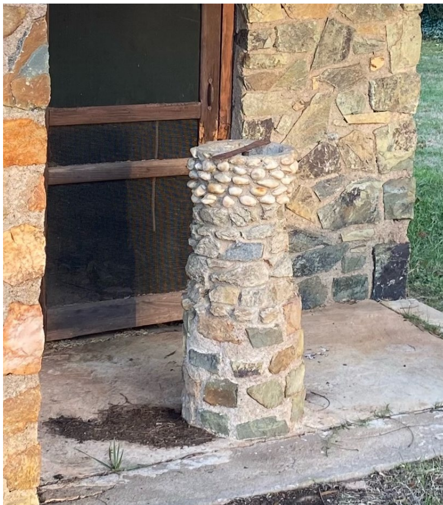
Detail of water fountain at front elevation of Akers Acre well house. Source: Roger Ball.
