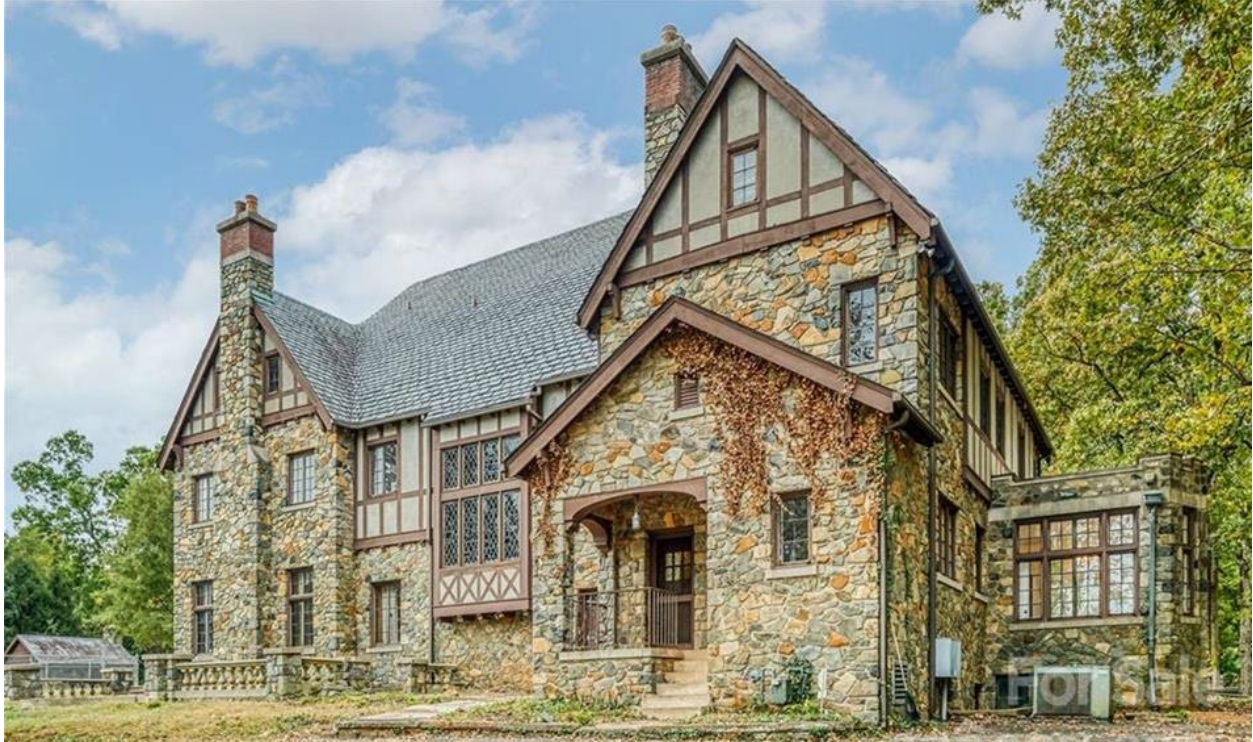
Akers House, rear and left elevations.
