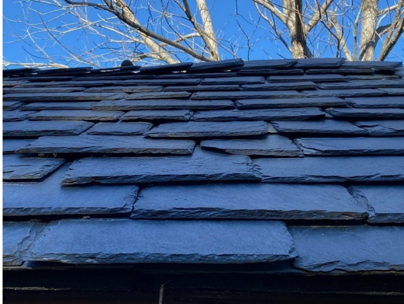
Slate roof of Summer House at Akers Acres. Source: Roger Ball.
