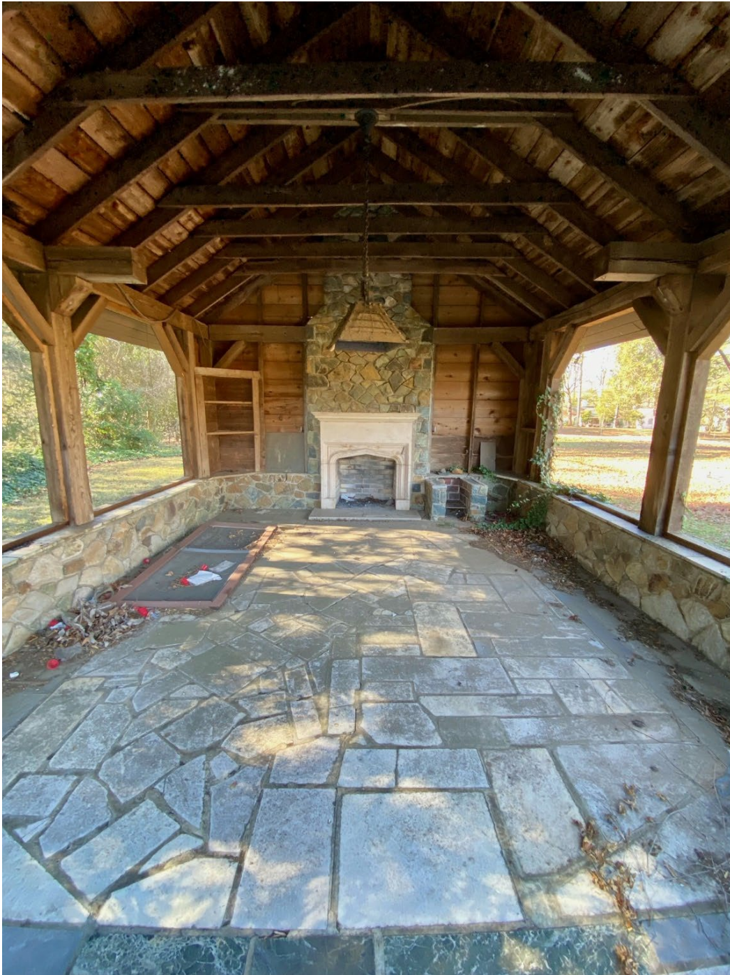
Interior view of Summer House at Akers Acres. Source: Roger Ball.
