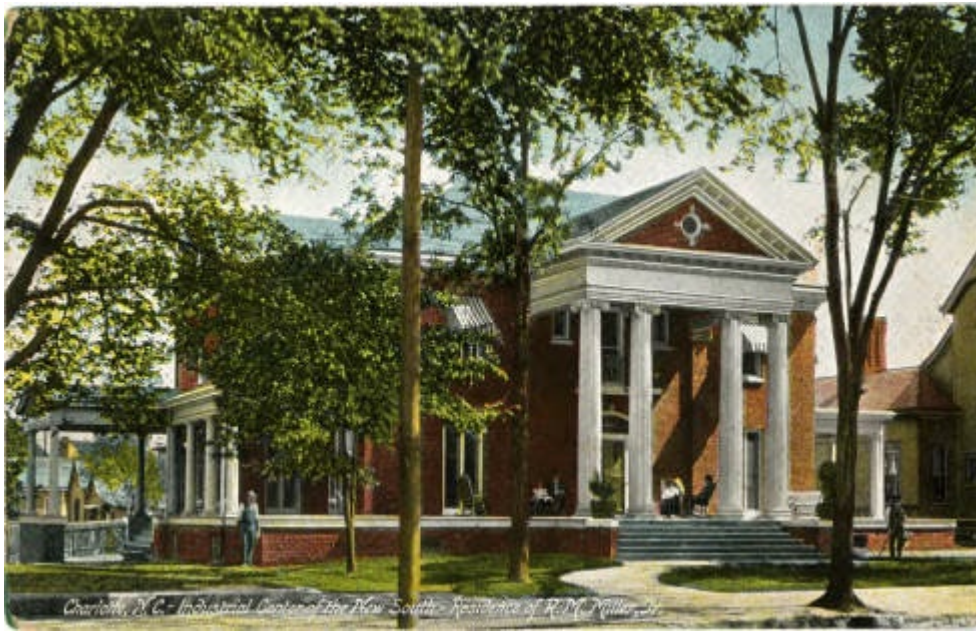
R. M. Miller, Jr. House (no longer standing)
