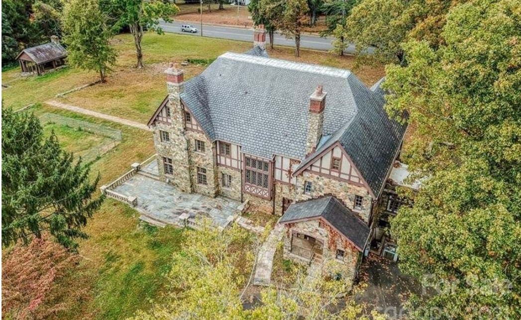
Akers House, aerial view of rear elevation.
