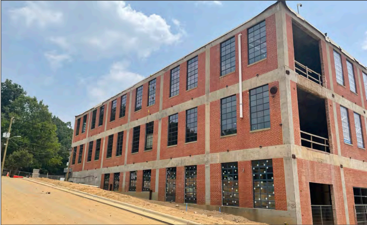
6. North facade of Paper Warehouse, looking SE
