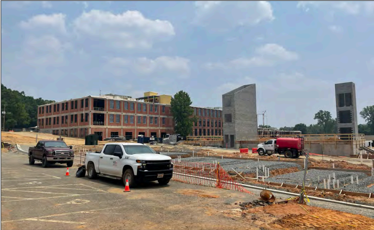
3. Overall site view, looking SE
