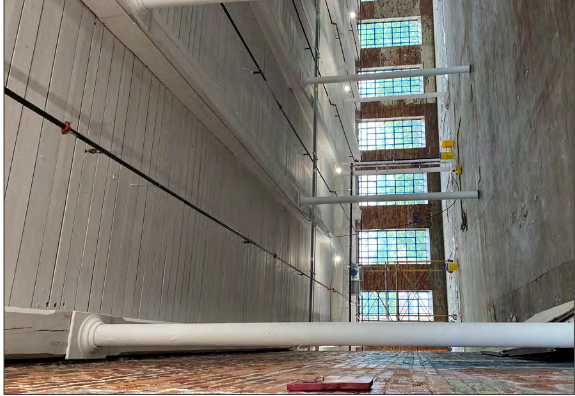
25. Spinning Mill, second floor, looking E along interior wall
