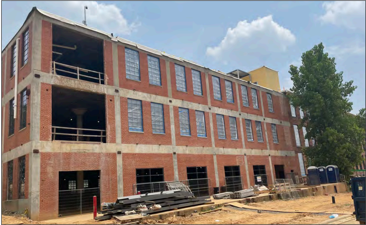
7. West facade of Paper Warehouse, looking E
