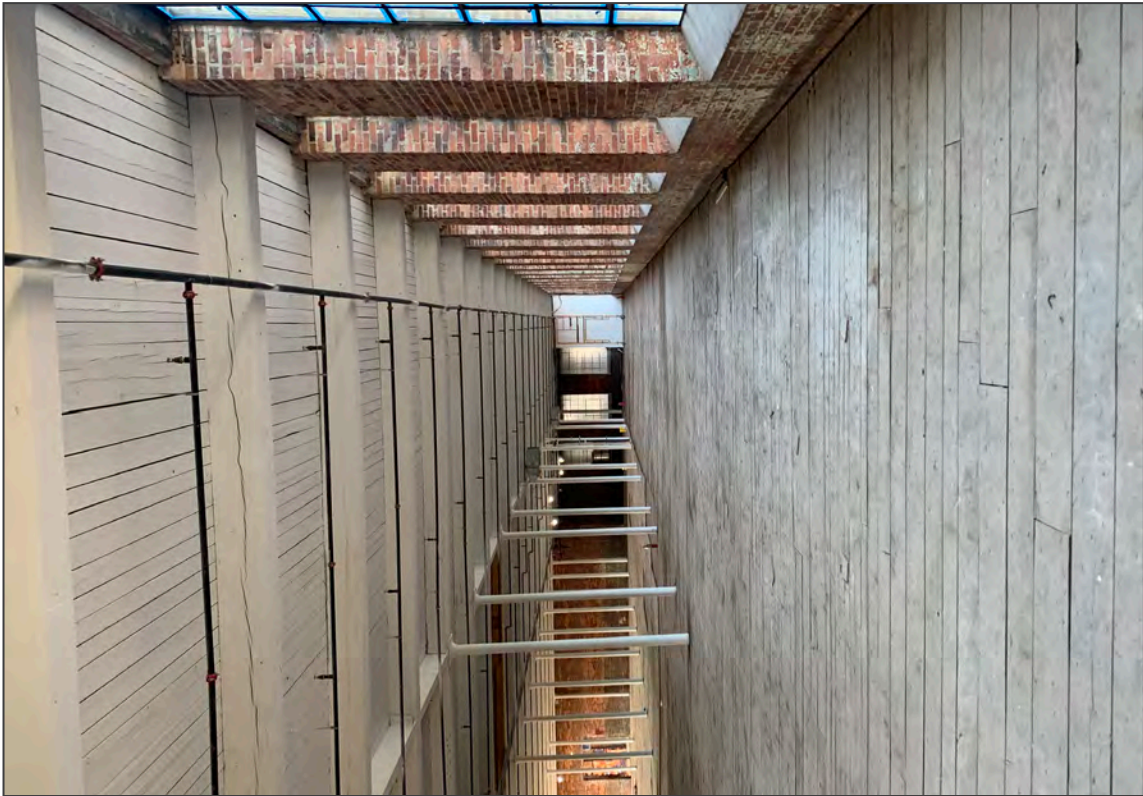
21. Spinning Mill, second floor, looking N along E wall
