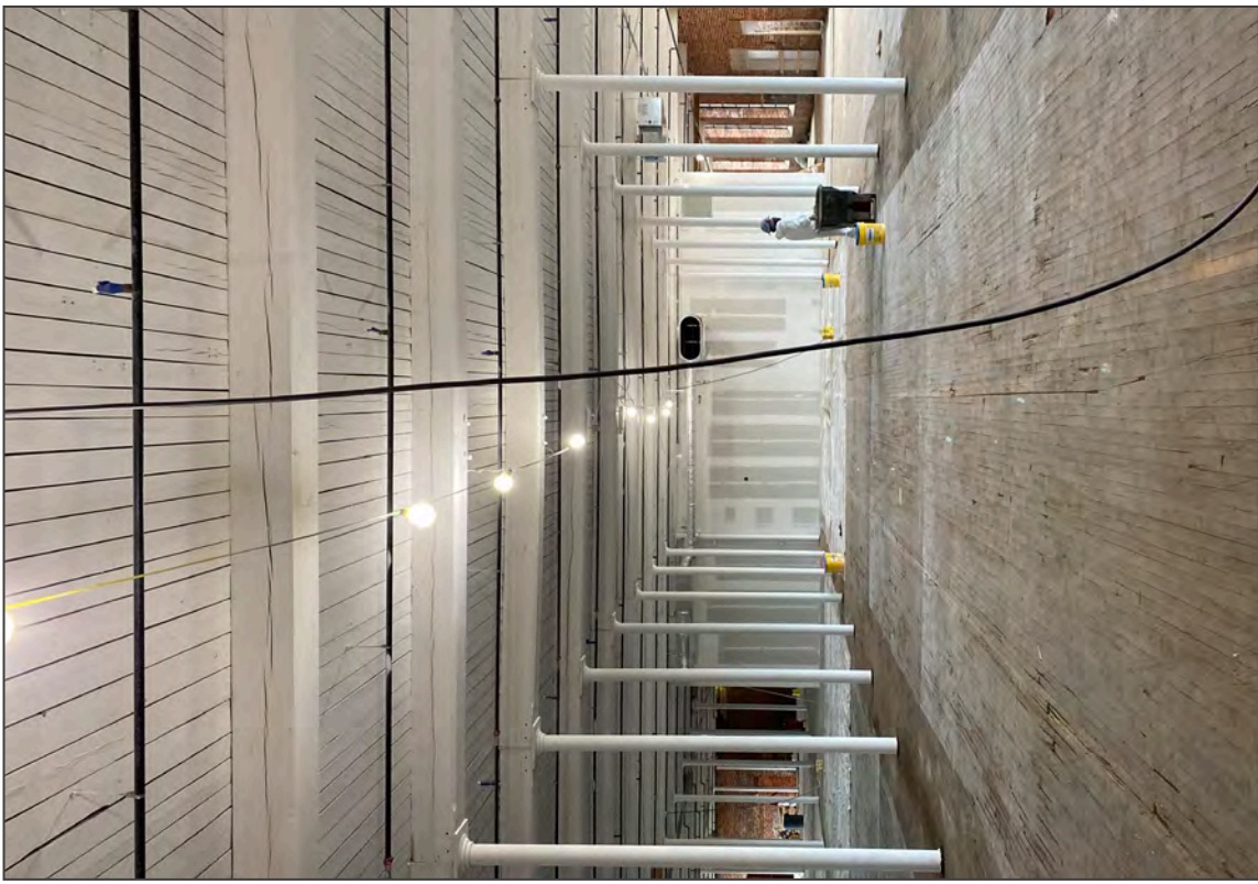
22. Spinning Mill, second floor, looking S
