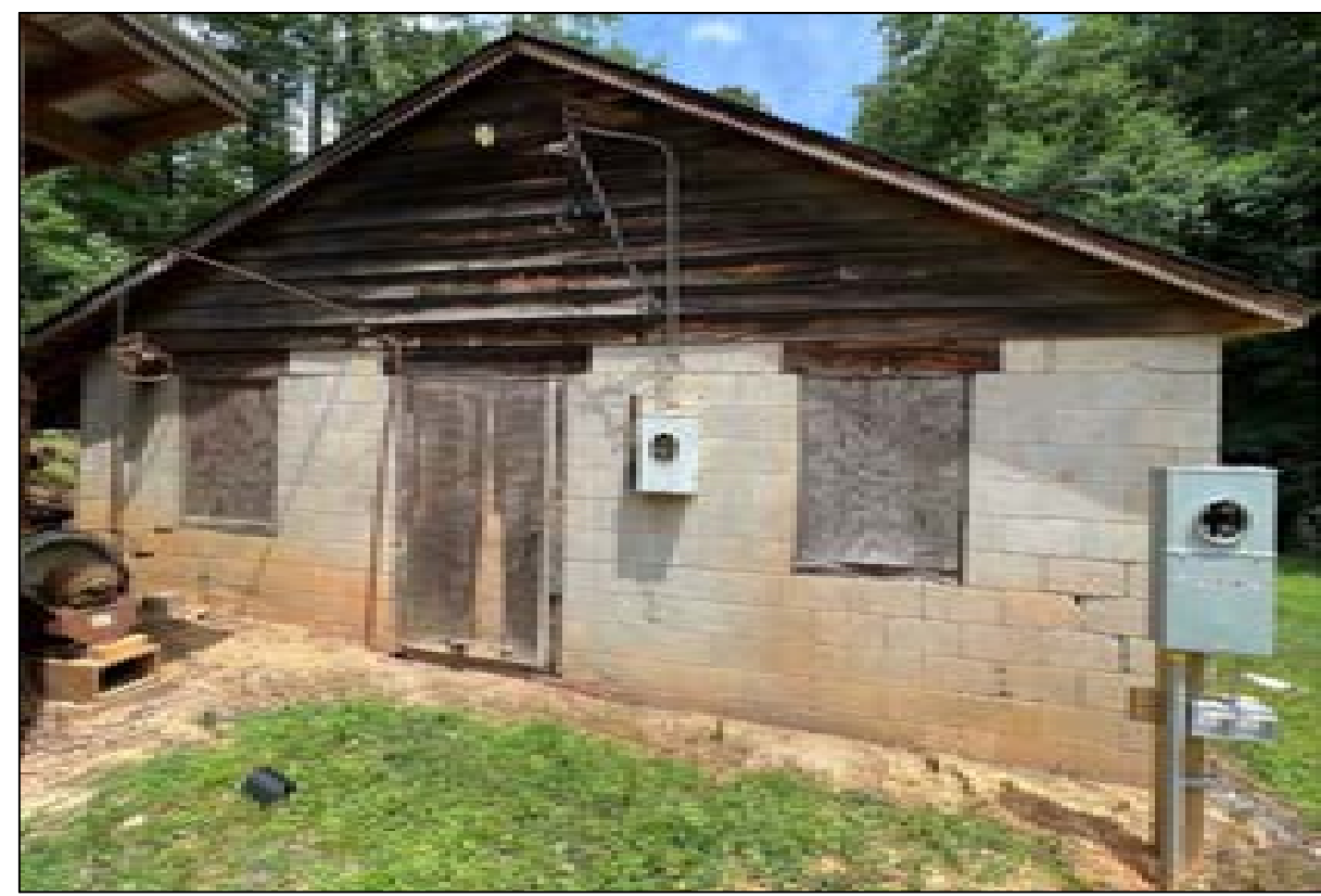
SOUTH ELEVATION - OVERVIEW
