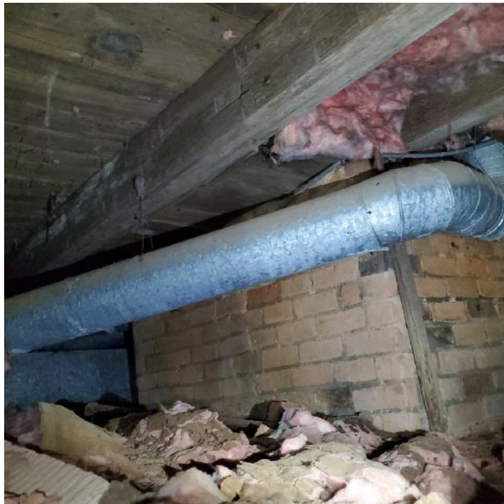
Photograph 58: View of floor framing at interior chimney.
