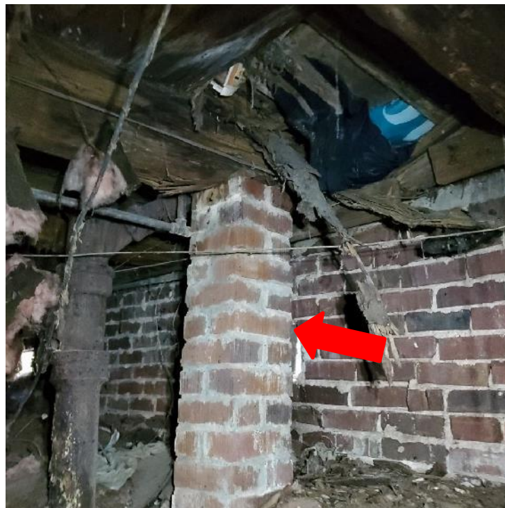
Photograph 56: View of brick masonry pier in crawlspace (arrow).
