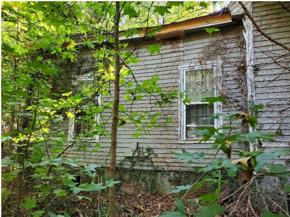
Photograph 6: Partial view of west elevation.
