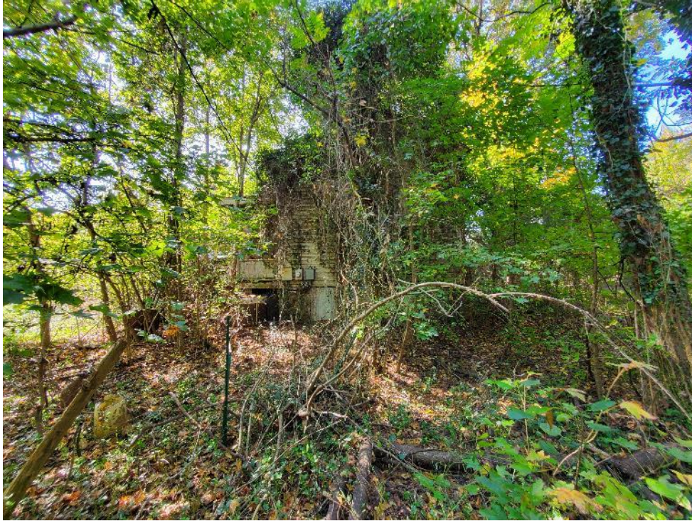
Photograph 7: View of north elevation.
