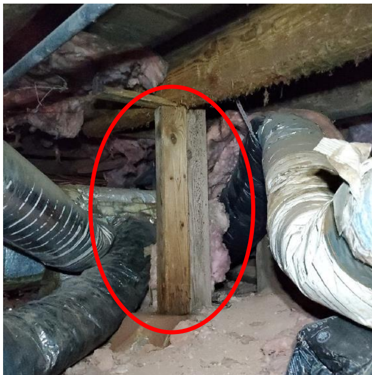
Photograph 62: Representative view of wooden post to ground (oval).
