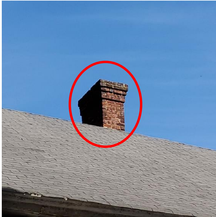
Photograph 23: View of chimney above roof level (oval).
