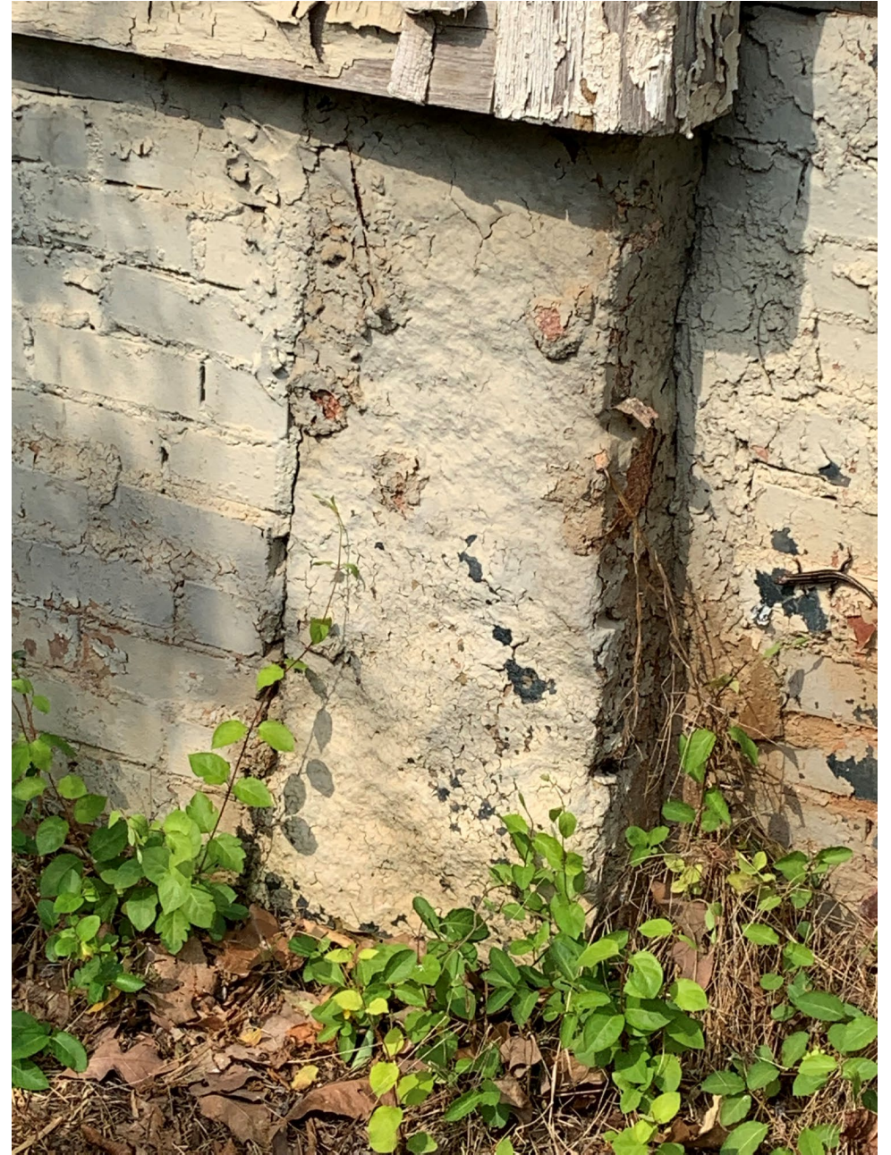
Stone pier and brick curtain walls
