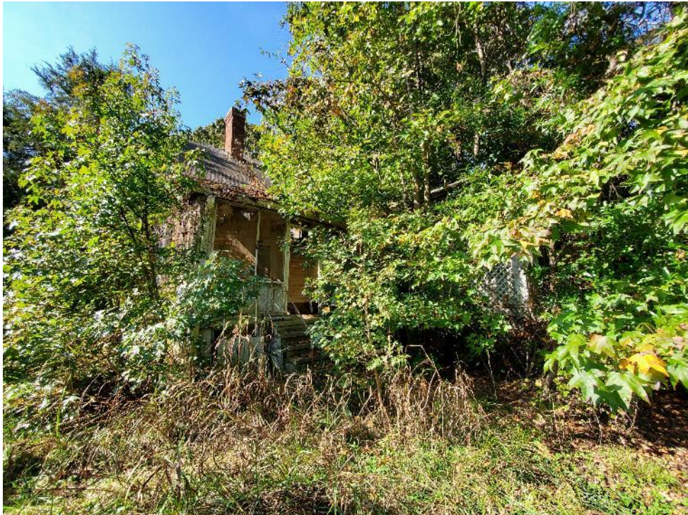
Photograph 8: Partial view of north and east elevation from the northeast direction.
