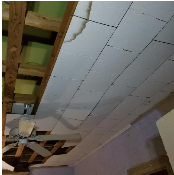
Photograph 44: Representative view of ceiling below original ceiling.
