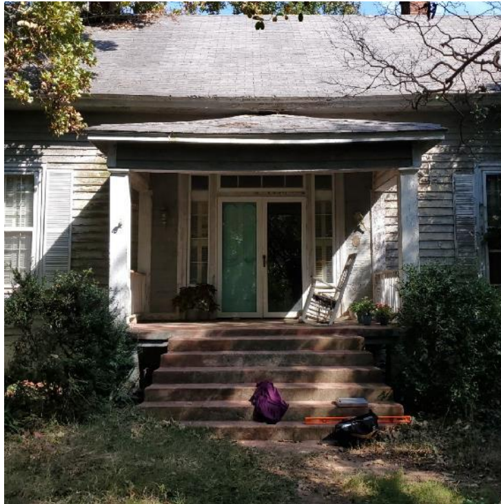
Photograph 15: Representative view of front porch.
