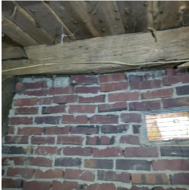
Photograph 57: View of front porch bearing along infill brick masonry wall.
