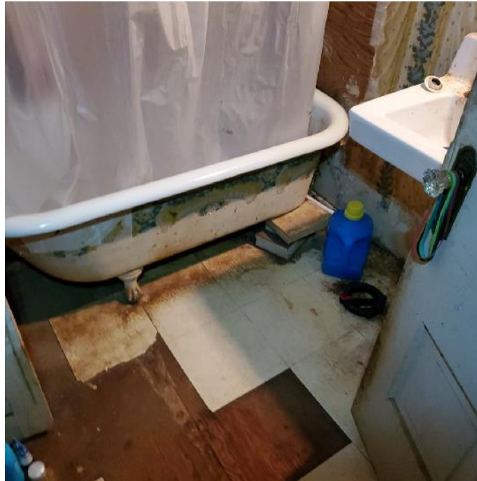
Photograph 45: Representative view of bathroom addition at corner of L-shaped porch.
