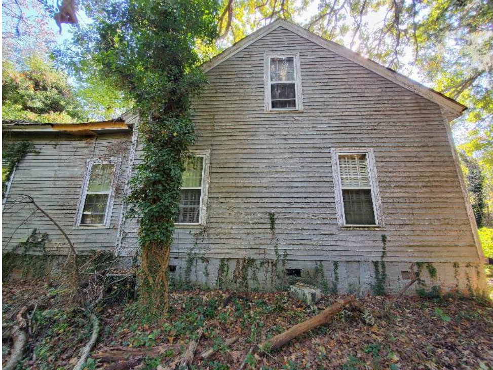
Photograph 5: Partial view of west elevation.
