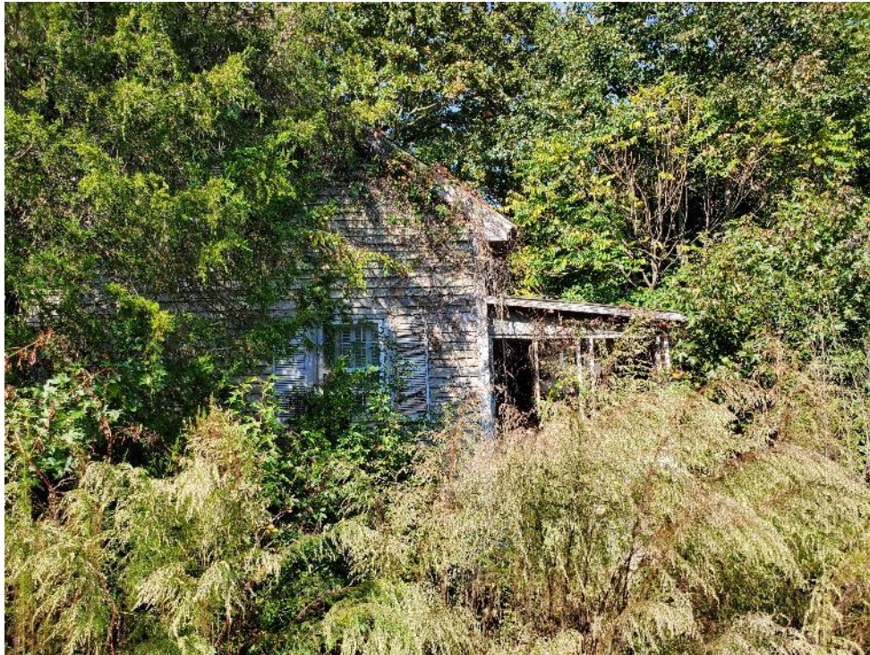
Photograph 9: View of east elevation.
