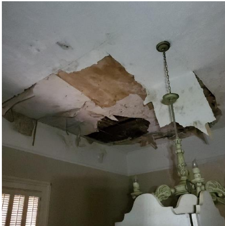
Photograph 42: View of water related damage to the ceiling at the southwest corner.
