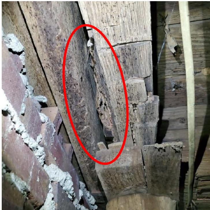
Photograph 70: View of insect related damage (oval).
