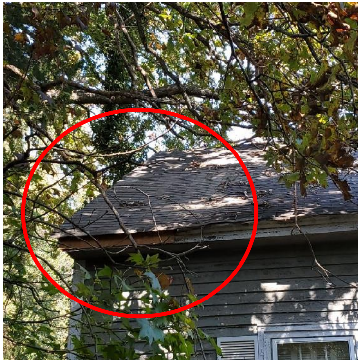
Photograph 22: View of different color shingles and replaced fascia at southwest corner (oval).
