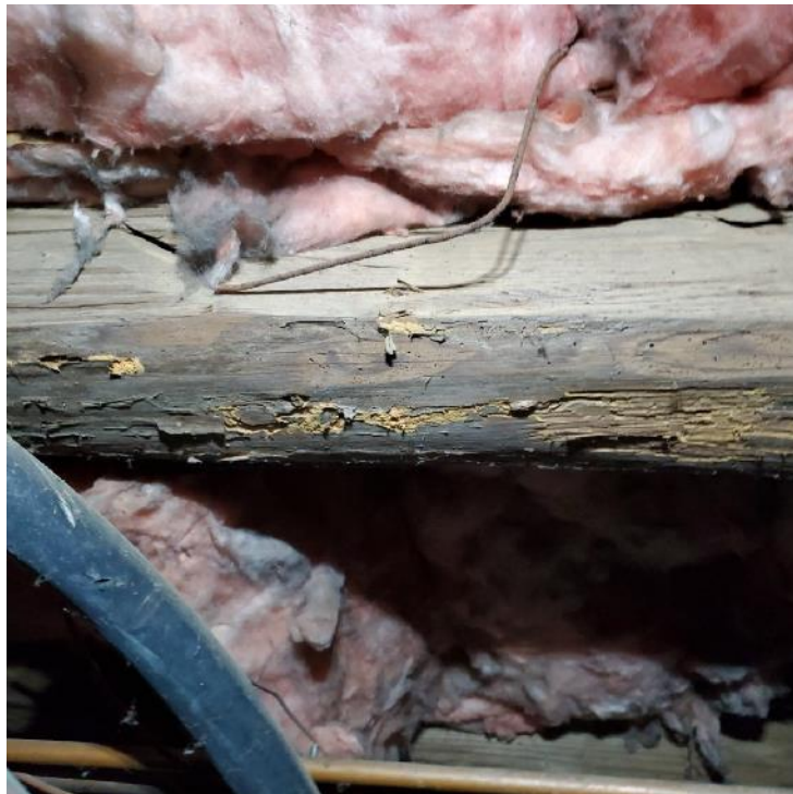
Photograph 72: View of potential insect related damage (oval).
