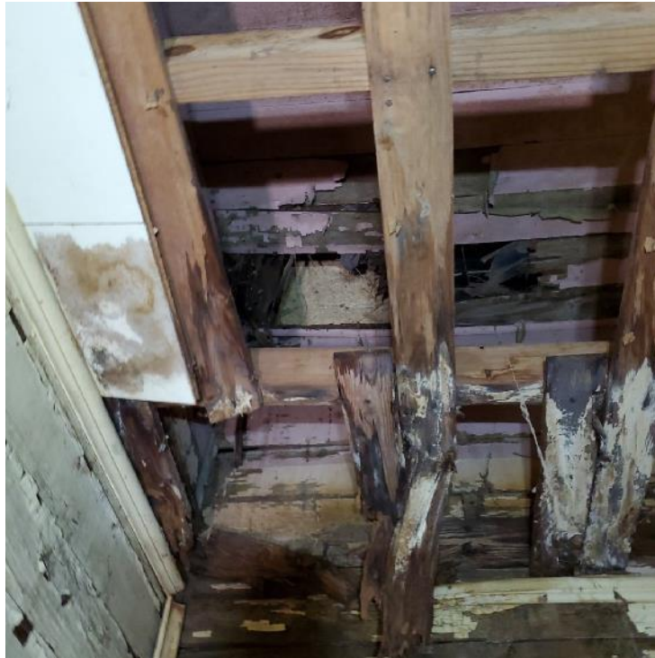
Photograph 51: View of water-related staining and damage in bedroom at north end of the rear portion of residence.
