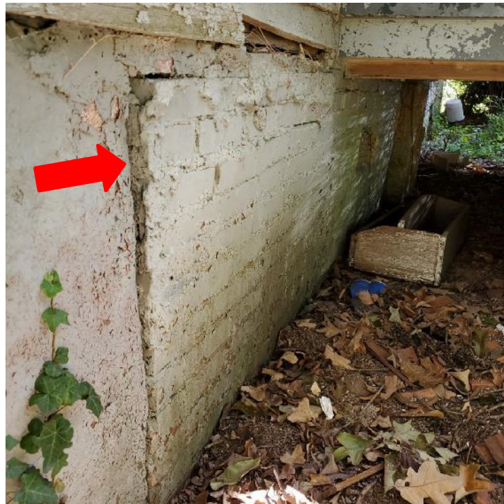
Photograph 18: View of vertical displacement of brick infill adjacent to the front porch (arrow). Note the paint along the side of the exposed brick.
