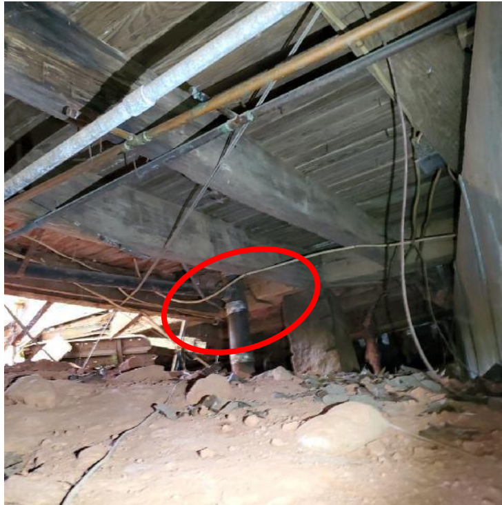
Photograph 61: View of porch framing below bathroom addition. Note the distress of the floor framing at the beam to girder connection (oval).
