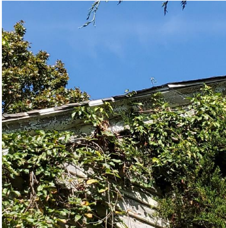
Photograph 13: View of vegetative growth along east elevation of original portion of residence.
