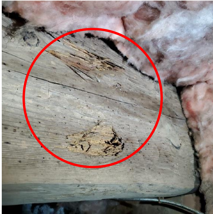
Photograph 73: View of potential insect related damage (oval).
