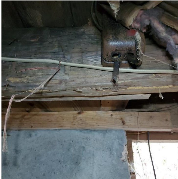
Photograph 71: View of potential insect related damage.
