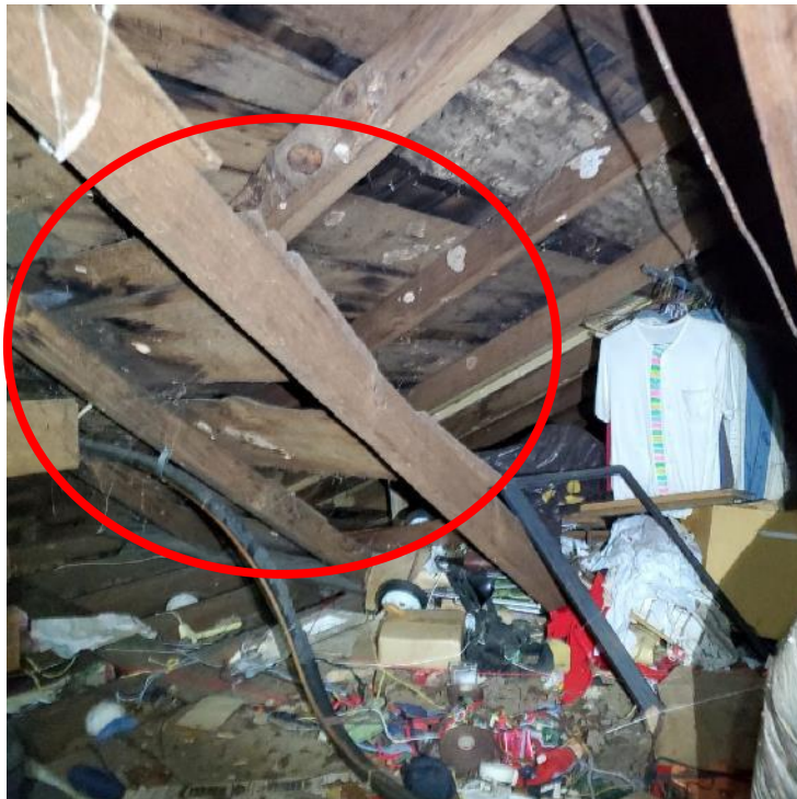
Photograph 38: View of water-related staining at original to rear portion roof transition (oval).
