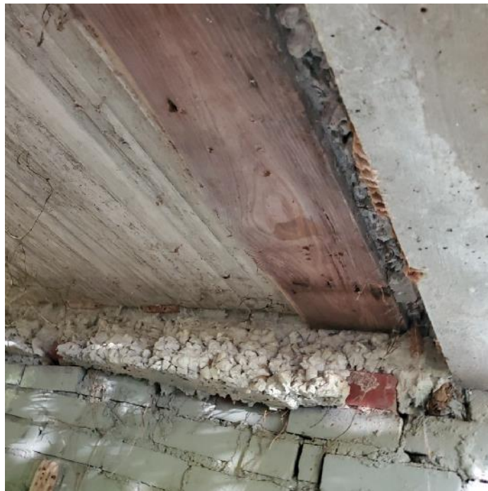
Photograph 16: View of front porch CIP concrete slab bearing on brick masonry infill.
