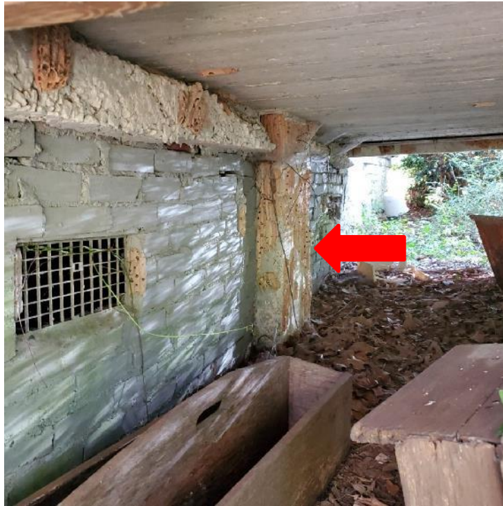
Photograph 19: View of mass stone pier located along south elevation porch slab bearing (arrow).
