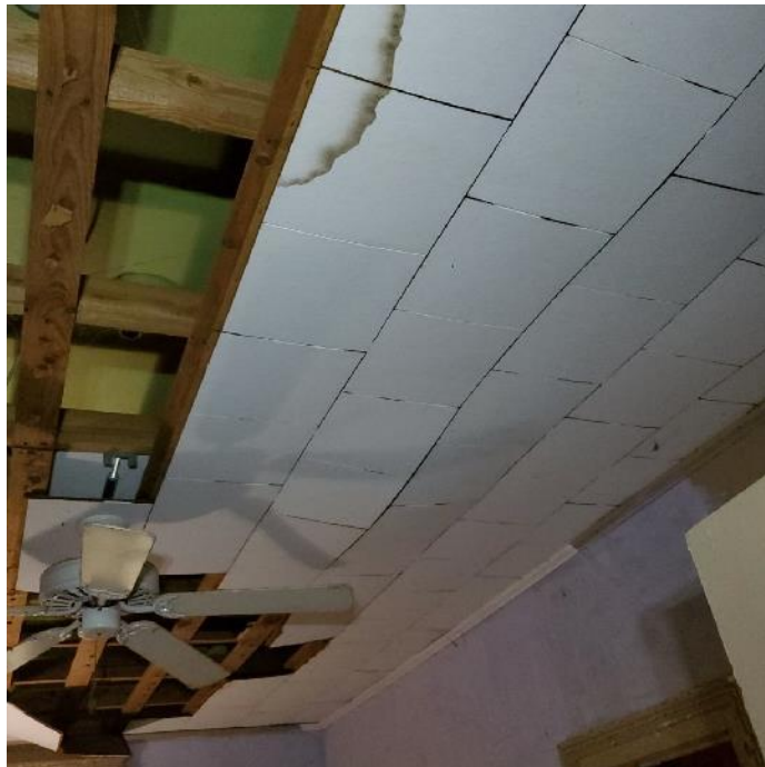
Photograph 44: Representative view of ceiling below original ceiling.
