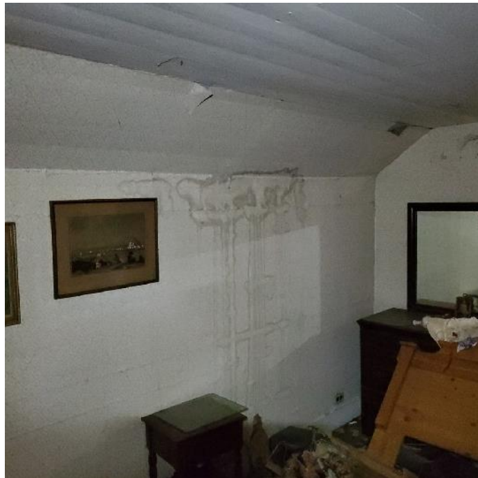
Photograph 36: View of water-related staining on wallpaper.
