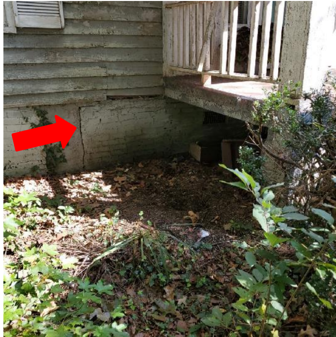
Photograph 17: View of vertical displacement of brick infill adjacent to the front porch (arrow).
