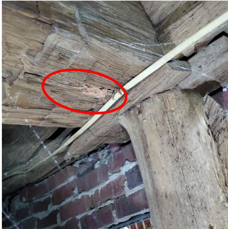
Photograph 69: View of insect related damage (oval).
