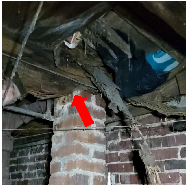
Photograph 63: View of brick pier at location of insect and water related damage to flooring. Note the crushed beam at the pier bearing (arrow).
