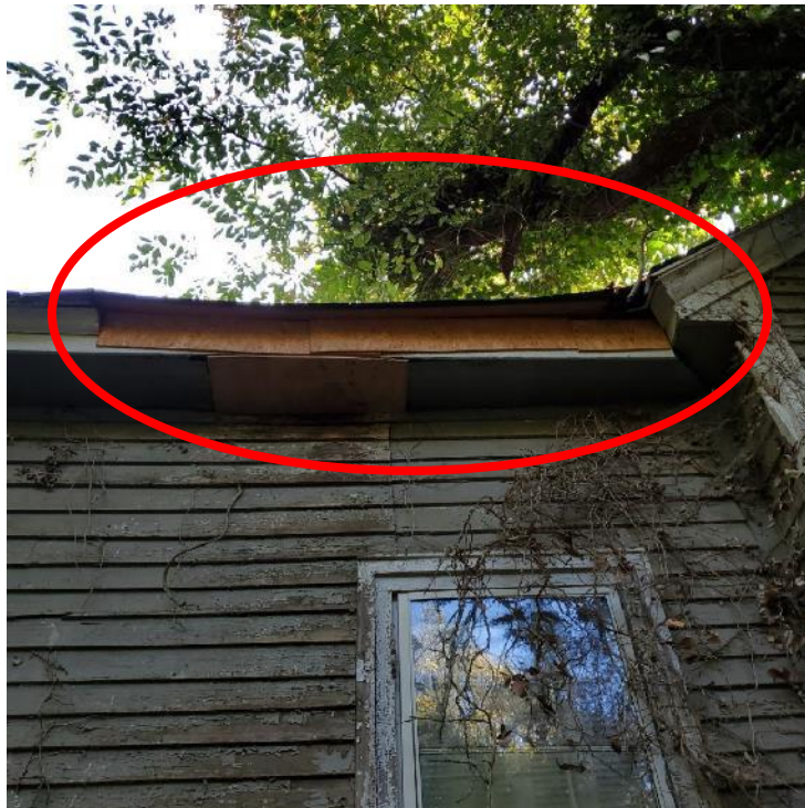
Photograph 24: View of plywood at fascia along the west elevation of the rear portion of the residence (oval).
