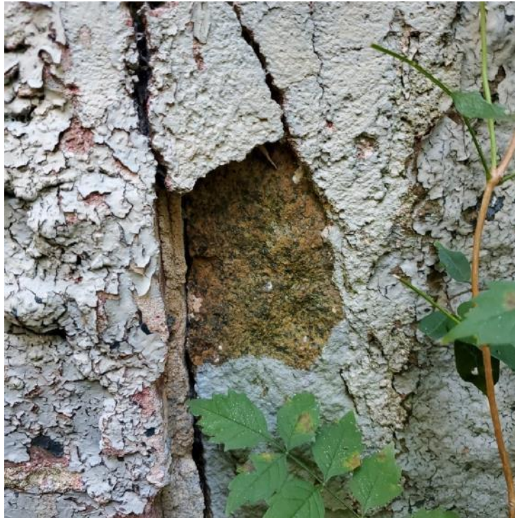
Photograph 21: Close-up view of delamination on the exterior face of the mass stone pier along the south elevation.
