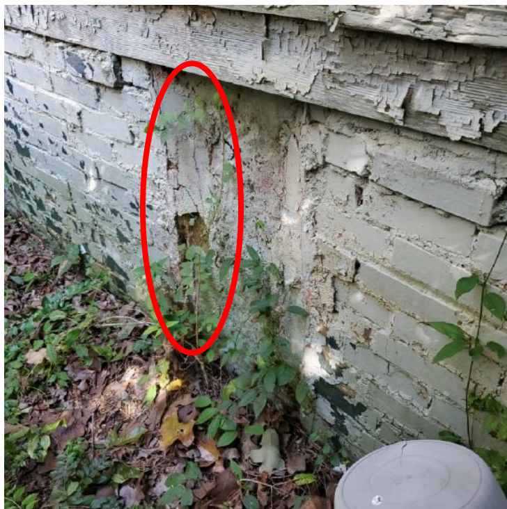
Photograph 20: View of delamination on the exterior face of the mass stone pier along the south elevation (oval).
