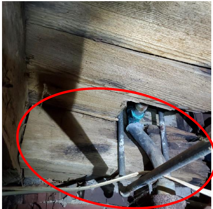
Photograph 66: View of insect and/or water related damage and downward displacement of the perimeter girder, see additional photo below (oval).
