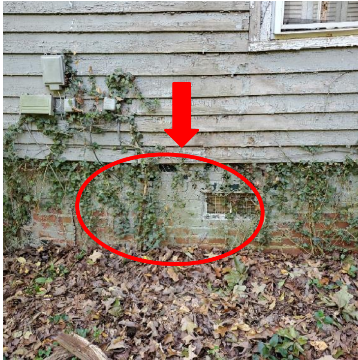
Photograph 25: View of sag in siding at the first-floor level along the west elevation of the rear portion of the residence (arrow). Note the step crack in the brick masonry infill (oval).
