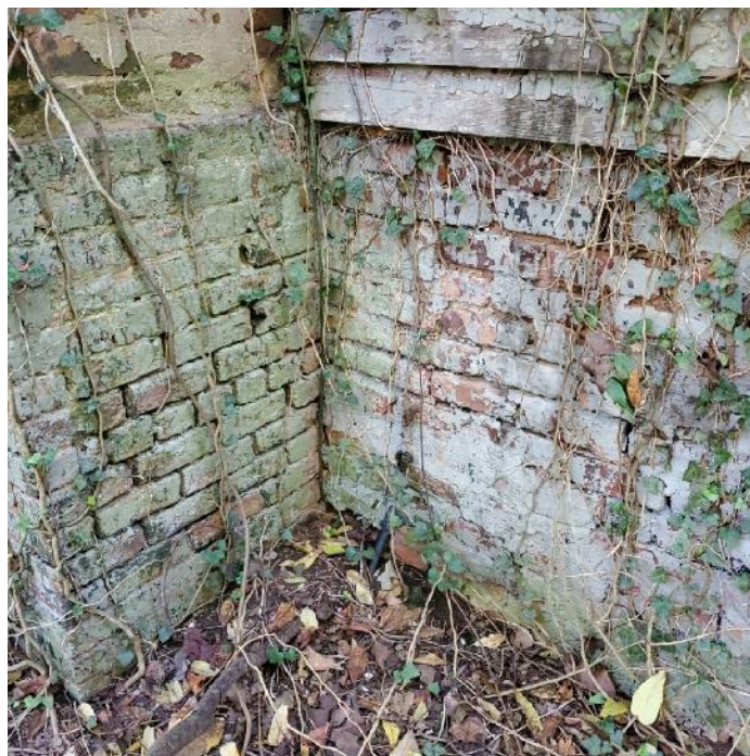
Photograph 26: View of recessed mortar joints in brick infill masonry and in the exterior chimney masonry.
