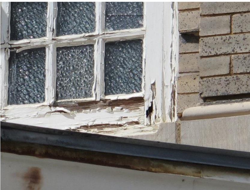
Figure 25: Severe window deterioration at clerestory.
