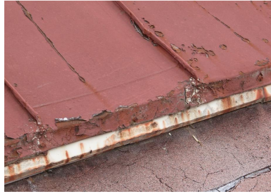
Figure 20: Corroded standing seam roof edge.
