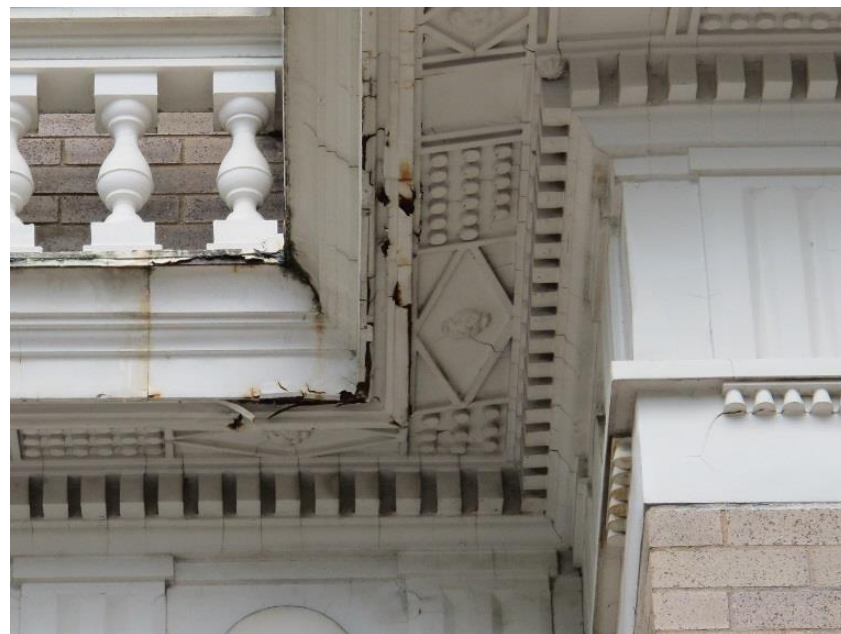
Figure 27: Severely corroded flashing components.
