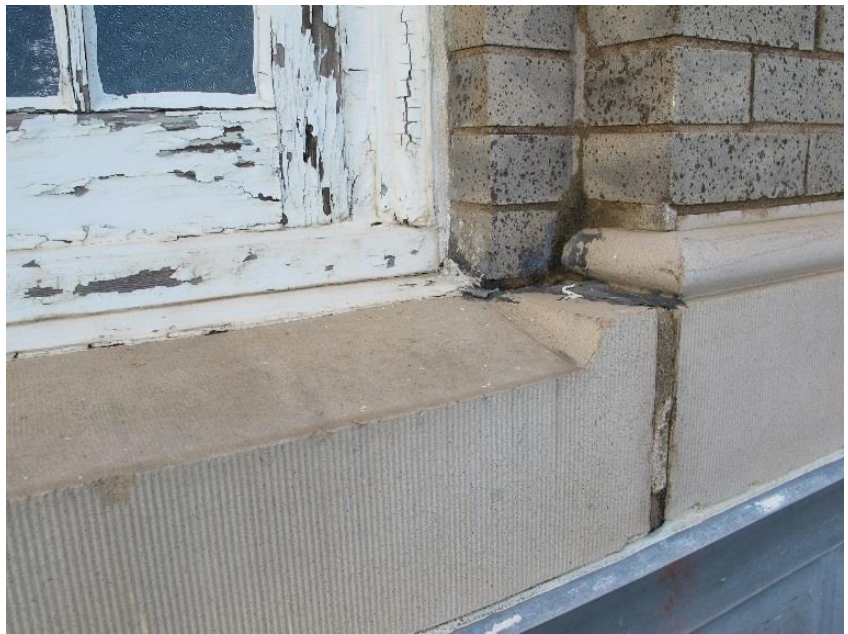
Figure 21: Severe window deterioration at clerestory.
