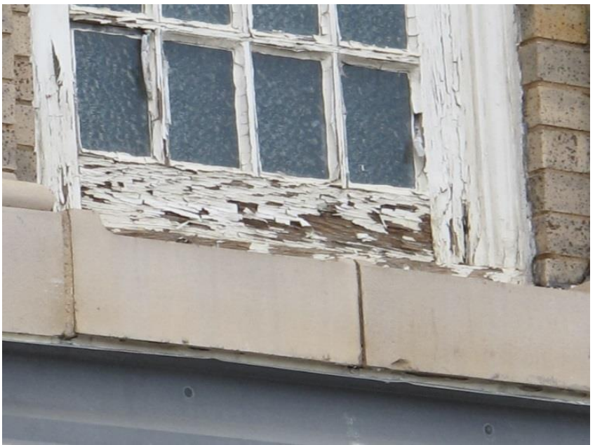
Figure 23: Severe window deterioration at clerestory.
