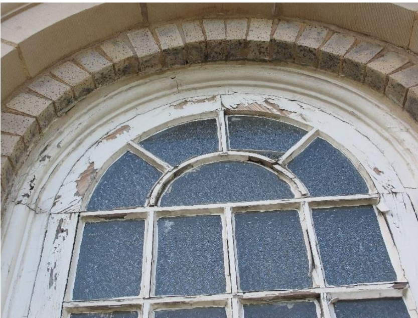
Figure 22: Severe window deterioration at clerestory.
