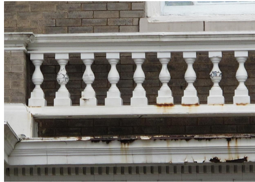
Figure 17: Balustrade over original First Baptist church entrance in need of repair / replacement.
