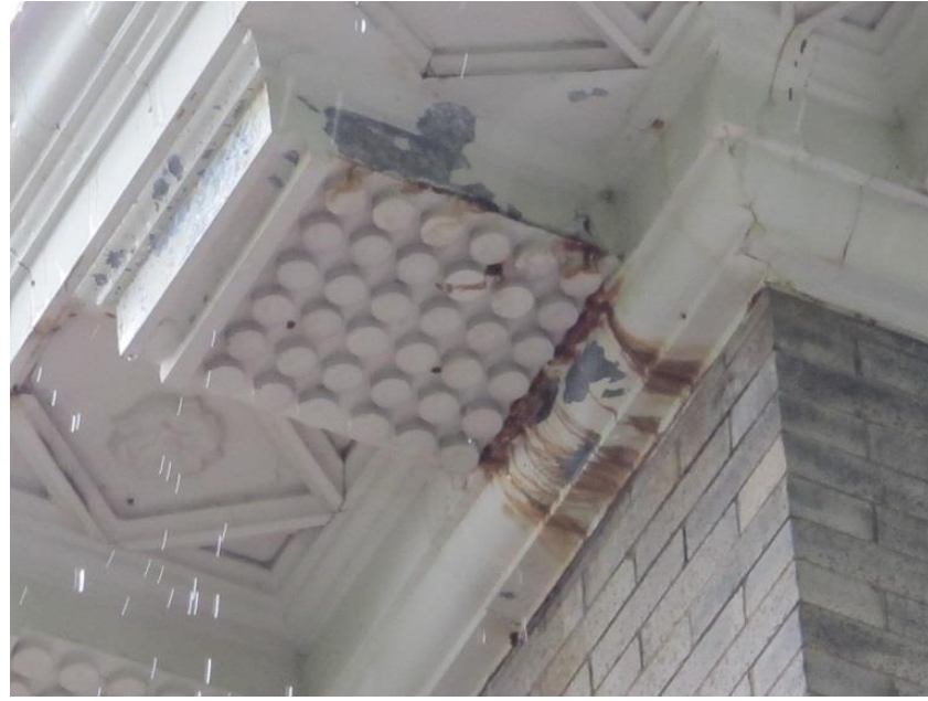
Figure 29: Active gutter leak at northeast soffit.
