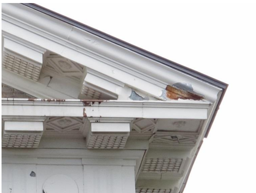
Figure 28: Severely corroded flashing components.
