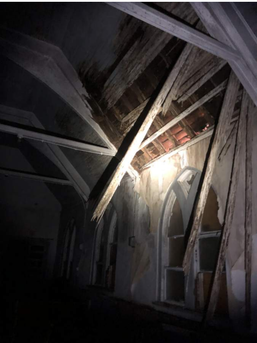
ROOF FAILURE
