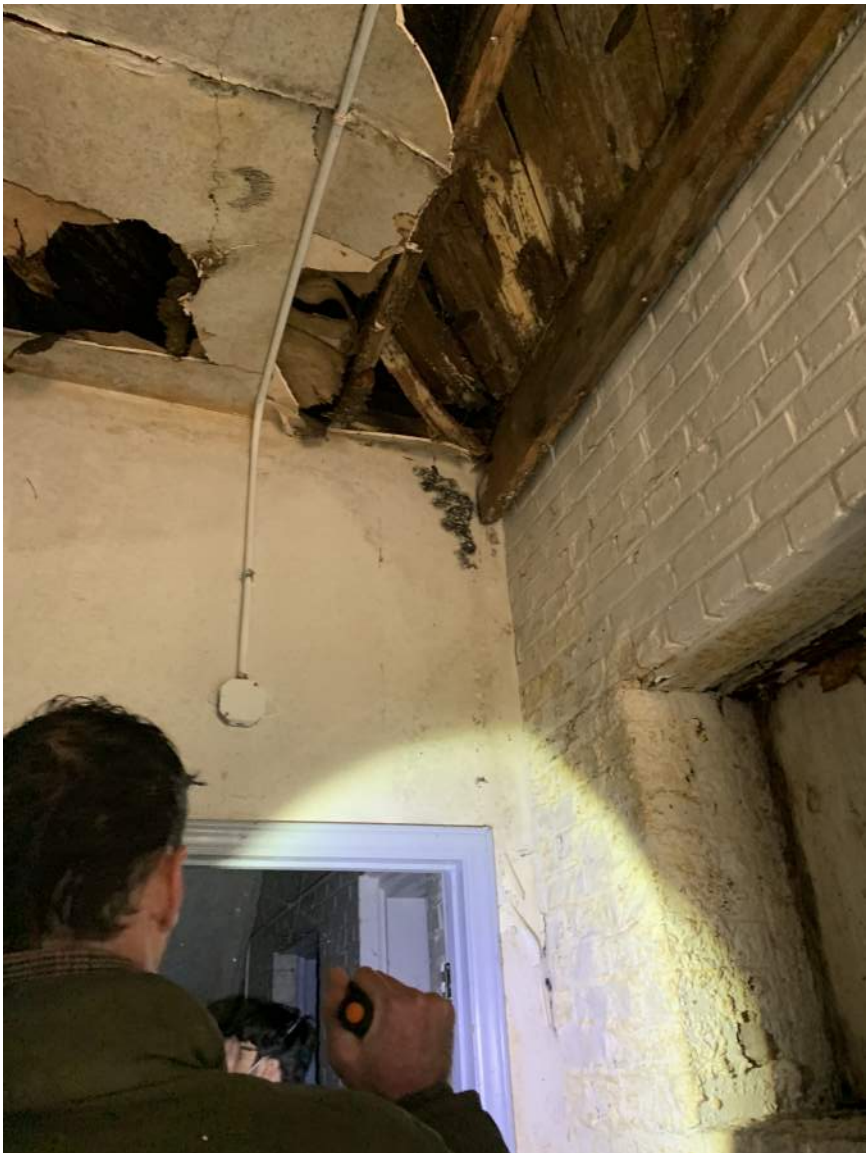
FLOORING FAILURE
