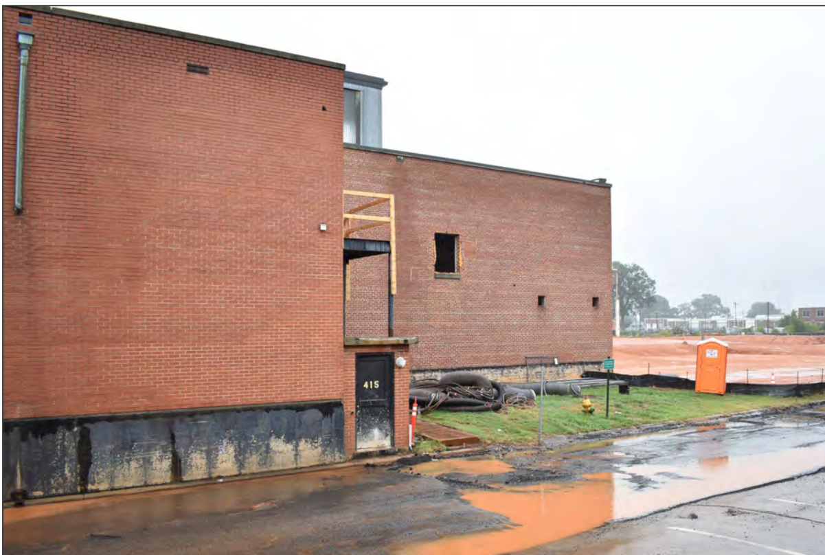
27. 701 Keswick, west elevation, view south
