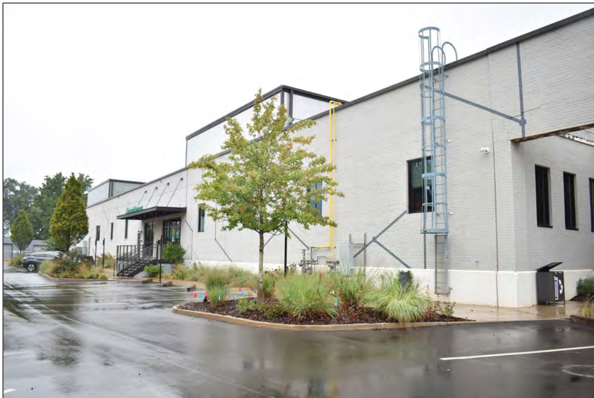
38. 1701 N. Graham, east elevation, view southwest
