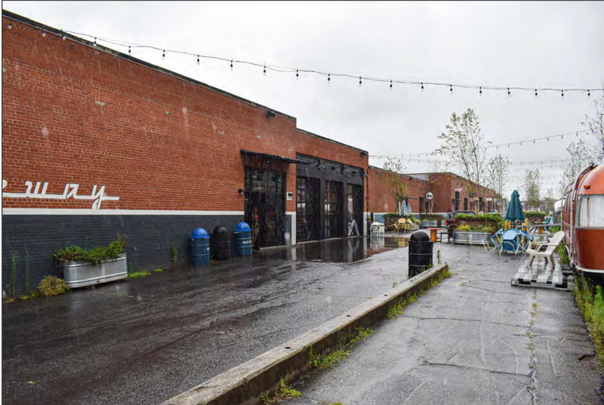
52. 1824 Statesville, south elevation, view northeast
