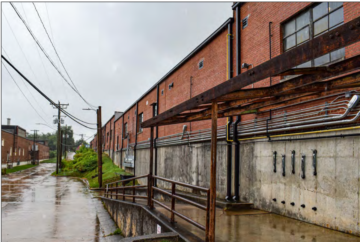
51. 1824 Statesville, north elevation, view southeast
