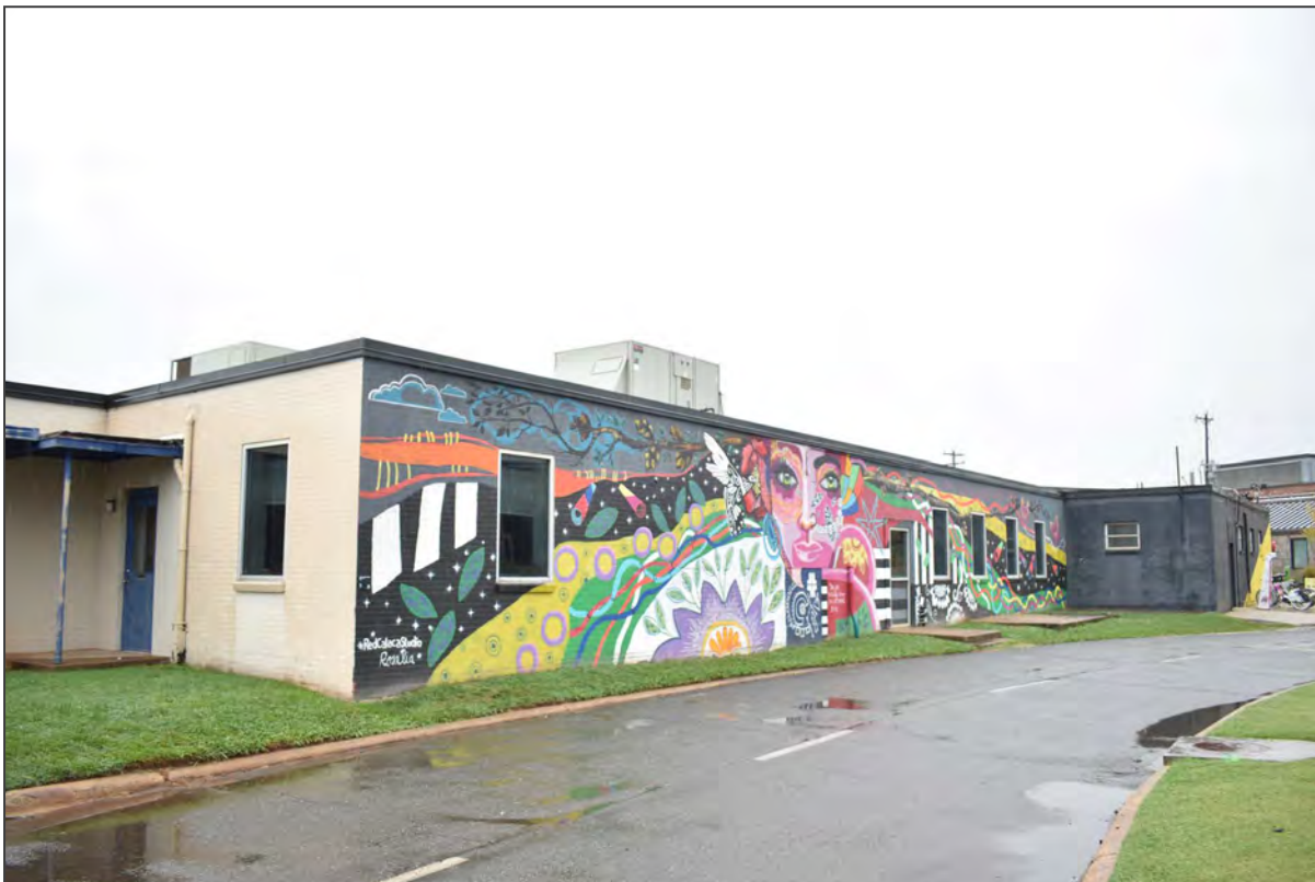
47. 330 Camp, west and south elevations, view northeast
