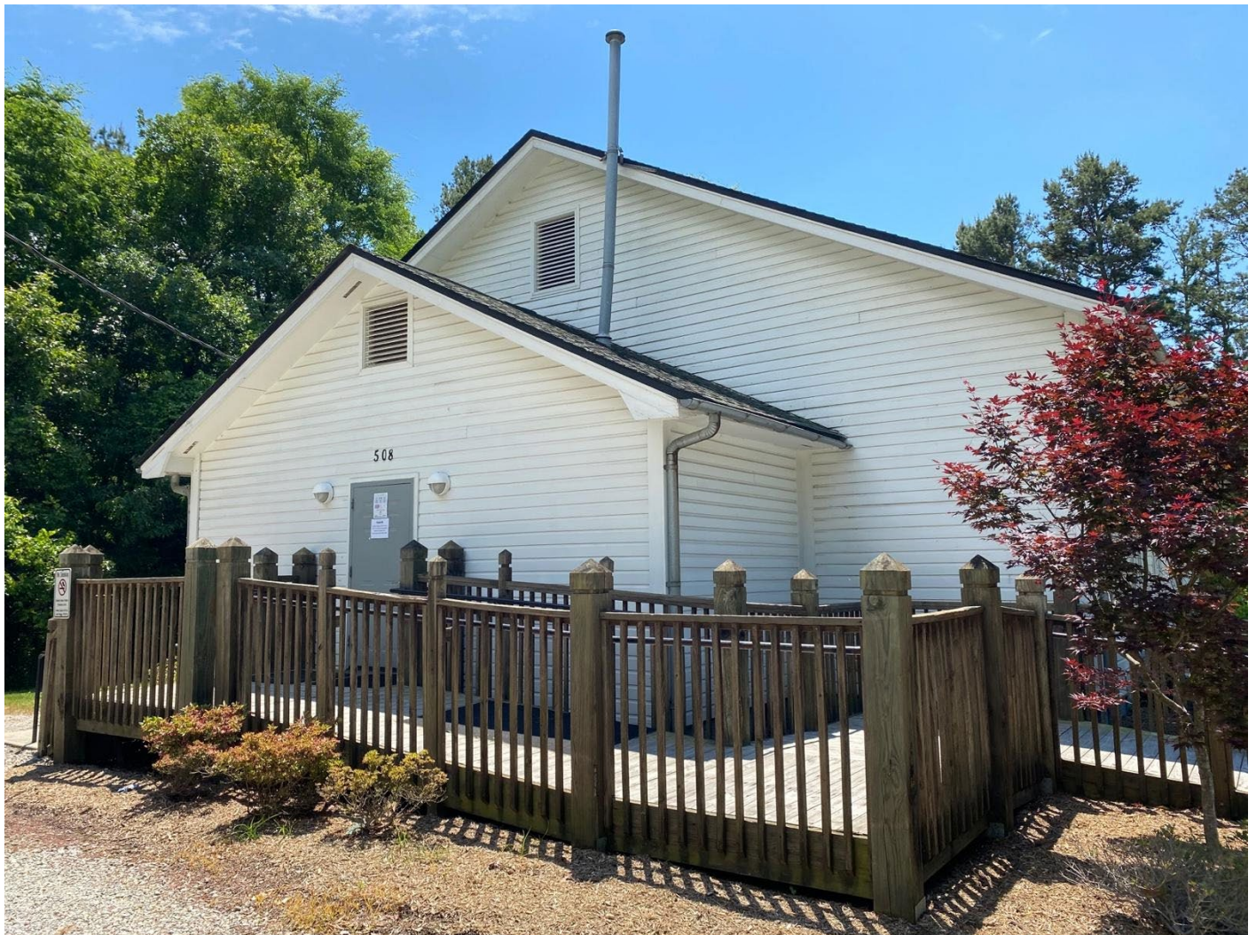
Fig. 2: Front (North) Elevation
