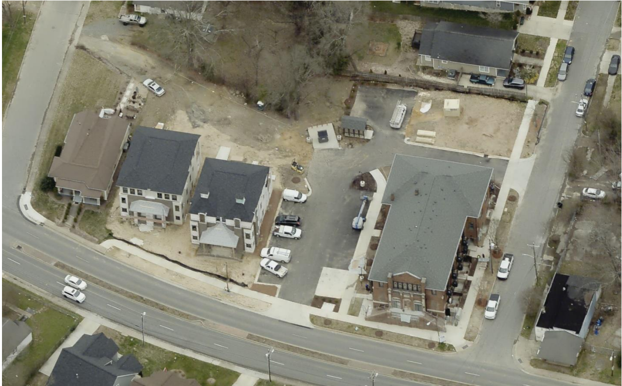
Figure 7 Aerial view of the former Parkwood Avenue A. R. P. Church property.
