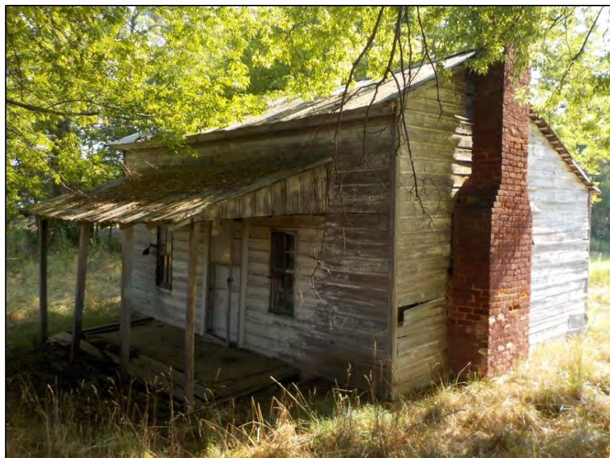
Figure 8. Resource No. MK2293, facing northeast.
