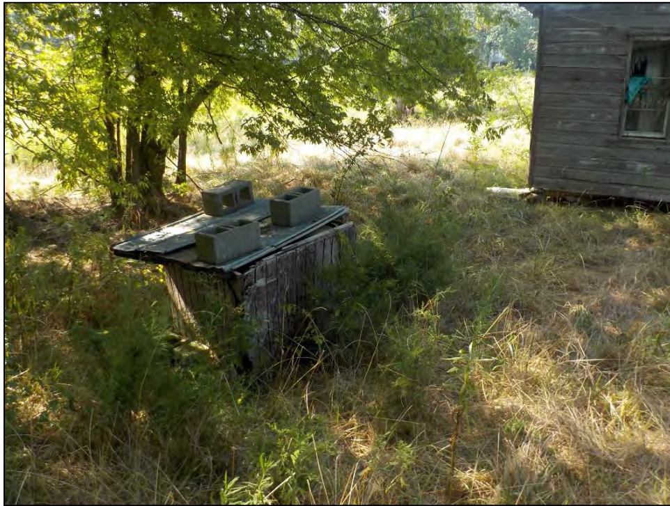
Figure 11. Wellhouse, facing southeast.
