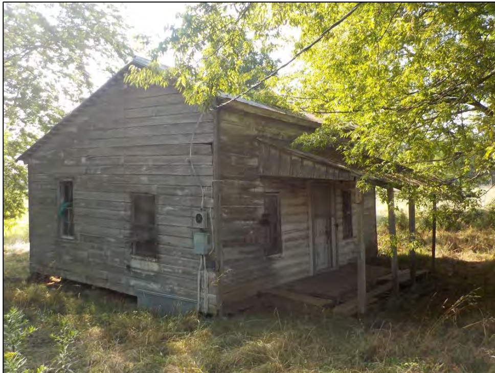
Figure 10. Resource No. MK2293, facing southeast.
