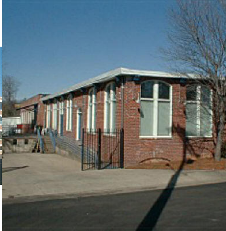
W.C. Newell Company warehouse
