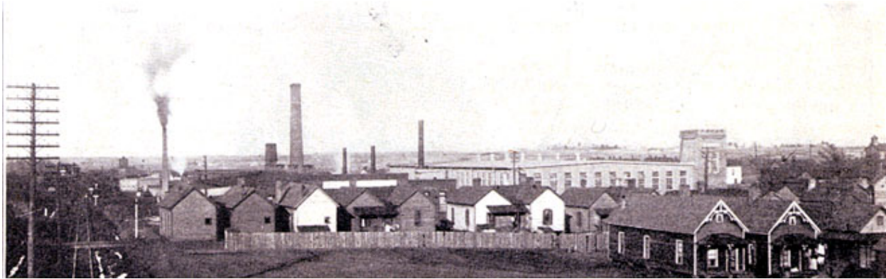
Early 20th-century photograph of the Alpha Mill village west of the mill, now demolished
